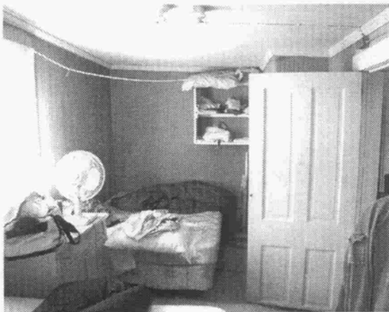
Figure 34 View to west in Room 101. (NPS-SERO-CR, 2002)
