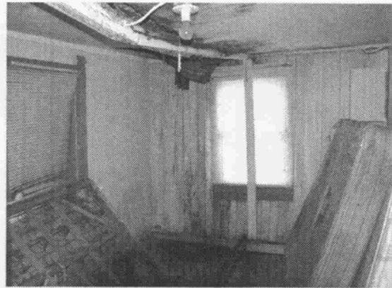
Figure 40 View to west in Room 104. (NPS-SERO-CR, 2002)
