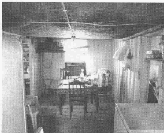
Figure 37 View to northeast in Room 102. (NPS-SERO-CR, 2002)
