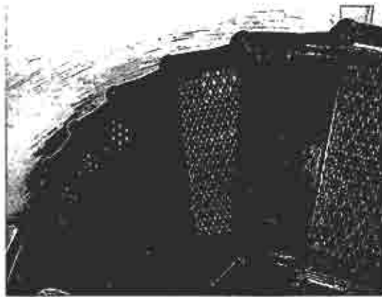
Figure 14 Existing repairs to stair treads.
