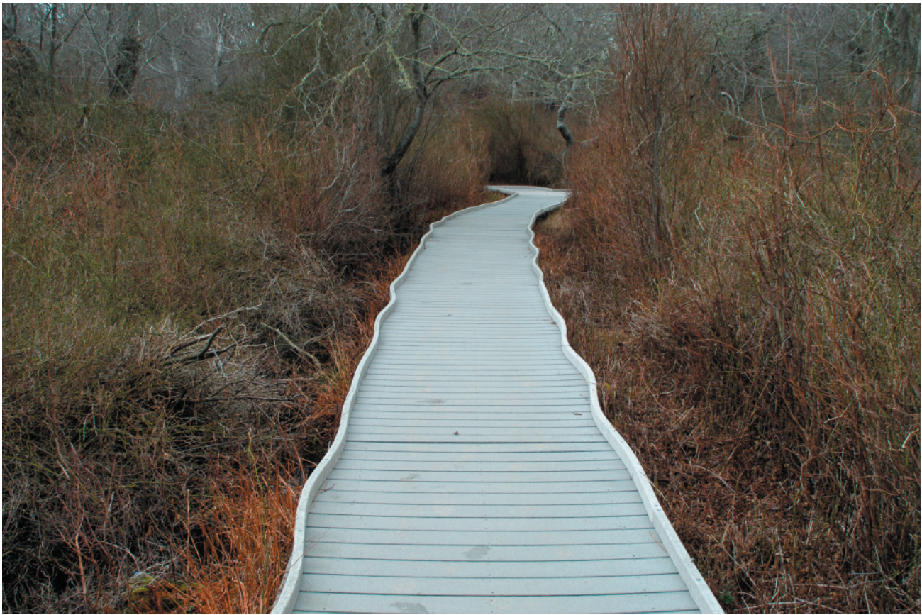
Figure 68. Photograph of the boardwalk on the Red Maple Swamp Trail. The thin pieces of recycled wood used for edging have expanded, causing the boardwalk to have a warped, wavy appearance (OCLP, January 2007).
