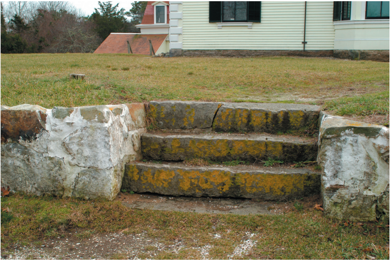
Figure 25. Granite steps on the north side of the Penniman house along Fort Hill Road. The addition of a simple, unobtrusive hand rail would aid visitors with mobility or sight impairments (OCLP, January 2007).
