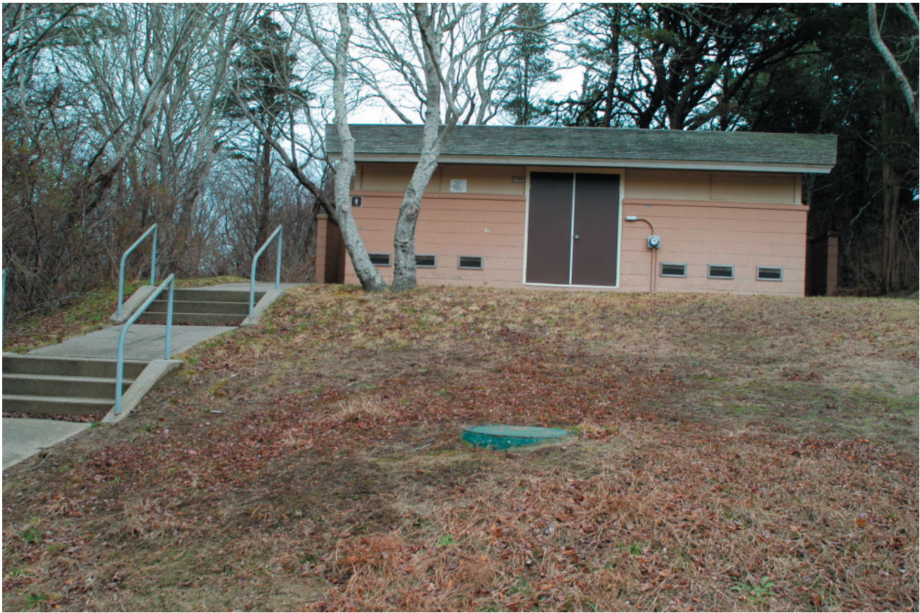
Figure 76. Photograph showing the comfort station at Skiff Hill, near the Hemenway Road entrance (OCLP, January 2007).
