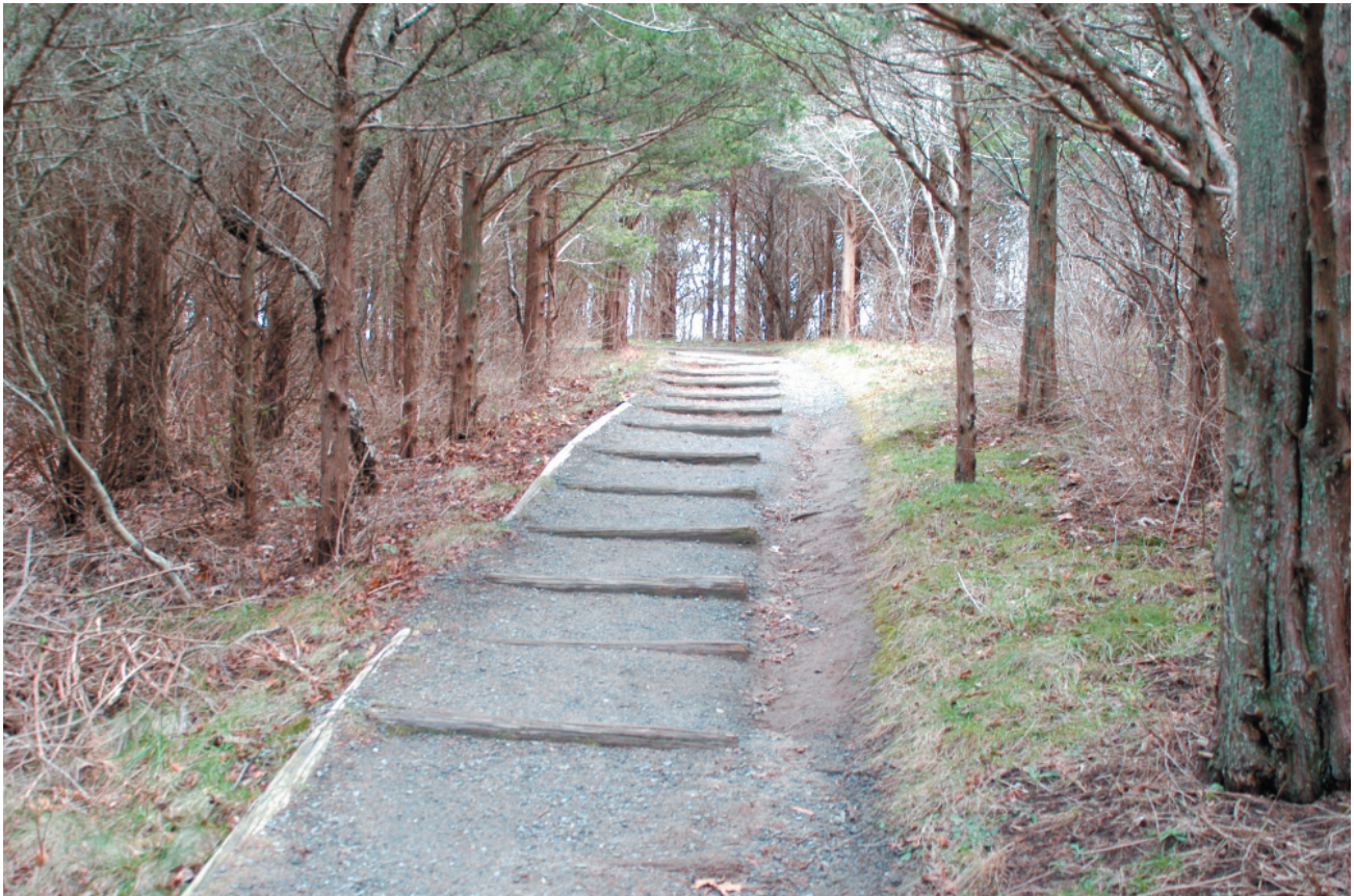
Figure 73. Photograph of the erosion along the gravel trails in the Red Maple Swamp (OCLP, January 2007).
