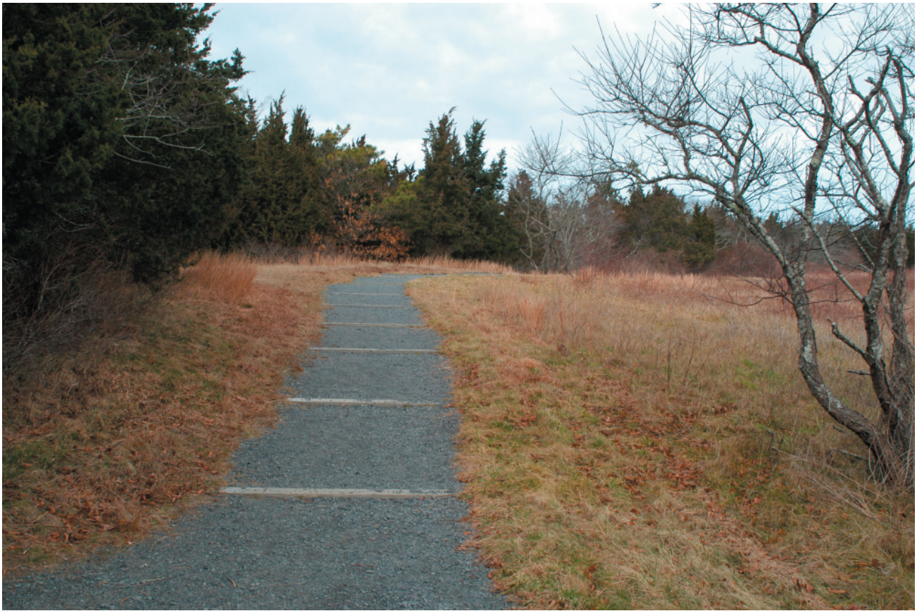
Figure 23. Photograph showing the existing bluestone gravel surface of the Fort Hill Trail. The surface material for these paths will be changed to a native colored gravel to harmonize with the natural setting (OCLP, January 2007).
