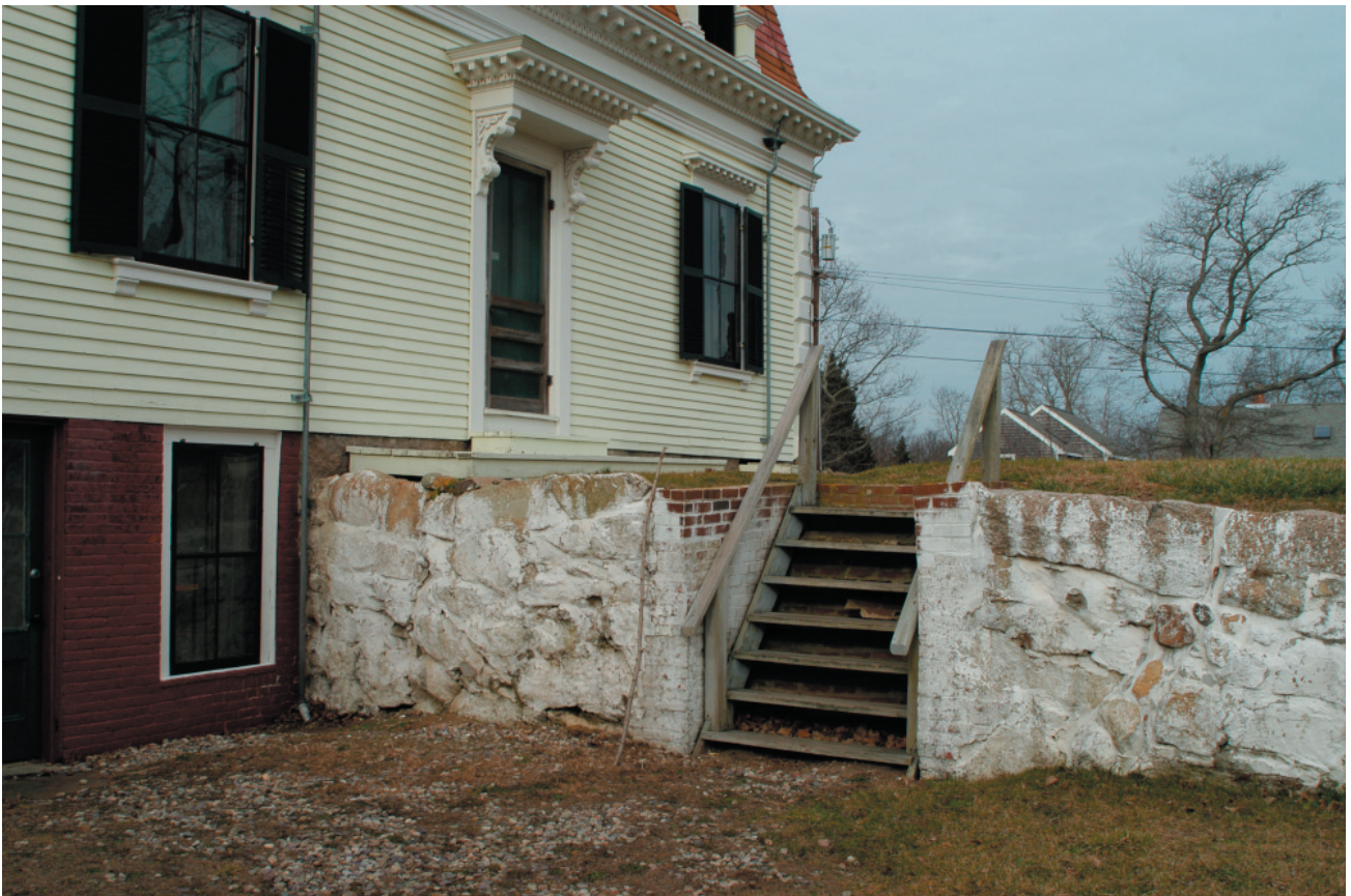
Figure 26. Steep wooden steps on the east side of the Penniman house, which connect the driveway and barn yard. The steps could be rebuilt with a gentler pitch by extending them out from the wall towards the driveway (OCLP, January 2007).
