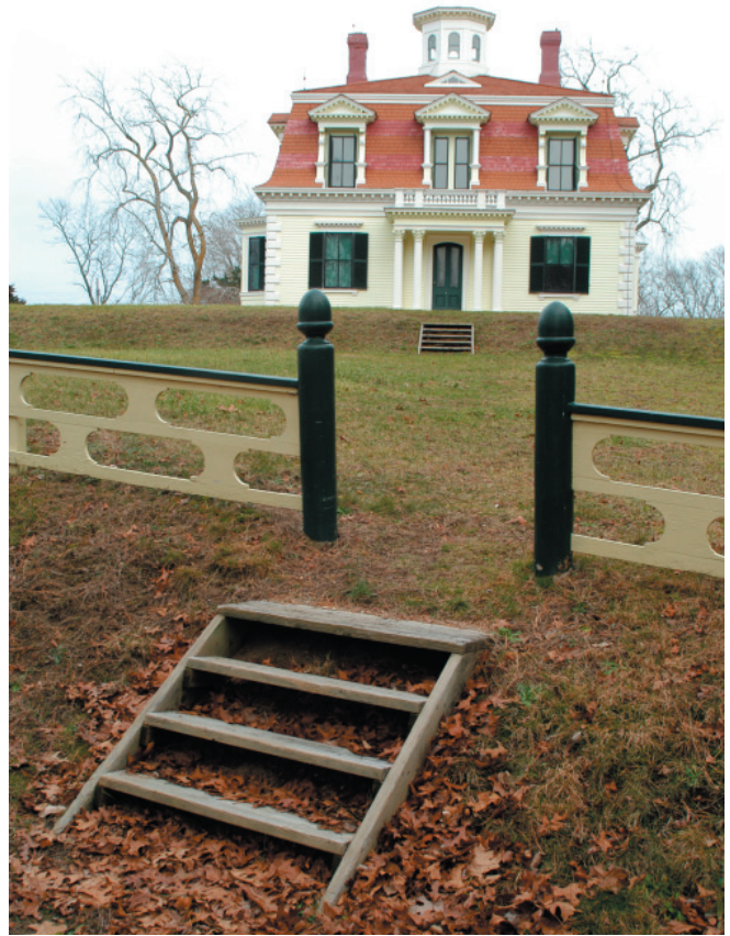
Figure 3. View looking east at west facade of Penniman house, perched on terraced lawn as seen from the south side of Fort Hill Road. A decorative fence surrounds the lawn (OCLP, January 2007).
