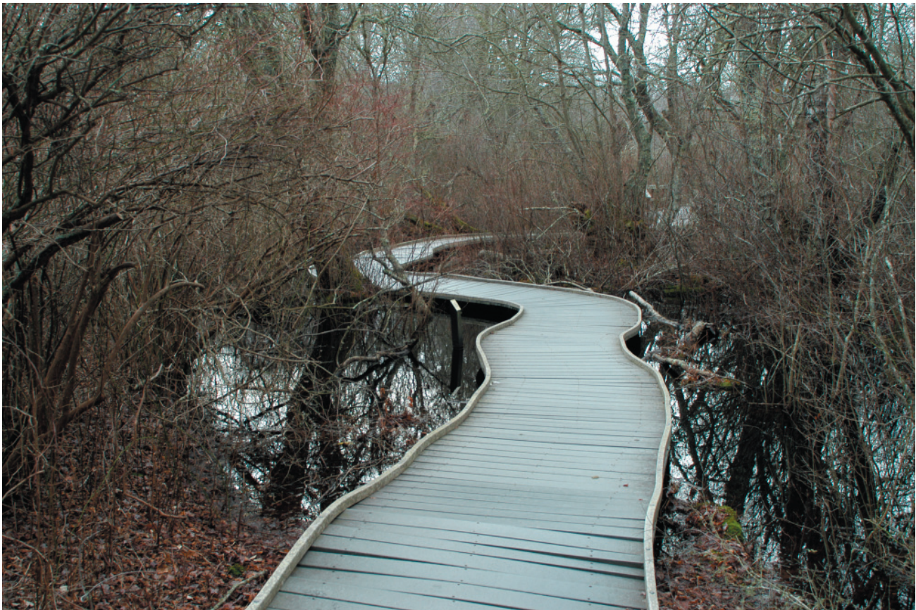
Figure 69. Photograph of the boardwalk on the Red Maple Swamp Trail, over standing water. In the foreground the old posts under the new boardwalk have rotted, causing the decking to collapse (OCLP, January 2007).
