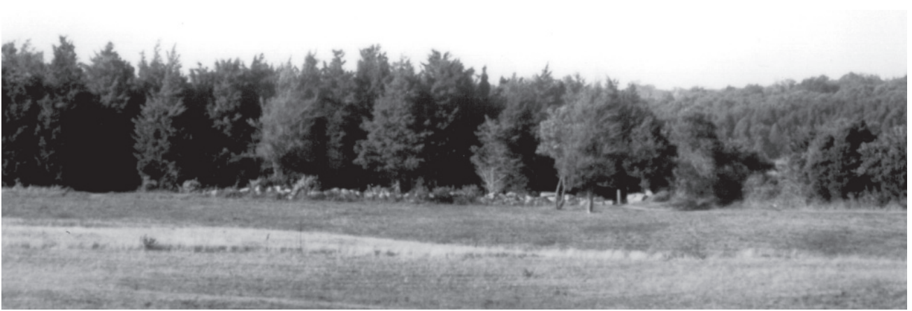
Figure 61. Photograph looking north at a stone wall on the northern edge of the open fields, also referred to as wall #1, 1993. The wall is still clearly visible as a hard edge to the field (Fort Hill CLR, 1995, 69).
