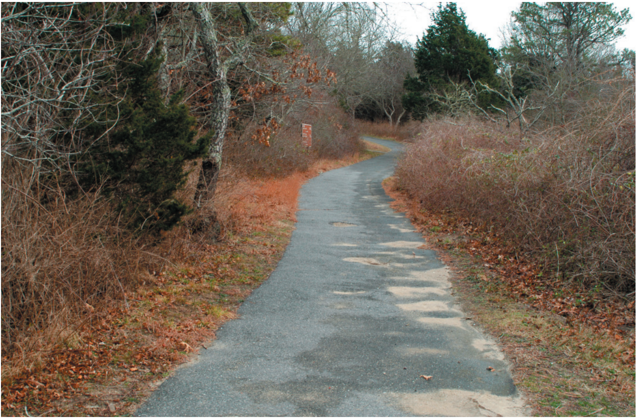
Figure 70. Photograph of the asphalt path at the Hemenway Road entrance. This surface could be replaced with gravel, narrowed, or chip-sealed and top-coated with bound gravel (OCLP, January 2007). The photograph below shows an example of a chip-sealed surface.
