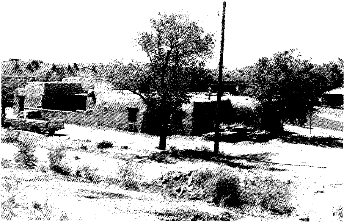
From the rear (south) the building's original massing remains. The stucco finish is too highly textured for this building.
