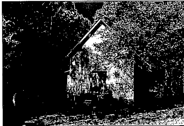
Figure 66. Erbie Church, 1977. Despite depopulation of Erbie, a congregation continued to hold regular services here until 2000. Fred Mang, Jr. collection, Buffalo National River.
