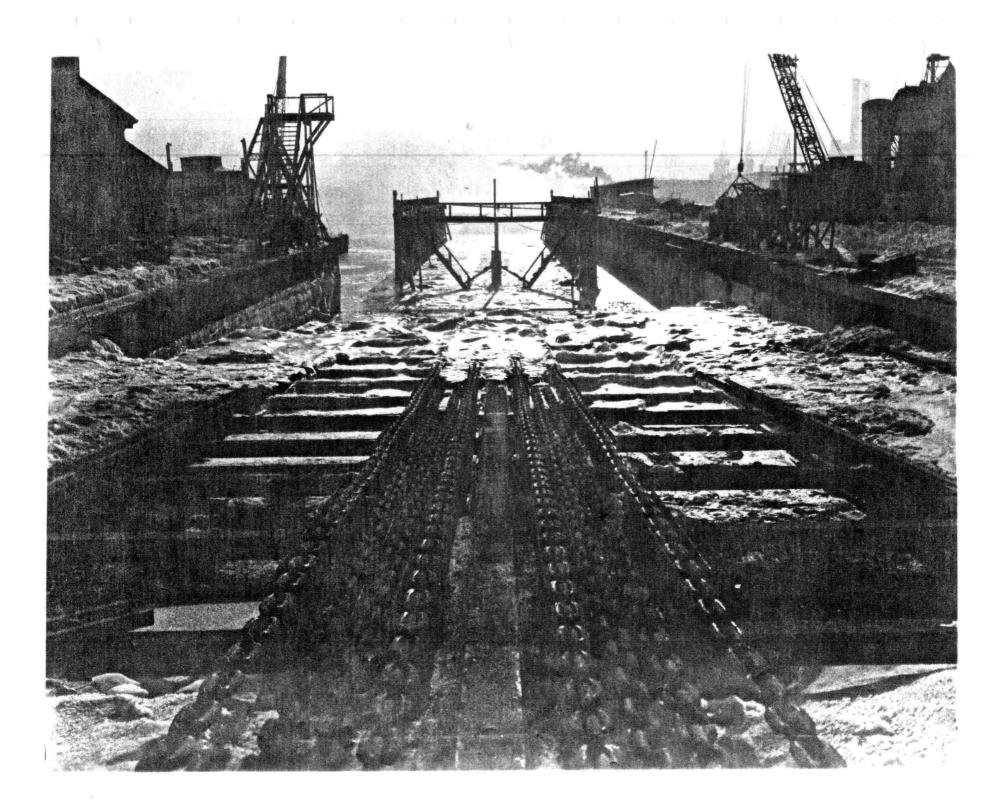
Entering the Cradle of the Marine Railway, Submarine USS Torsk (SS-423).
