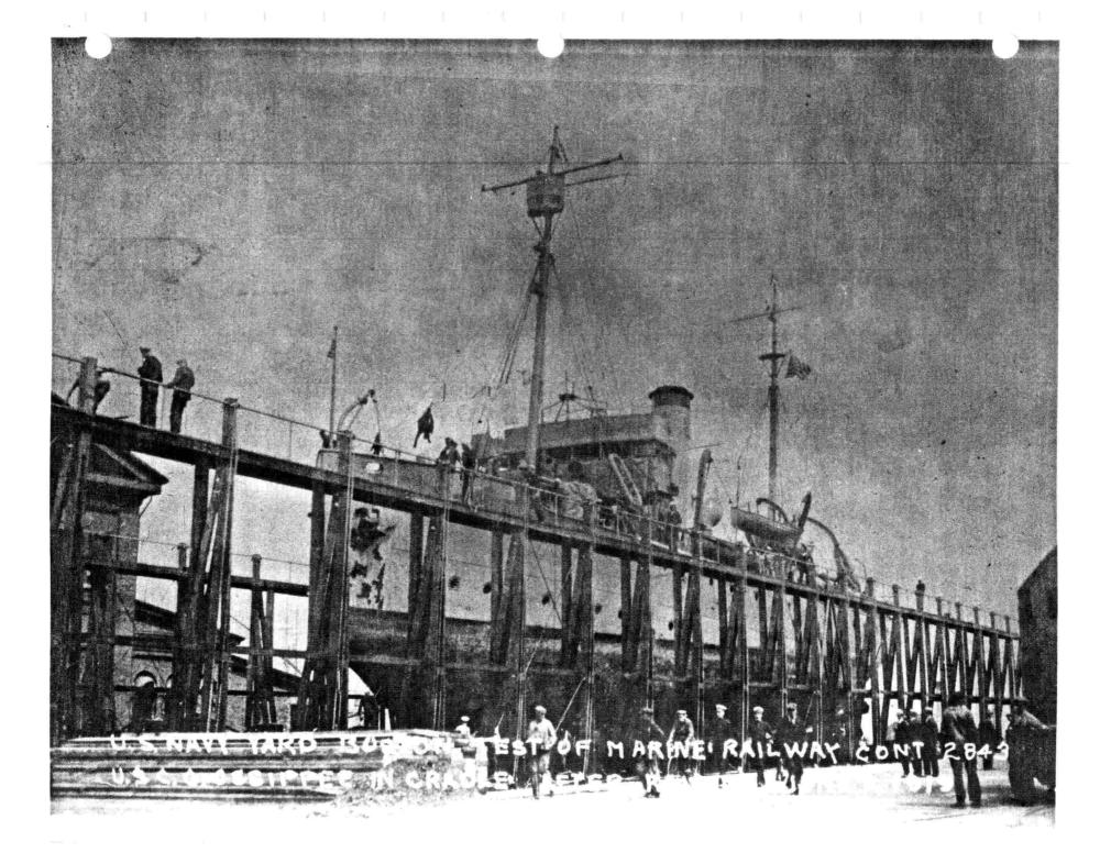
"Navy Yard Boston, Test of Marine Railway, Cont. 2843, Cradle Out With U.S.S. Grebe & U.S.S. Acushnet, June 10, 1919." From north.
