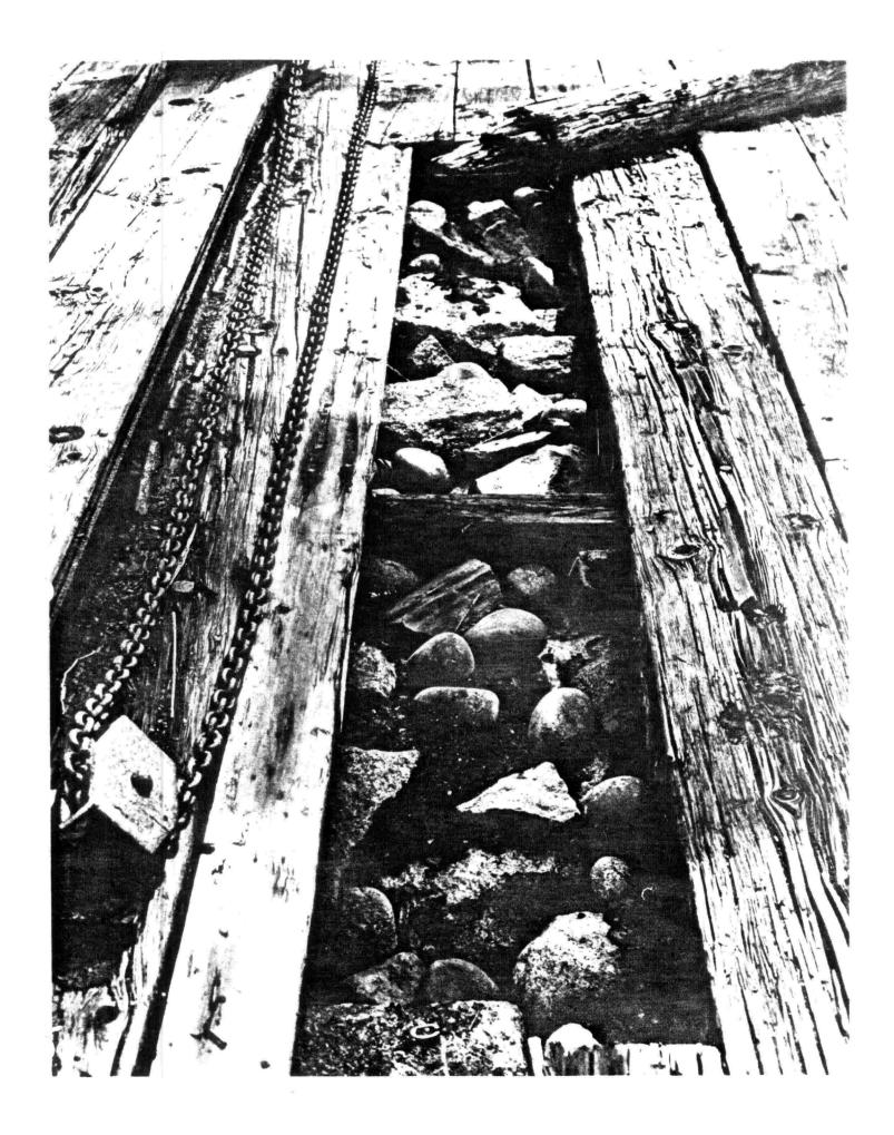
"Marine Railway #11. Underdeck Inspection. Cradle Joint Inspection Between Bearers #10 & #11. East Side," 1951.
