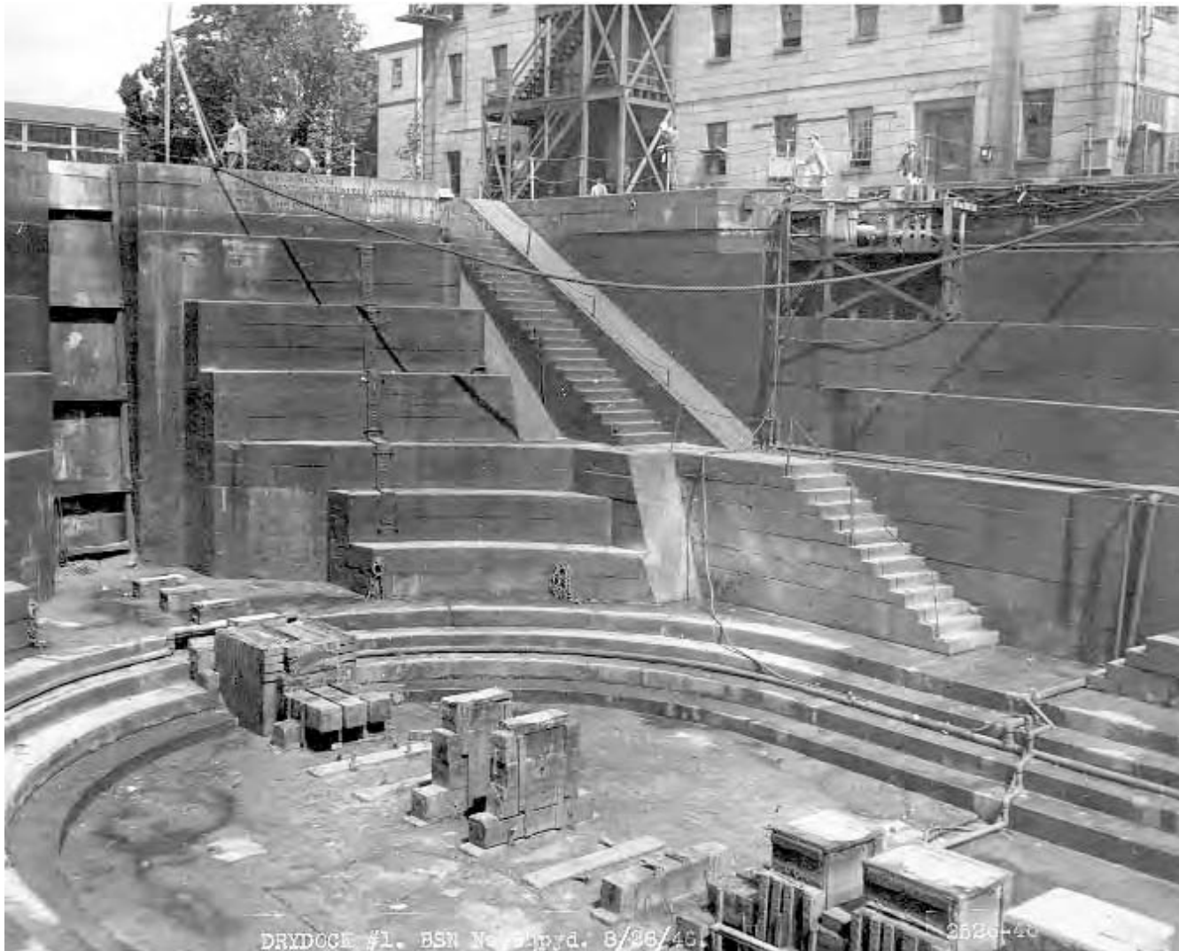
Fig. B-13 Photo BOSTS – 8795. View of the head of dock, looking northeast, on August 26, 1946. Note the altered center slide, which entailed the removal of the slide’s massive granite blocks, carried out about five years earlier. Note that the granite backing, which was behind the center slide, is now visible. Most of this granite backing was later covered with concrete. Note the wooden platform, above the granite stairway. This platform was replaced with a steel platform in the mid-1950s. Also note that the curved granite steps at the floor level are still in place.
