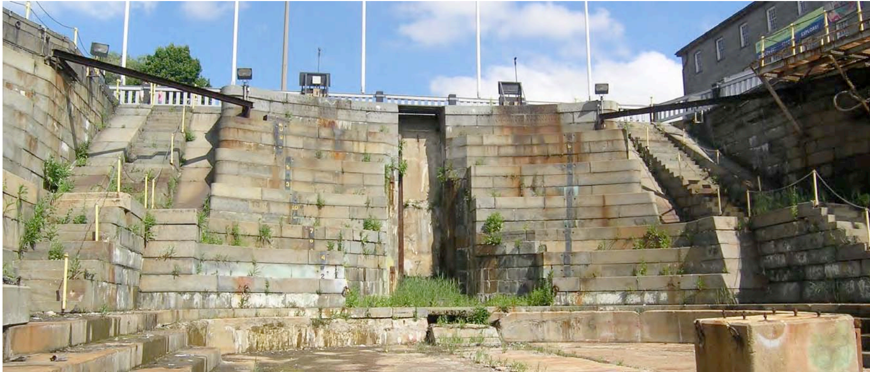
Fig. 20 View of head of dock showing alterations to center slide and lower stairs to the dry dock floor.
