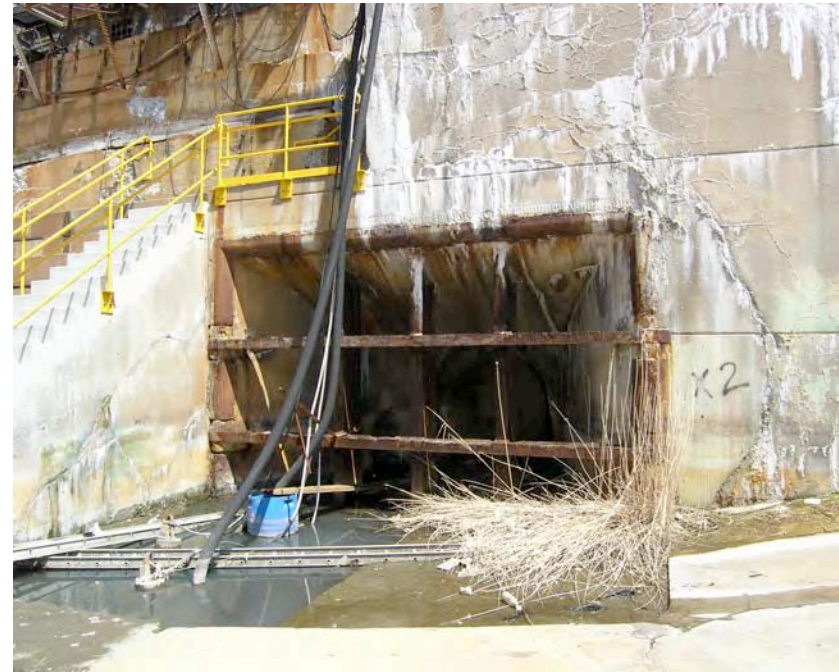
Fig. 27 Detail of tunnel intake and steel frame across its entrance.
