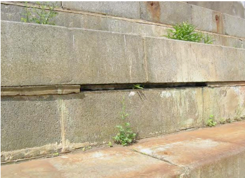
Fig. 11 Detail of vegetation, missing grout, and deteriorated mortar in joints of the lower altars on the west side of the chamber. This condition is prevalent throughout the dry dock.
