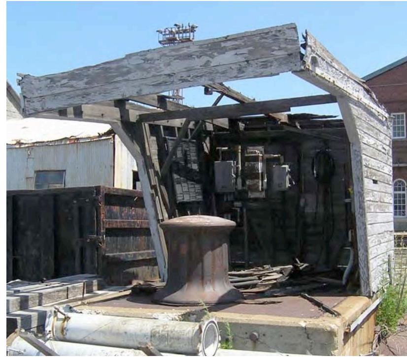
Fig. 30 Capstan No. 3 on the dock's east side near the caisson gate, looking east. The dilapidated wood-frame structure, which contains electrical panels, partially encloses this capstan.
