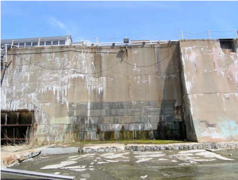
Fig. 26 View of east wall of the 1947-1948 seaward extension, showing deteriorated concrete work. The lower courses of granite that were part of the original turning basin were retained.
