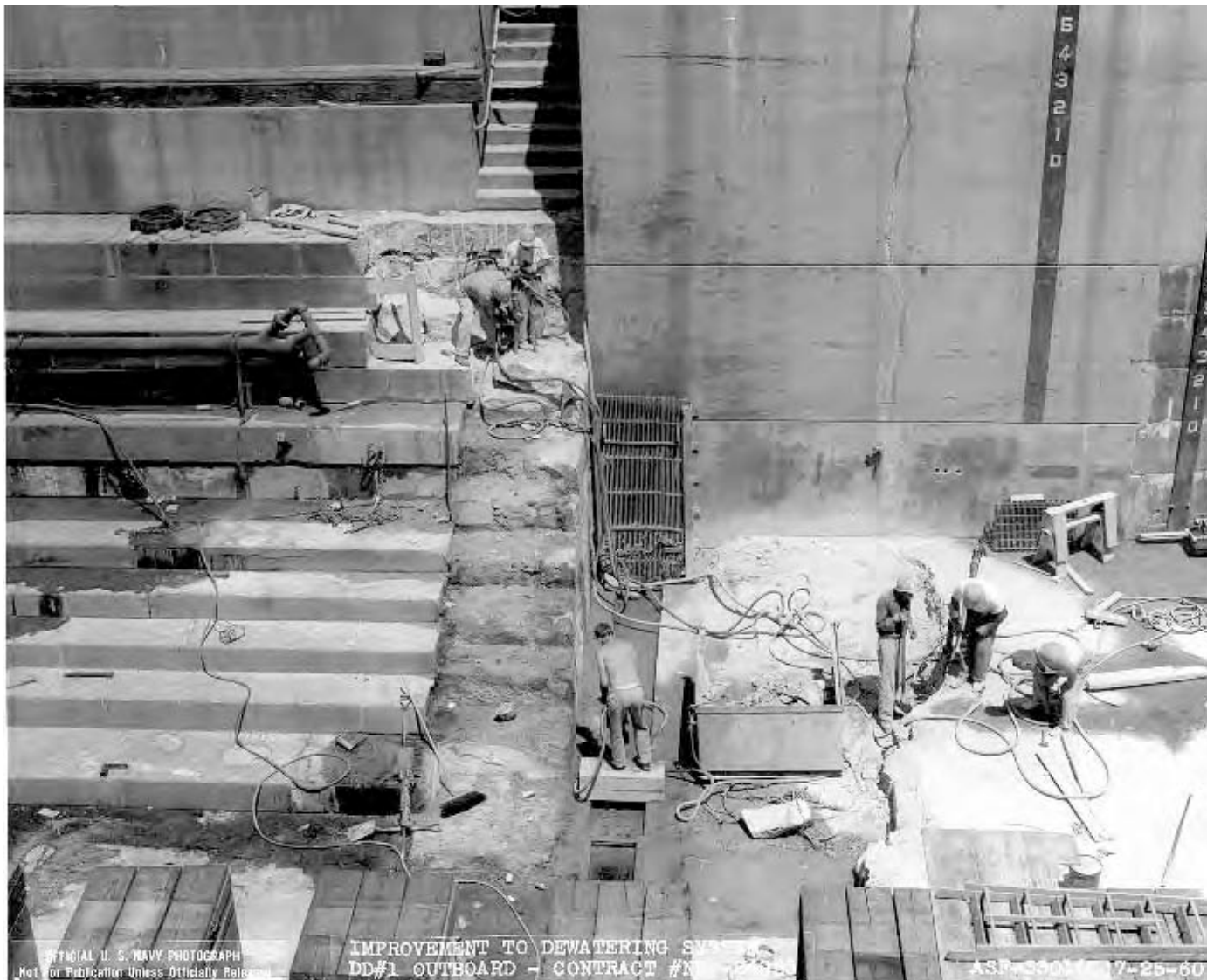
Fig. B-28 Photo BOSTS – 8800. July 25, 1960 view showing workers demolishing the original granite Stair I at the west wall near the seaward extension. This was done in advance of cutting a section through the west wall for the tunnel intake.
