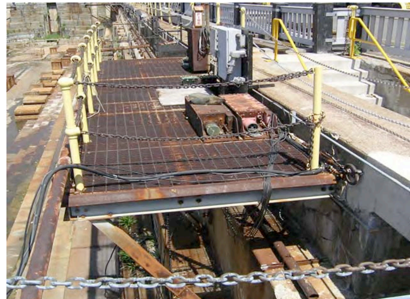
Fig. 33 Work platform, east wall, near seaward end. Note the abandoned utility lines and boxes on the platform.
