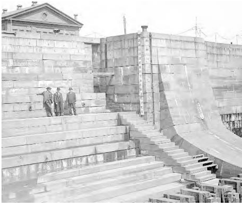
(B7) View of one of the draft gauges of Dry Dock 1 in the late-19th century. This gauge was adjacent to the original seaward stairs (Stair 1) on the east side of the dock.
