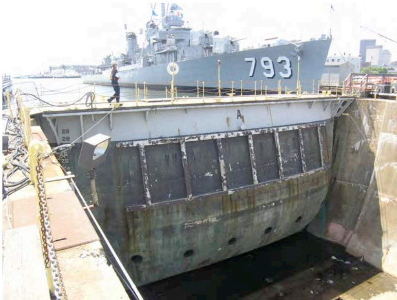
Fig. 22 View of the steel caisson, looking south.
