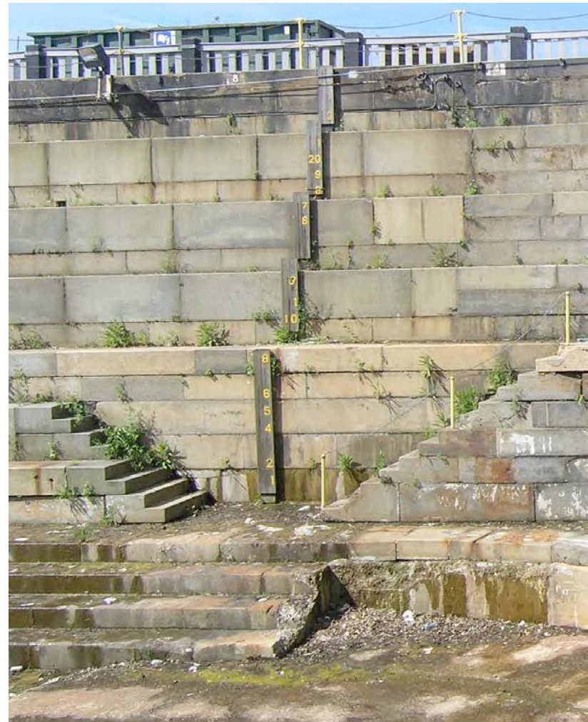
Fig. 17 Granite stairs at lower altars, west side of the chamber. Note that some deterioration has occurred in the lower steps (at lower right) where a section of the lower steps, extending around the arc of the dock's head, were removed and replaced with a low concrete wall that is now in poor condition.
