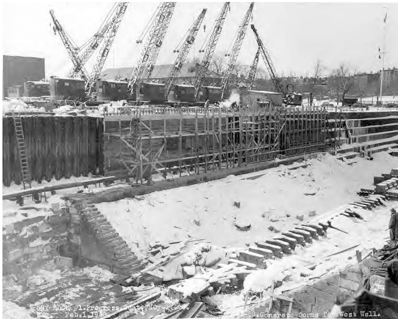
(B19) Photograph taken in February 1948, during reconstruction of the upper altars, on the west side of the chamber, showing sheet piling and formwork prior to pouring concrete. For about half the length of the dock, reinforced concrete altars replaced the original granite altars.
