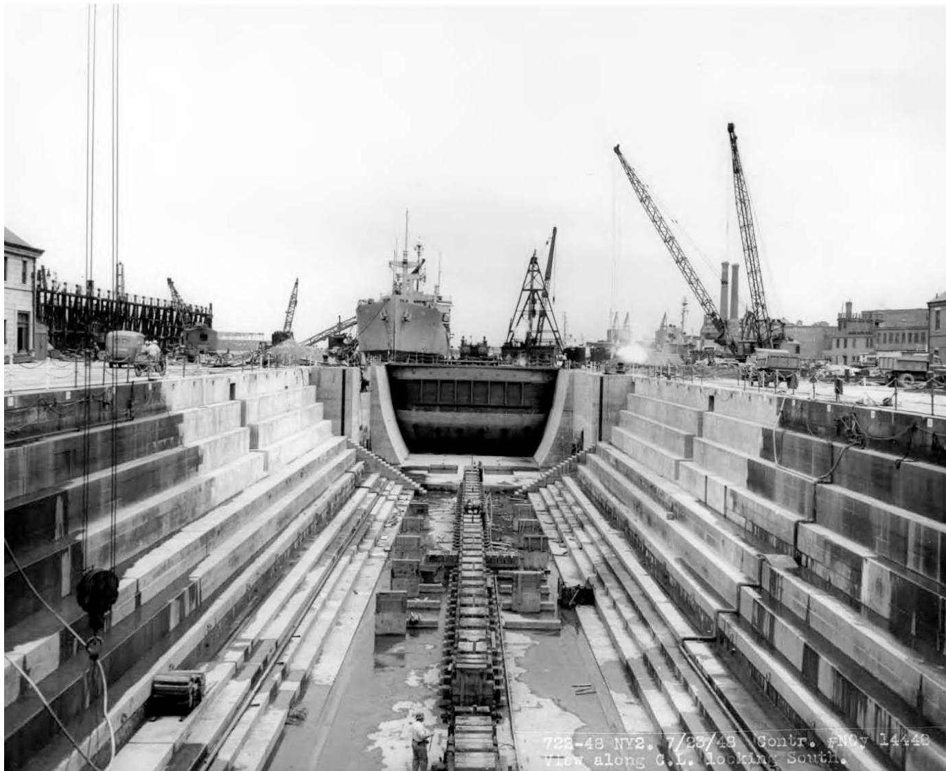
Fig. B-25 Photo BOSTS – 8796. July 23, 1948 view, looking south, showing the seaward extension, by which time most of the construction work was completed. Note that the 1901 steel Caisson is in place.
