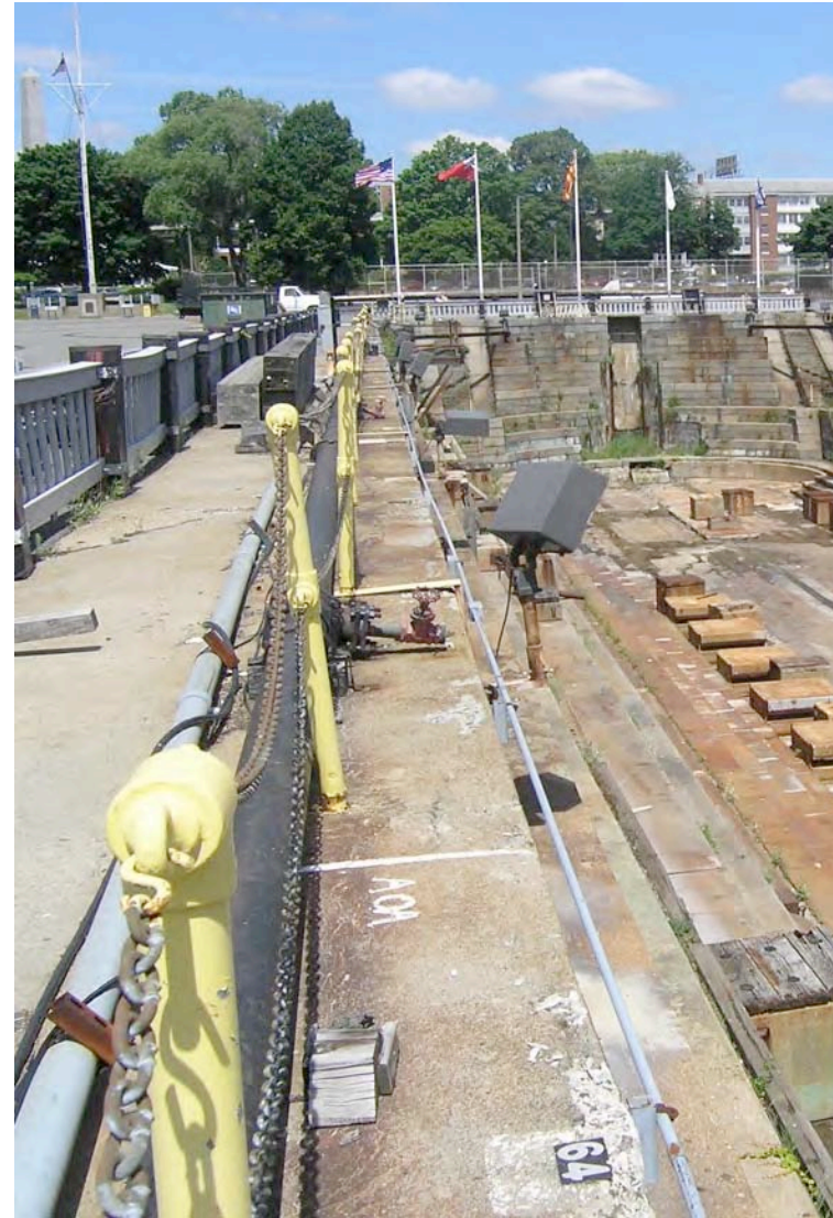
Fig. 34 View of pipes, electric cable, and floodlights along the west side of the dock.
