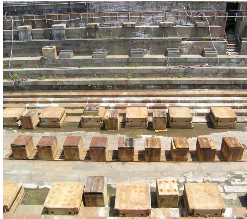
Fig. 31 View of concrete keel blocks showing the three different types of blocks.
