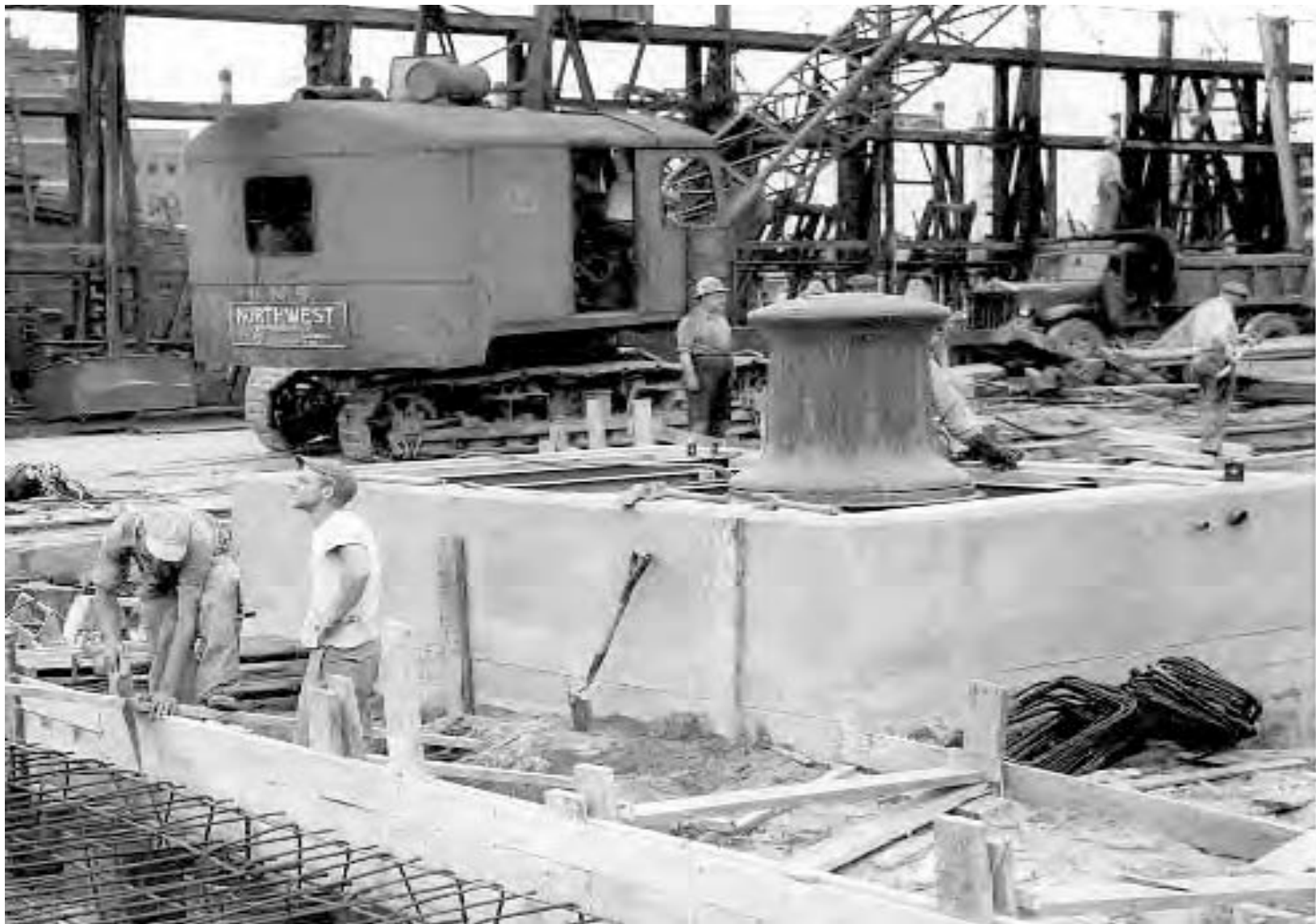
Fig. B-24 Photo BOSTS – 8796. July 1948 view looking southeast at relocated Capstan 3, including the capstan barrel, which rests on top of the newly constructed capstan pit.
