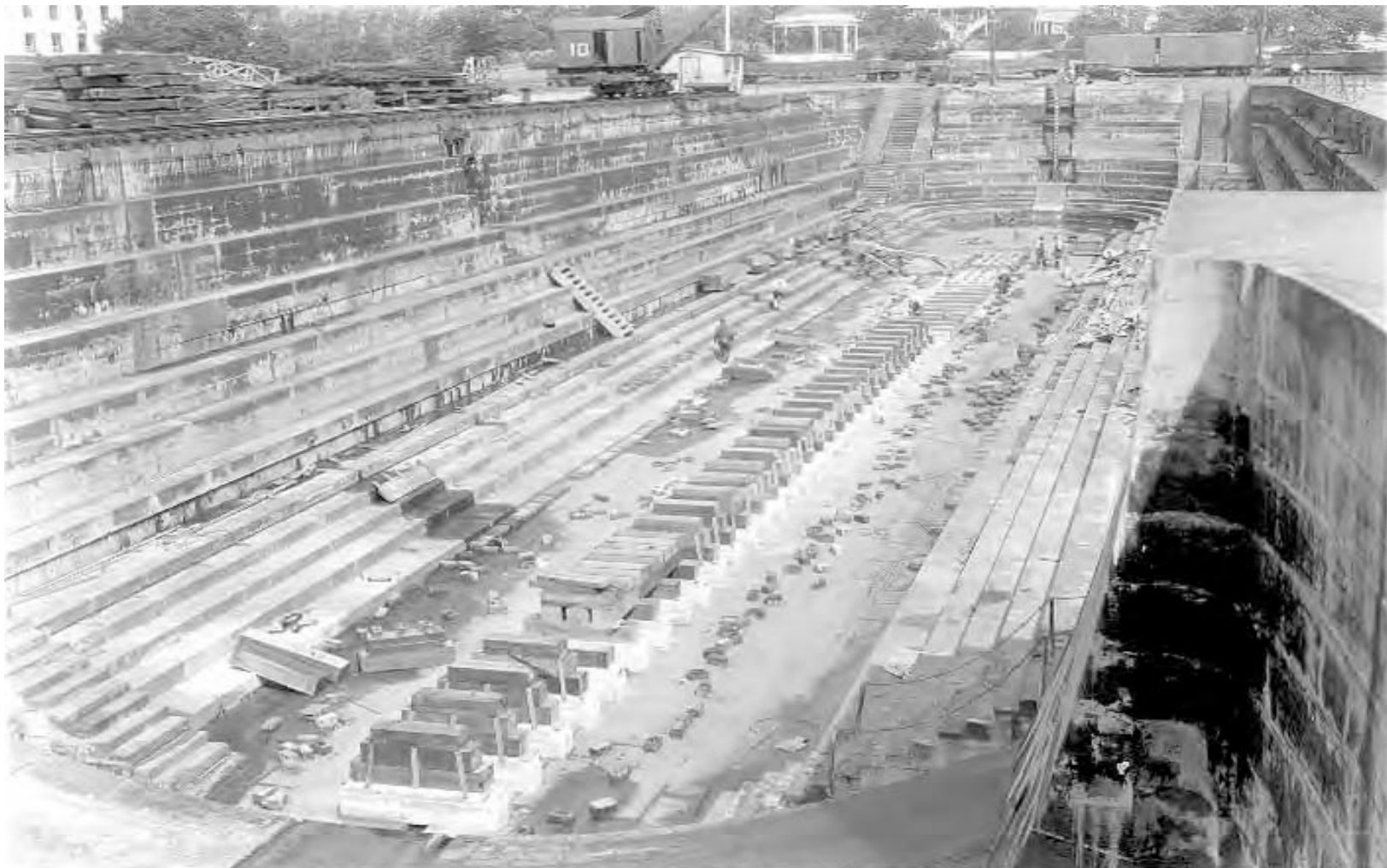
Fig. B-10 Photo BOSTS – 8793. View of Dry Dock I, from 1930, looking northwest, toward the head of dock, with the turning basin in the foreground. Note that at the middle of the dock, on the west side, a wooden stairway was located above the lower altars and provided access to the dock's floor. Note also that a concrete keelson is being constructed on he granite floor near the head of dock.
