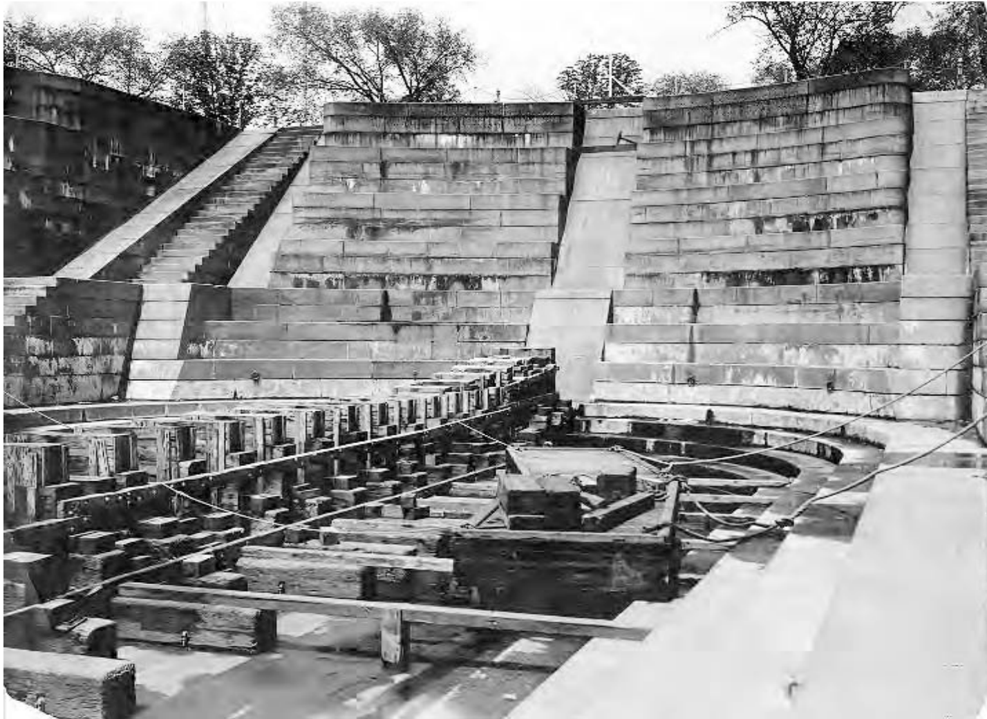
Fig. B-8 Photo BOSTS – 8790, c1900-c1920. View of the head of Dry Dock I, looking northwest. The center slide and adjacent altars are intact, as are the curved granite stairs that lead to the dock's floor.
