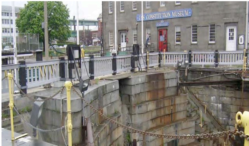
Fig. 28 View of safety fencing, with wood posts and composite railing, at head of dock, looking northeast. In the foreground is the older stanchion and chain fence, with the stanchions painted yellow.
