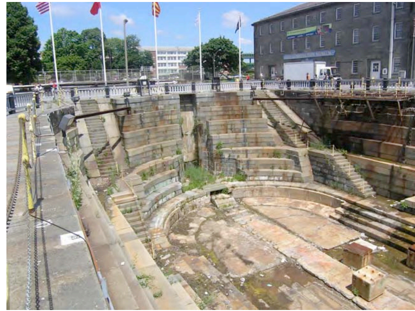
Fig. 7 View of floor at head of dock, showing the concrete slab and concrete ties that extend along the centerline of the dock.
