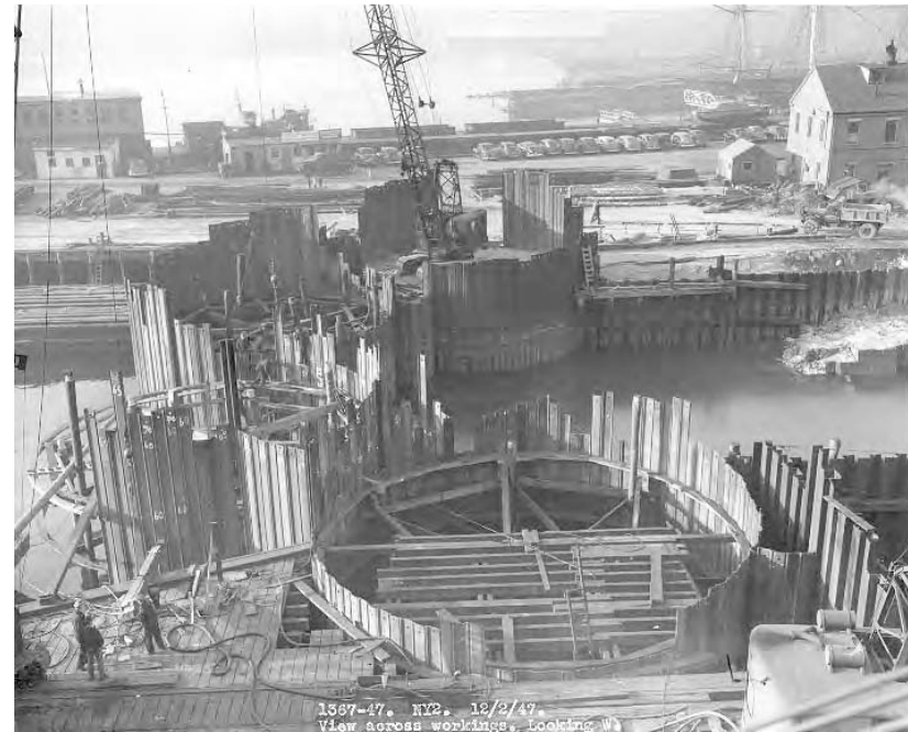
(B17) View looking west, showing the construction of the circular cofferdams in December 1947.
