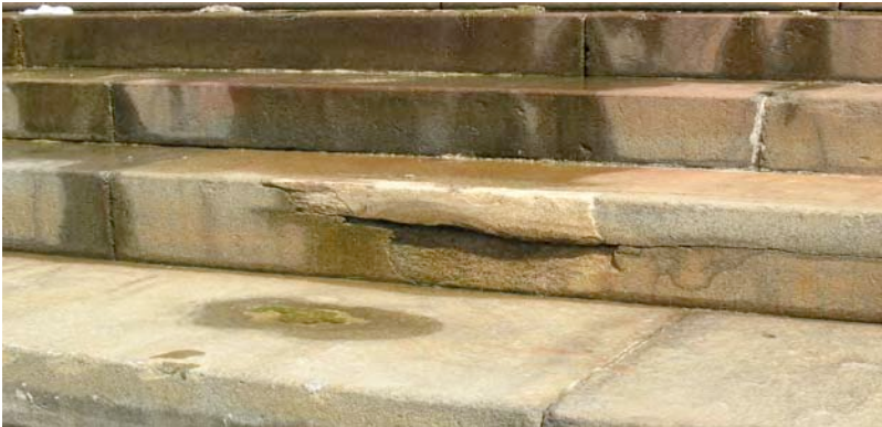
Fig. 10 Detail of cracked and broken granite block in step-back along the west wall that has been repaired with concrete.
