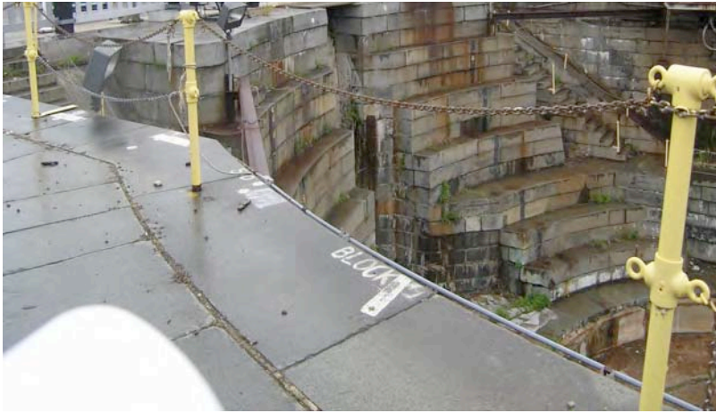
Fig. 18 Detail of coping on the west side near the head of the dock, where the original granite remains in place.
