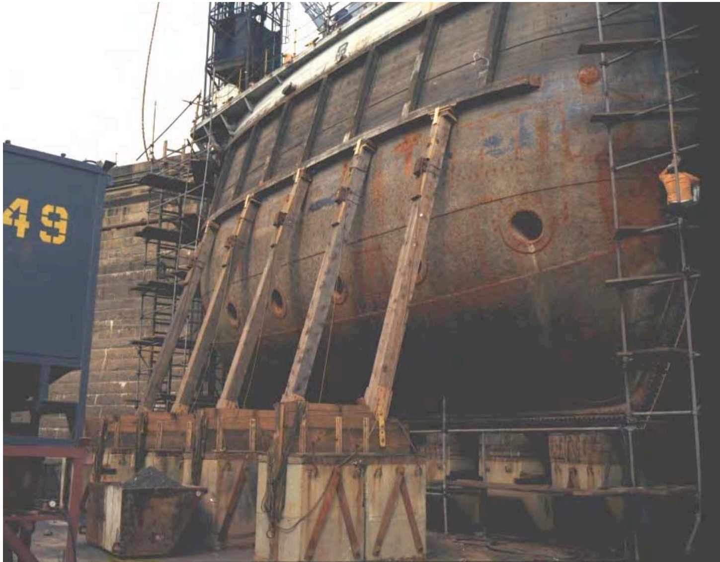
Fig. B-30 Photo BOSTS – 8805. September 13, 1972 view at Dry Dock 3 at South Boston of the steel Caisson undergoing its last renovation before closure of the Navy Yard.
