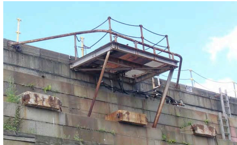
Fig. 5 View of steel platform on west side of the dry dock.
