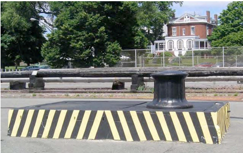
Fig. 2 View of Capstan 2 at the head of dock. This is one of three electric-powered capstans dating from 1942.
