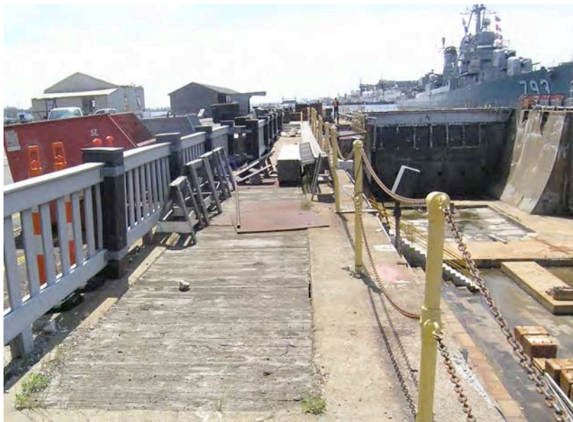
Fig. 15 Detail of blocked entrance to the chamber of Stair 6, near the middle of the dock.
