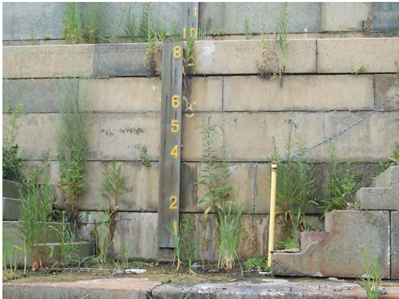
Fig. 32 Detail of draft gauge [file Dry Dock 8/10/05; #6612]
