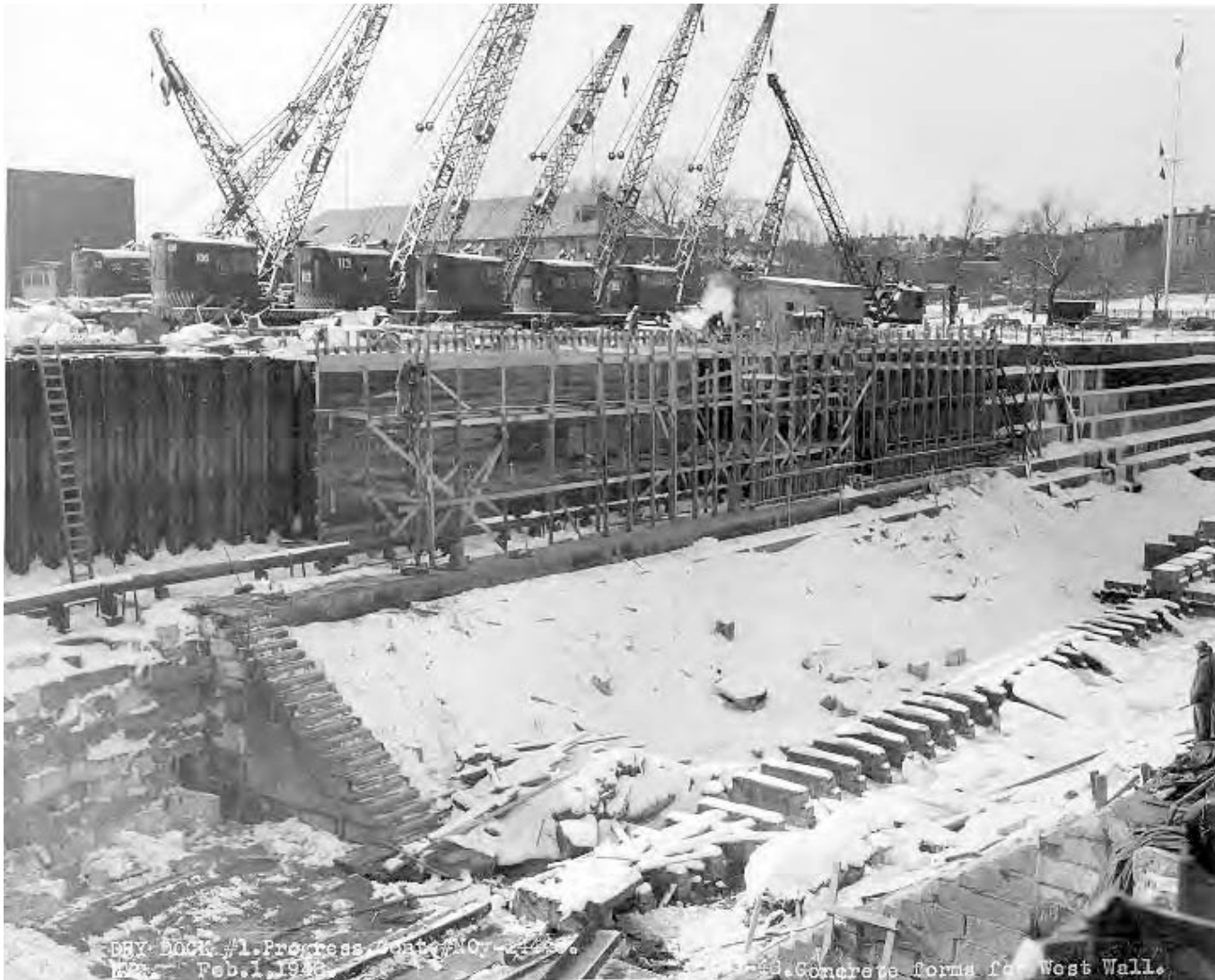
Fig. B-19 Photo BOSTS – 8796. February 1, 1948 view looking northwest of the reconstruction of the west wall. The granite blocks, below altar #4 (covered with debris and snow in this image), were retained, while reinforced concrete was used in reconstructing the walls above altar #4.
