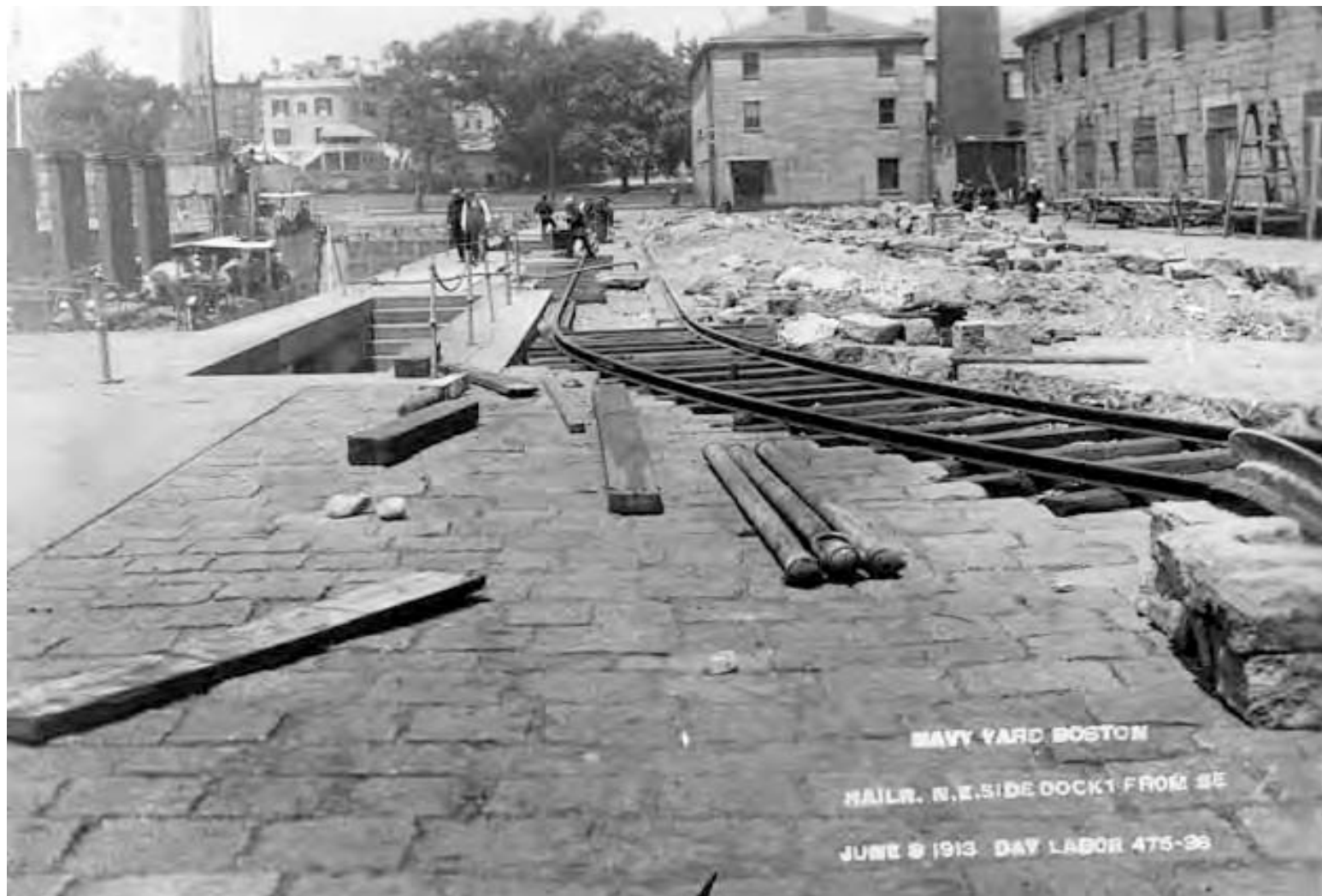
Fig. B-6 Photo BOSTS - 8791, June 9, 1913. Day laborers at work on the crane tracks on the east side of the dock. Note the stairway at the center of the dock that leads to the broad altar below. This access to the stairway is now blocked off.
