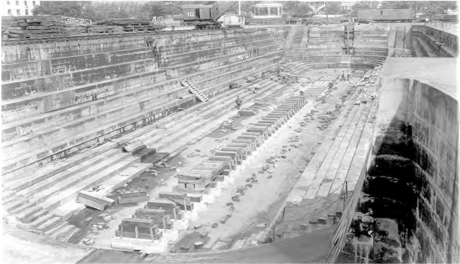
(B10) View of Dry Dock I, from 1930, looking northwest, toward the head of dock, with the turning basin in the foreground. Note that at the middle of the dock, on the west side, a wooden stairway was located above the lower altars and provided access to the dock's floor.
