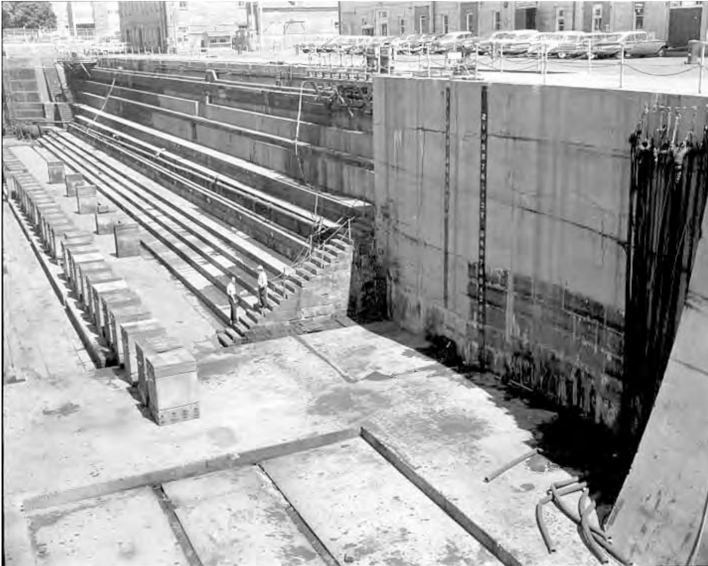
Fig. B-27 Photo BOSTS – 8800. June 1960 view of east wall at Stair I prior to the construction of the new tunnel intake and relocation of the stair. Note that the propeller pit had been enlarged, but retained its uniform edges, unlike the later expansion that drilled away additional sections of the concrete slab, leaving jagged edges that are visible today.
