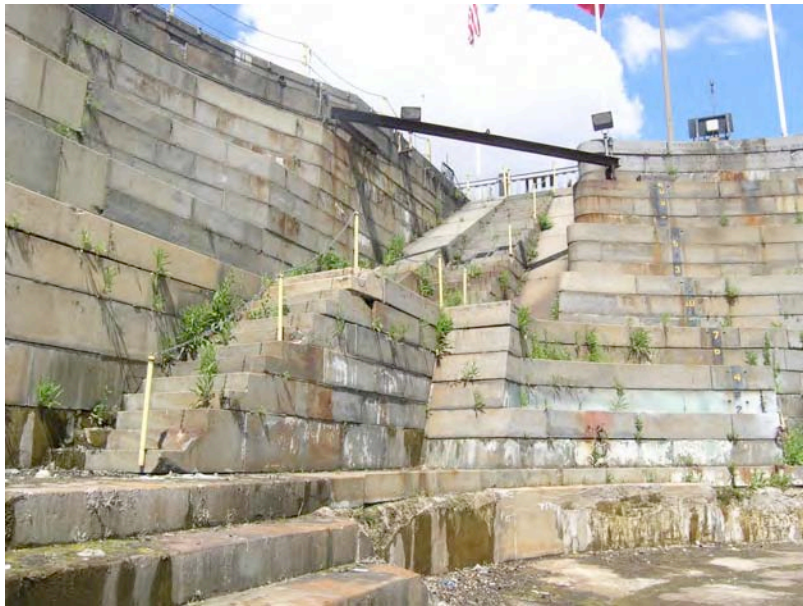
Fig. 13 Lower flight of Stair 3, on west side near the head of dock. Note that the three step-backs of the arc at the head of dock have been removed and replaced with a concrete wall that is now deteriorated.
