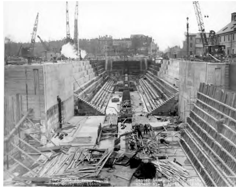
(B21) View of seaward extension of Dry Dock 1, looking north, April 1948.
