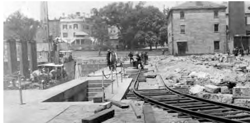
(B6) Detail from historic photograph from 1913, showing the opening at the coping level to Stair 5, on the east side of the dock.
