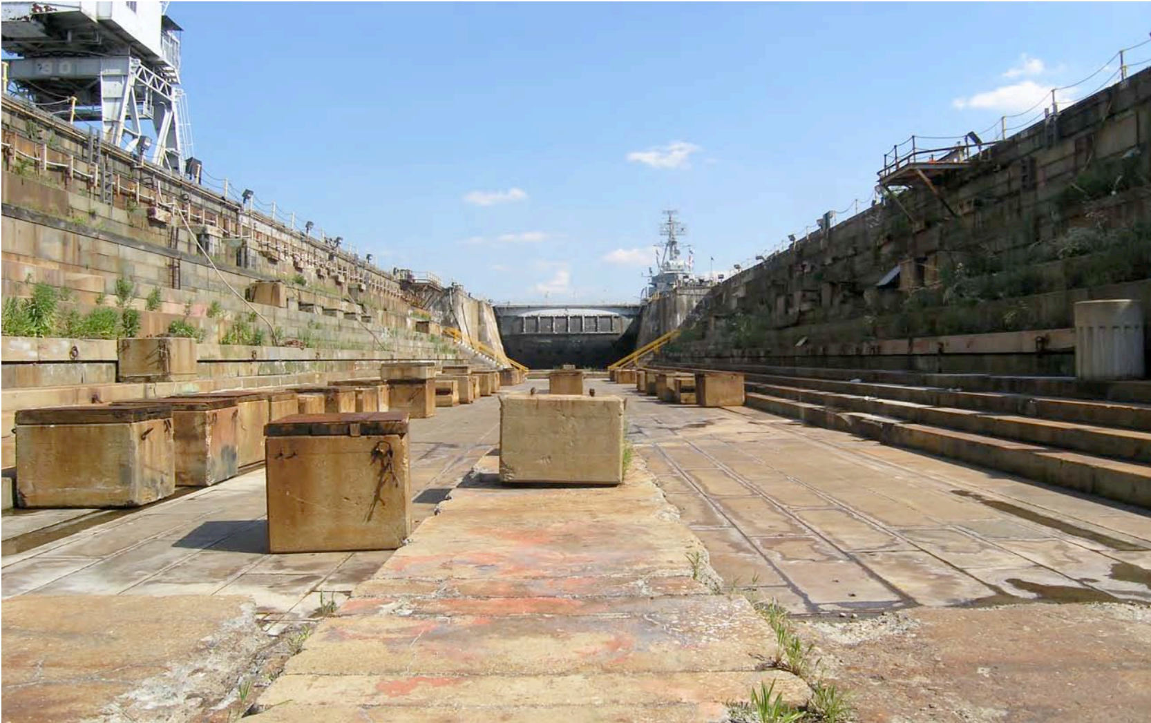
Fig. 24 Granite floor and keel blocks, looking south toward the steel caisson.
