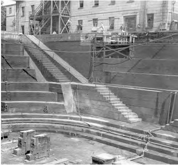
(B13) Detail from a photograph taken in August 1946, showing granite stairs (Stair 4) on the east side of the head of the dock. Located above the stairs is a wooden platform, replaced in the 1950s with a steel platform. Note the absence of fixed utility lines that were installed a few years later along with the steel platforms.
