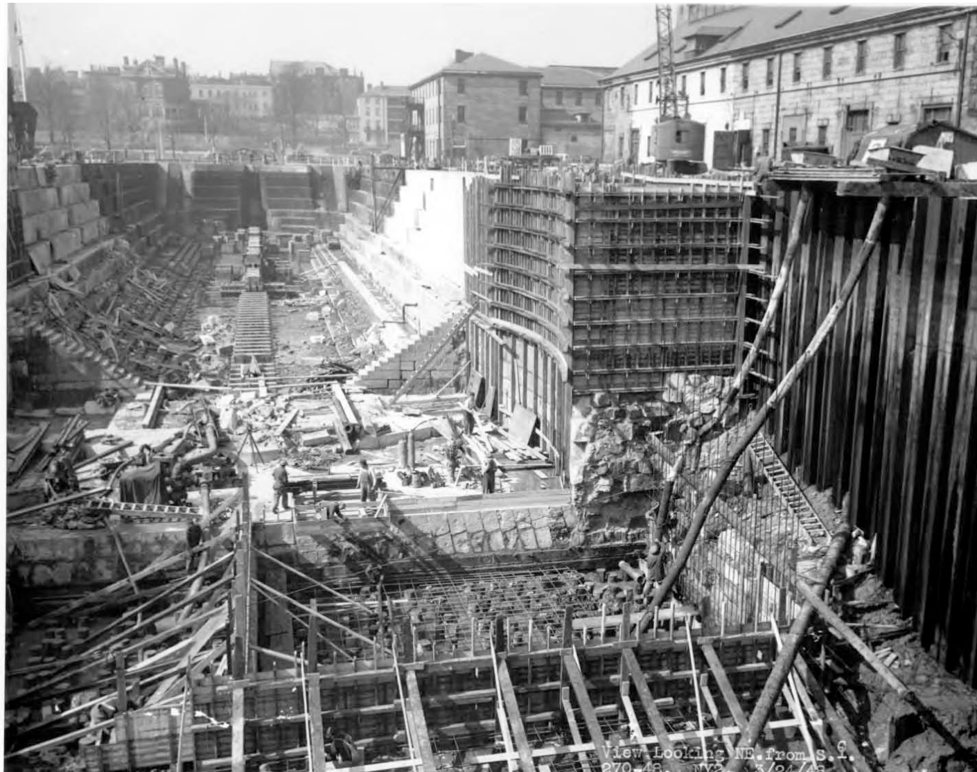
Fig. B-20 Photo BOSTS – 8796. March 24, 1948 view looking north showing the construction of the seaward extension. In the foreground is form work and reinforcing steel for the floor and propeller pit. Visible beyond are the recently completed reinforced concrete walls and altars that replaced the original granite masonry.
