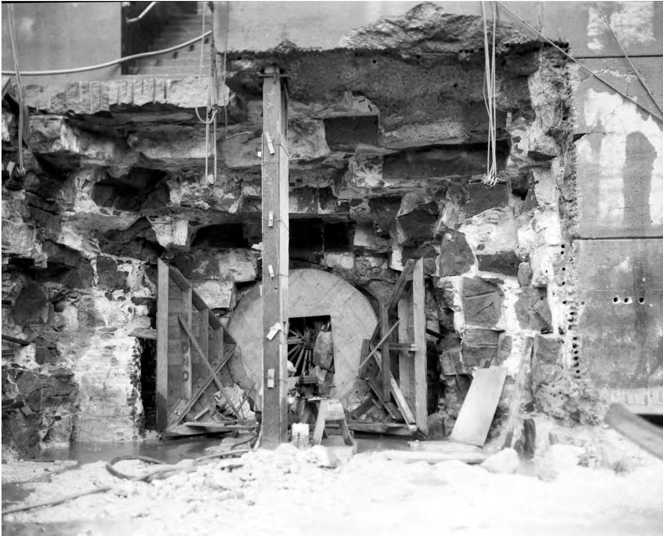
Fig. B-29 Photo BOSTS – 8800. November 1, 1960 view through a section of the west wall for the new tunnel intake. Workers blasted out some of the original granite masonry. A concrete-lined culvert was then built which decreased the amount of time needed to dewater the chamber. This photo shows some of the formwork for the new culvert. Note the stair above, the lower portion of which was demolished, prior to constructing a reinforced concrete stair to the left of this photo.
