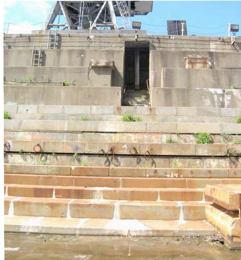
Fig. 16 Detail of entrance to the chamber of Stair 6, near the middle of the dock on the west side. One of the timber posts that supports the timber planking, which blocks off the ground-level entrance to the stairway, is visible in the center.
