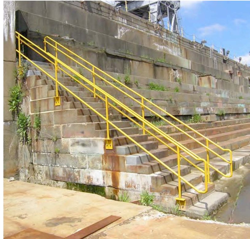
Fig. 14 Lower flight of Stair 2, on west side near the seaward extension. This original section of stair was preserved as part of the 2004 repairs of Dry Dock 1.
