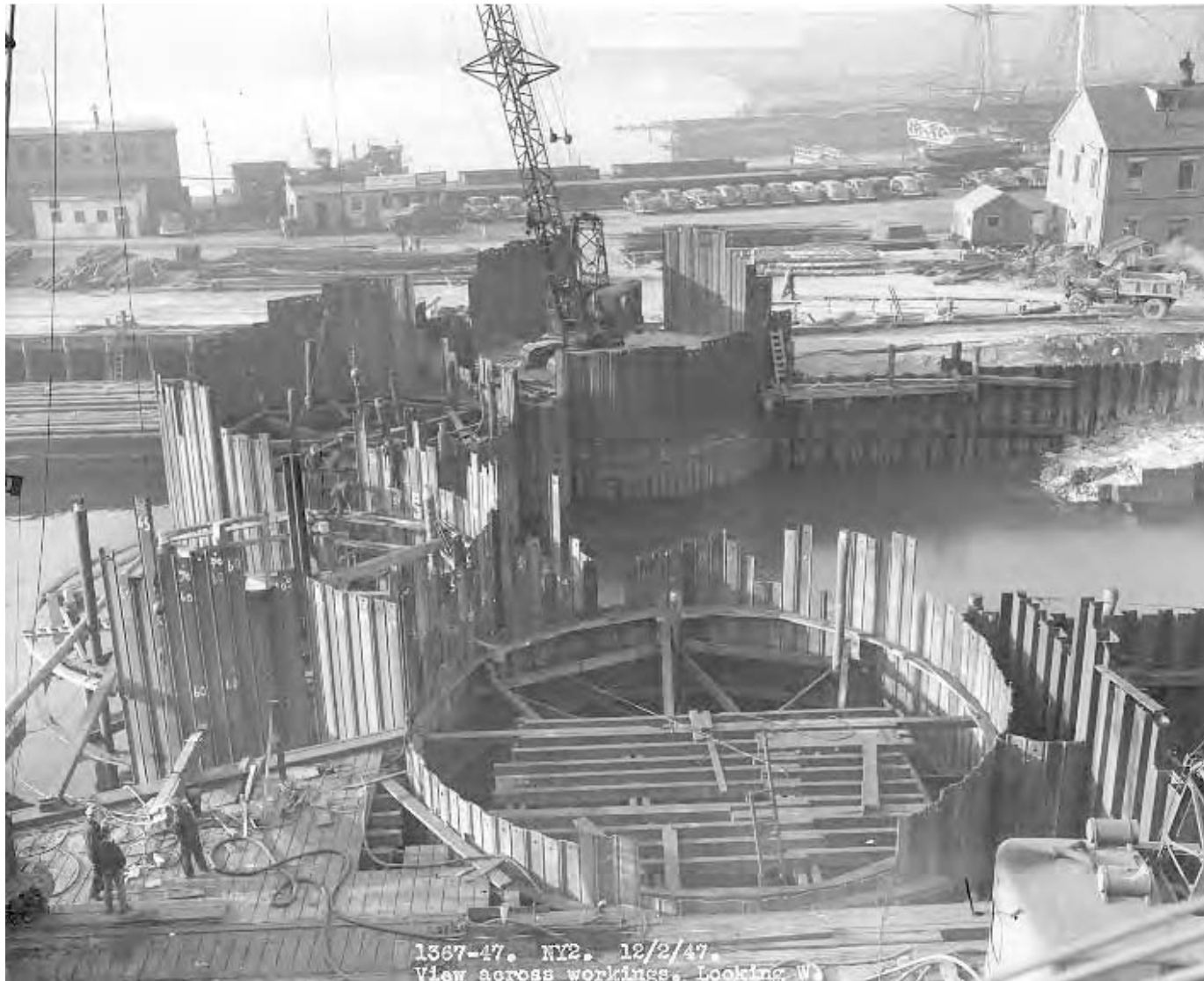
Fig. B-17 Photo BOSTS – 8796. December 2, 1947 view looking west at cofferdams needed to support construction of the seaward extension. Cofferdam in the foreground and that on the far opposite contain concrete vaults to house the dock’s electric capstans.
