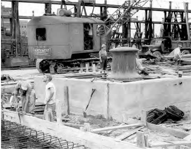
(B24) Photograph taken in July 1948, showing relocated Capstan 3, including the capstan barrel, which rests on top of the newly constructed capstan pit.
