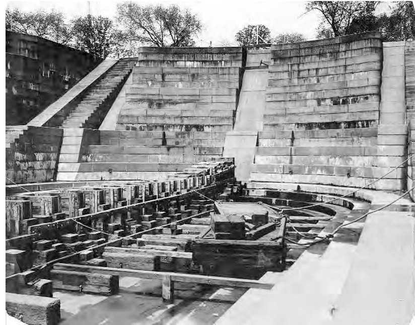
(B8) View of Head of Dock, taken prior to 1907, when the initial modification to the center slide was carried out,. At the time of this photograph the dock's head appeared much as it did following the completion of the extension in 1860.
