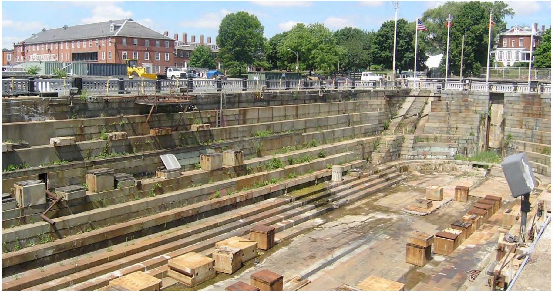
Fig. 9 View looking northwest toward the head of dock. Along the west side of the chamber, from left to right, may be seen the three major construction periods of Dry Dock I. At left are the concrete altars from 1947-1948; adjoining these concrete altars are the original altars of Quincy granite; the large blocks to the right are composed of Cape Ann granite, used to construct the altars as part of the inland extension completed in 1860.
