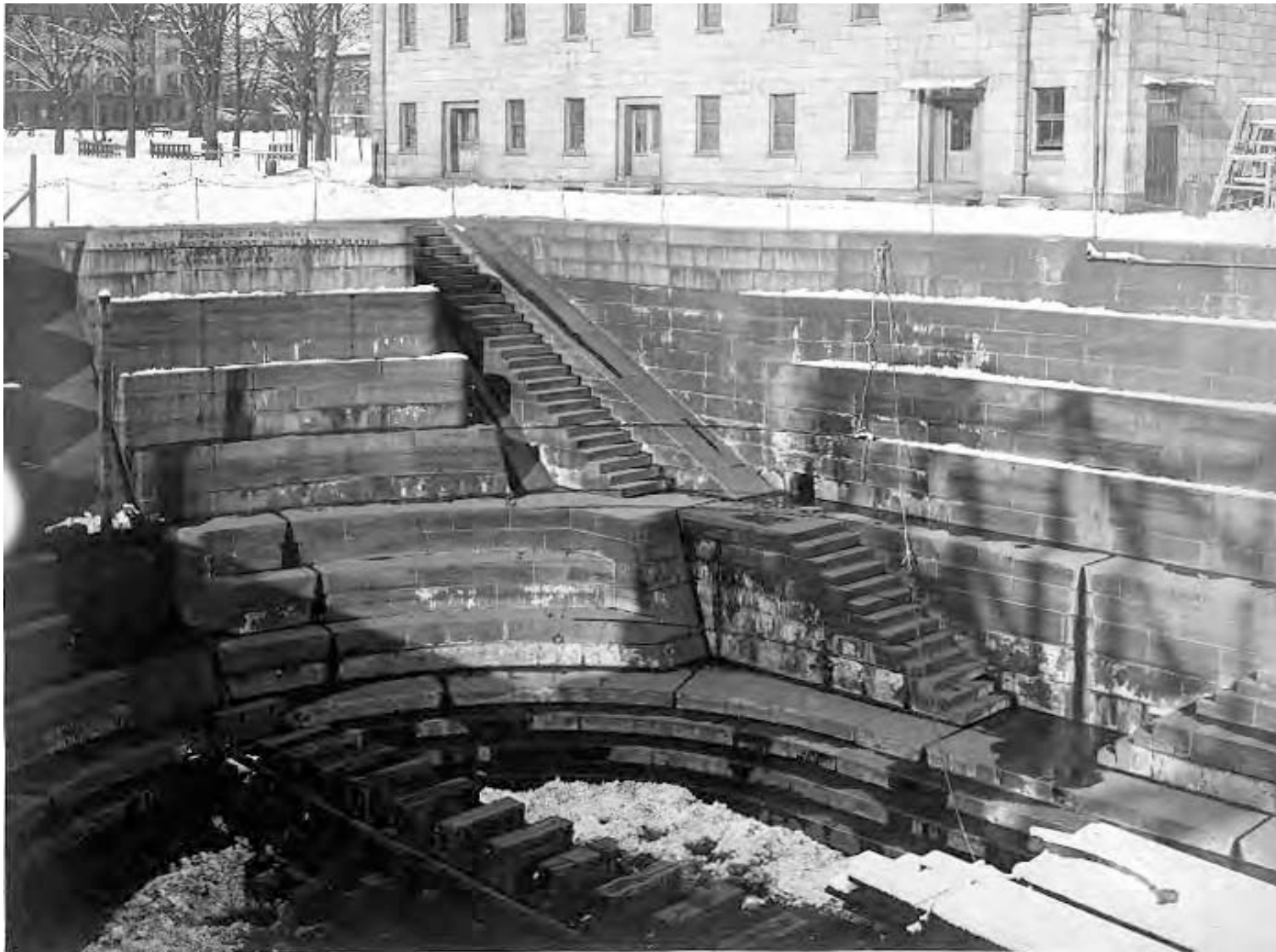
Fig. B-9 Photo BOSTS – 8790, c1910-c1920. View of the head of Dry Dock I, looking northeast. Note that the original iron stanchion and chain fencing is around the perimeter of the dock but there is no fencing on the stairs.
