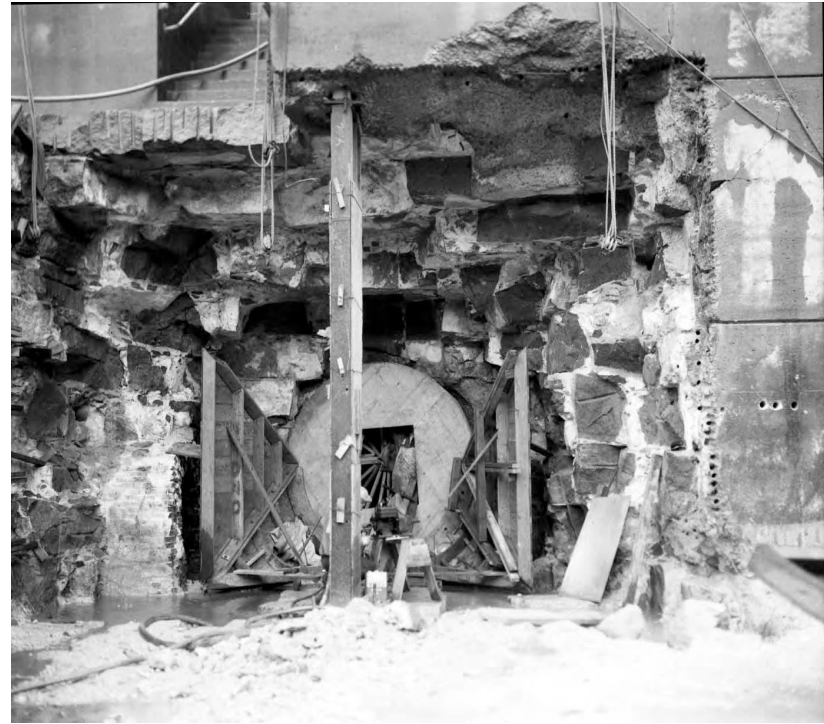
(B29) Taken in 1960, this photograph shows the construction of the dewatering tunnel intake, involving the removal of granite blocks and the building of a concrete-lined tunnel.
