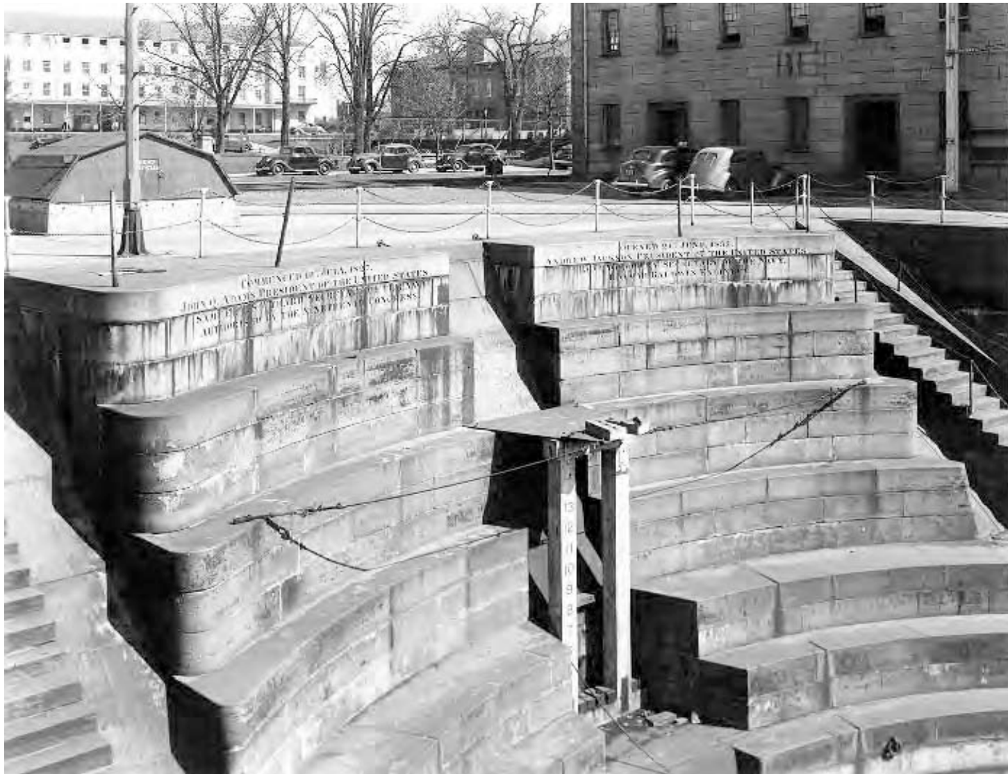
Fig. B-II Photo BOSTS – 8792. View in 1939 looking northeast at head of dock. At the top, flanking the center slide, is the original inscription in the granite, acknowledging the originators and builders of the dry dock.
