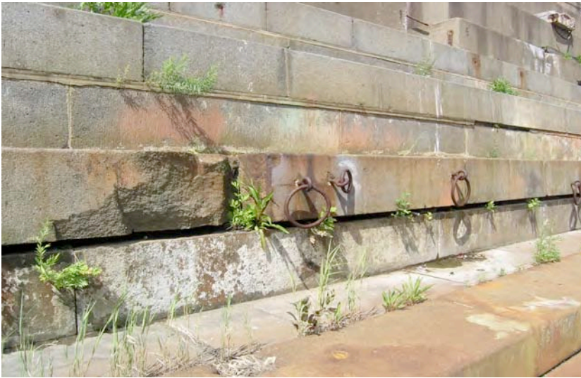
Fig. 4 Detail of iron rings along west wall of dry dock
