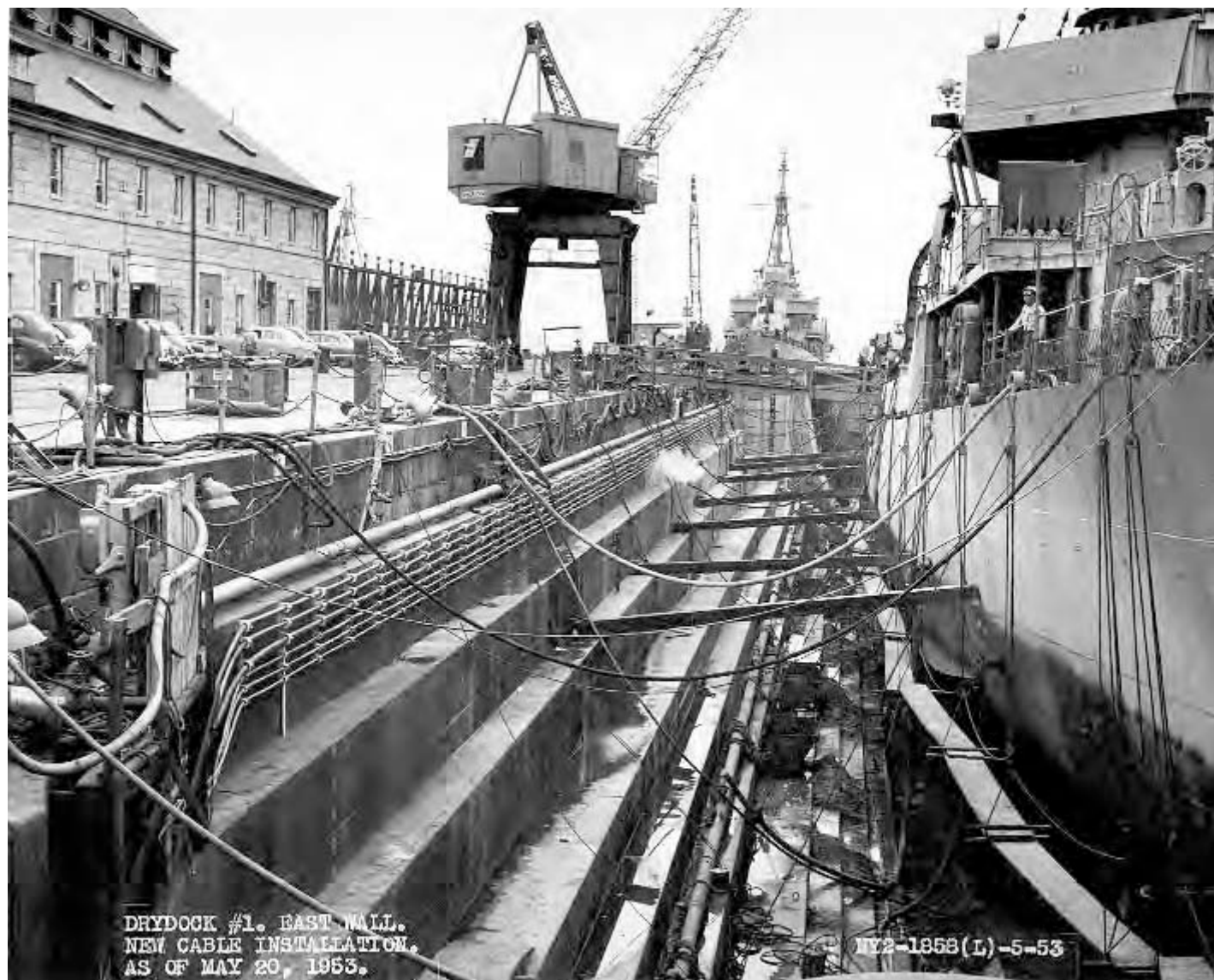
Fig. B-26 Photo BOSTS – 8797. May 20, 1953 view of the east wall of Dry Dock I, looking south, showing recently installed electrical cables, a portion of which remains today.
