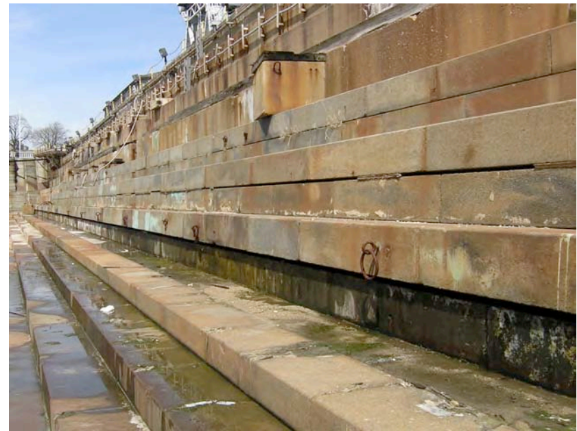
Fig. 12 View looking north showing the east side of the chamber. The lower altars and stairs of granite were retained, while the upper altars were replaced with reinforced concrete nearly half the length of the dock.
