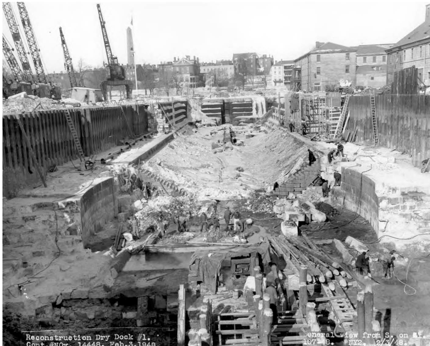
Fig. B-18 Photos BOSTS – 8796. February 3, 1948 view looking north during the reconstruction of a large section of the original granite chamber. This reconstruction work was carried out as part of the seaward extension and entailed the installation of steel sheet piling, a reinforced concrete backing (in place of the original rubble masonry backing), and reinforced concrete walls (in place of the original granite blocks).
