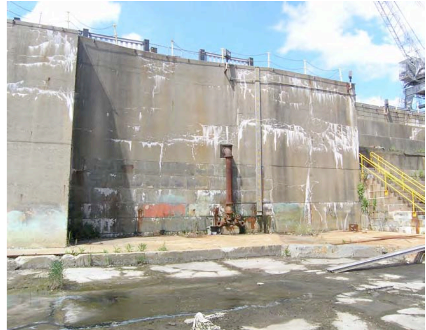
Fig. 25 View of the west wall, showing the condition of the concrete. This was part of the work carried out for the seaward extension in 1947-1948. Note that some of the lower courses of granite, which date from the original construction of Dry Dock 1, that were retained. The rusting steel pipe and valve structure in the center was part of the improved hydraulic system installed at the time of the seaward extension.
