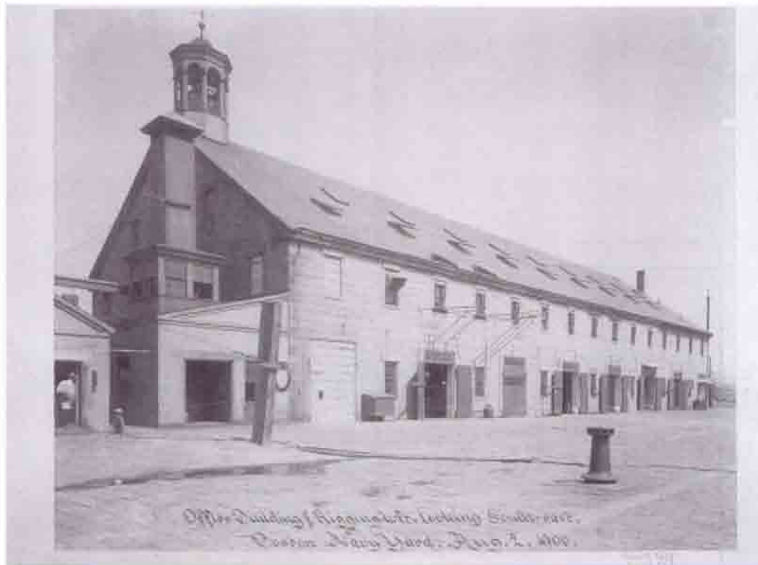
Fig. B-6 Photo "Office Building and Rigging Left, looking South-east; Boston Navy Yard, Aug. 2, 1900." CNY Archives (BOSTS 9298 & BOSTS 9583 & BOSTS 10047) Looking southeast: Shows the entire west and north elevations. On the north elevation note the muster bell, and galvanizing shop (with monitor and chimney not shown on the original plans for the shop). On the west elevation note the awnings on some of the second story windows (designated as offices on the floor plans), the blueprint drying racks at the second floor windows (designated as the Printing Room on the floor plans), the rain diverters over the blueprint drying racks, 12/12 windows, northwest corner door and two window openings blocked in with granite (much lighter and cleaner than surrounding granite, suggesting recent installation), "Porch A" vestibule at southernmost door, and skylights open for ventilation.
