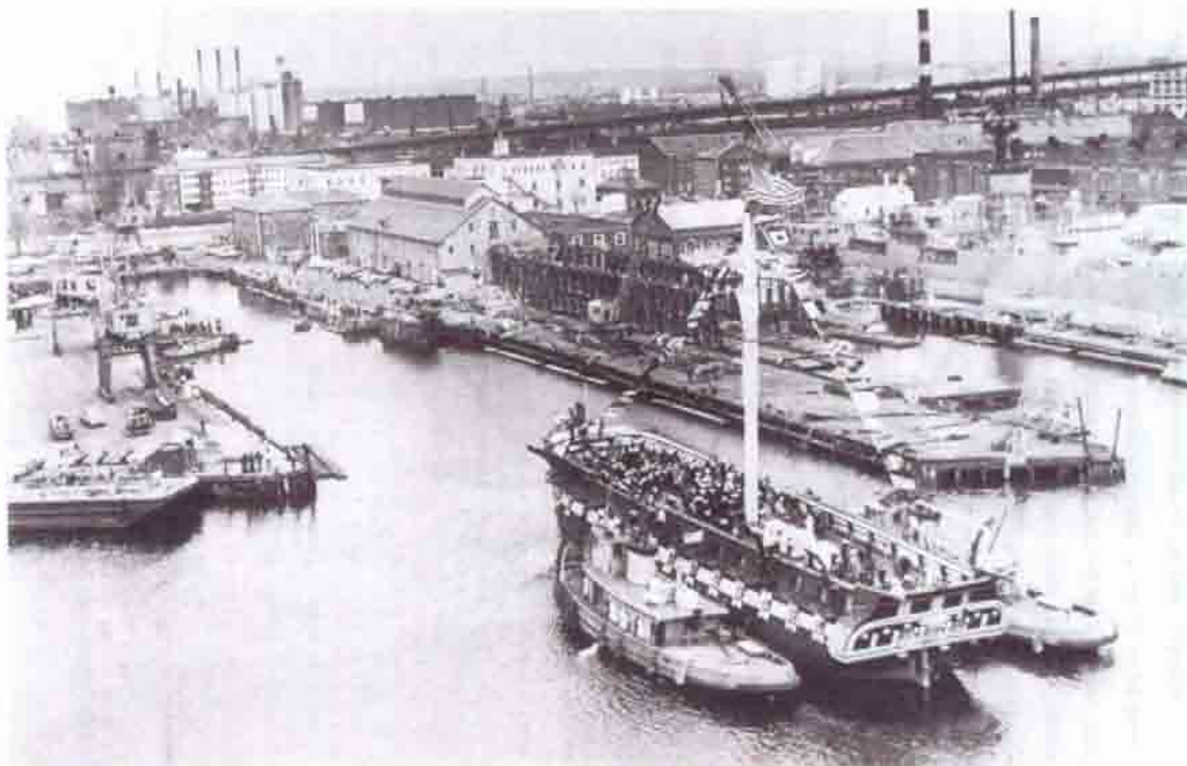
Fig. B-55 Photo of USS Constitution approaching Dry Dock 1, April 17, 1971 (copied from Black, 1988, p.797). Looking northeast from over the water. Dormer and six skylights visible on west roof.
