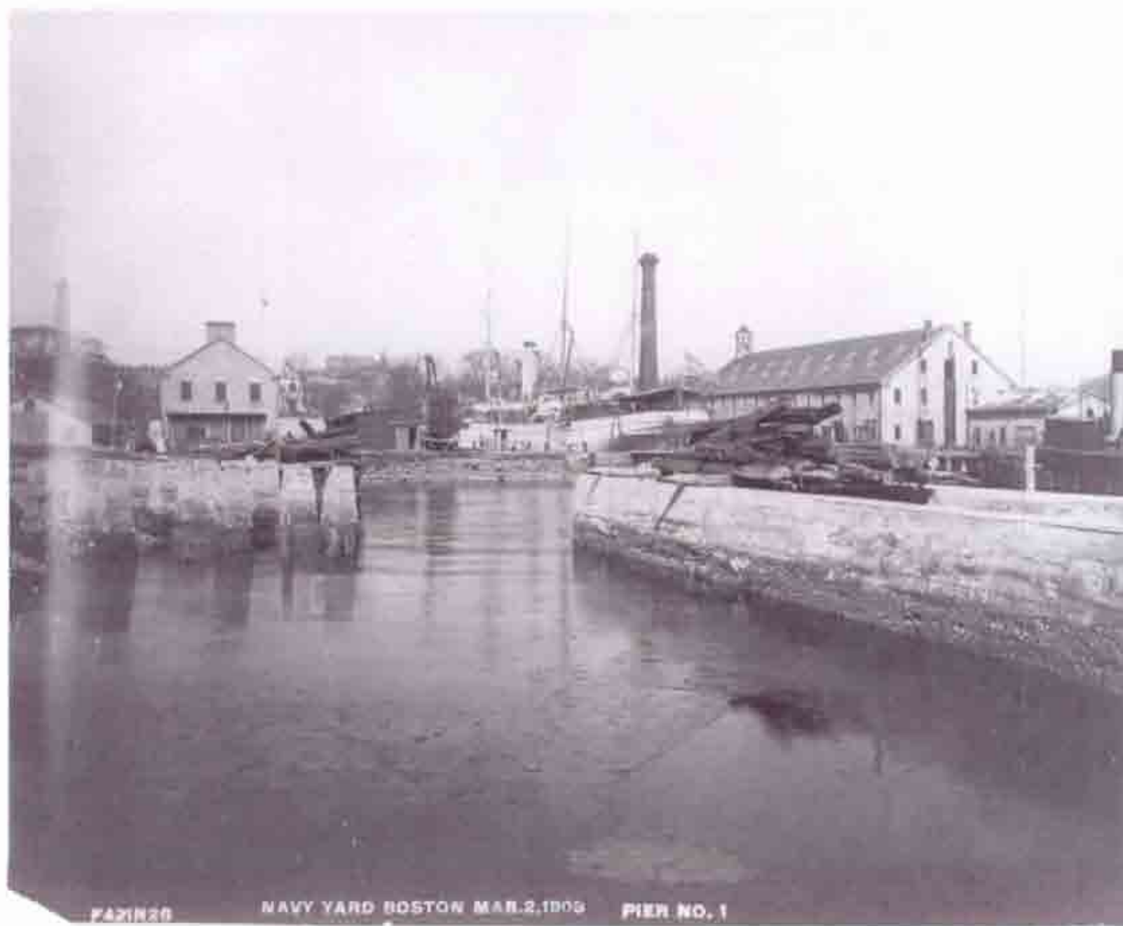
Fig. B-8 Photo "F421N28 Navy Yard Boston Mar. 2, 1903 Pier No. 1. CNY (BOSTS 8694). Looking northwest from the harbor. Shows most of south elevation and second floor and roof of west elevation. No apparent changes from the 1900 photographs.
