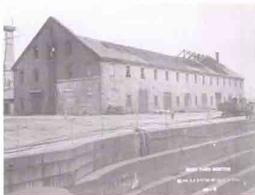
(B9) "NAVY YARD BOSTON BLDG 24 FROM W JULY 2 1913 24-B" Looking southeast. Shows the building after the 1910 fire and before the demolition of the roof and interior framing for reconstruction.
