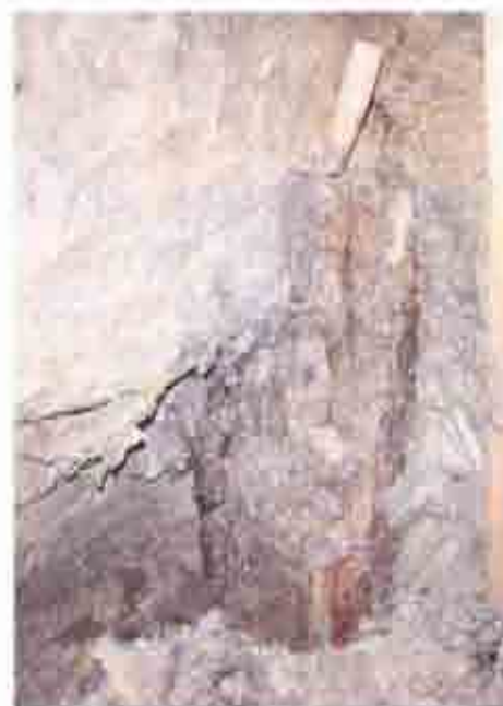
Fig. 37 Granite footing stones were discovered to have crushed the tops of each of the two wood piles discovered in Test Pit No. 1 during excavation in June 2002.
