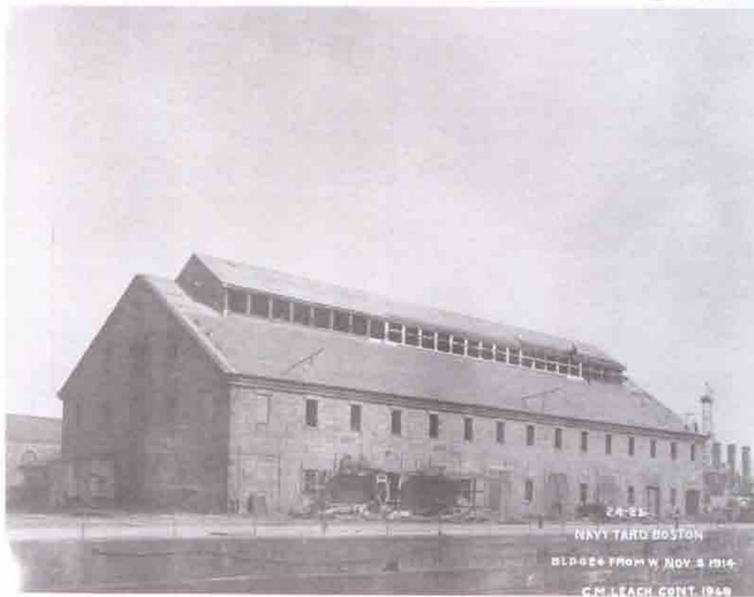
Fig. B-25 Photo "24-23 (note: this is not an entry mistake, both photos were labeled 24-23 - LH) NAVY YARD BOSTON: BLDG 24 FROM W NOV 3 1914 C. M. LEACH CONT. 1968". Exterior, looking southwest. New roof constructed with monitor. Slate not complete on main roof or monitor. Monitor window framing in progress. Windows not installed yet.
