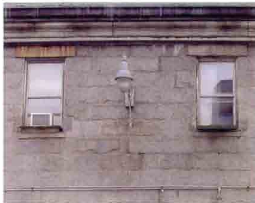
Fig. 6 Notches on either side of these windows just above the sills were infilled with granite after removal of blueprint-drying racks.
