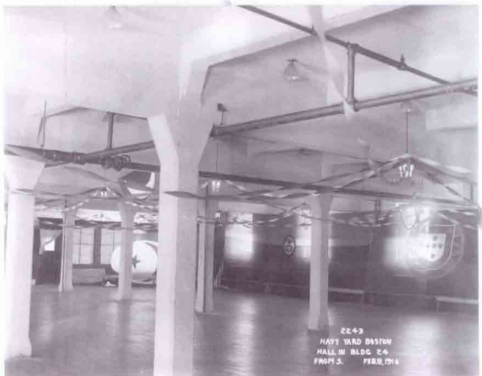
Fig. B-39 Photo "2243 NAVY YARD BOSTON HALL IN BLDG. 24 FROM S. FEB. 8, 1916". Second floor hall, looking north. Banners, lights and flags in place. Ceiling light fixtures and sprinkler system visible.
