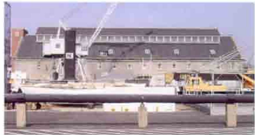
Fig. 1 West Elevation. Due to obstructions at ground level, a full view of the entire facade is not possible.
