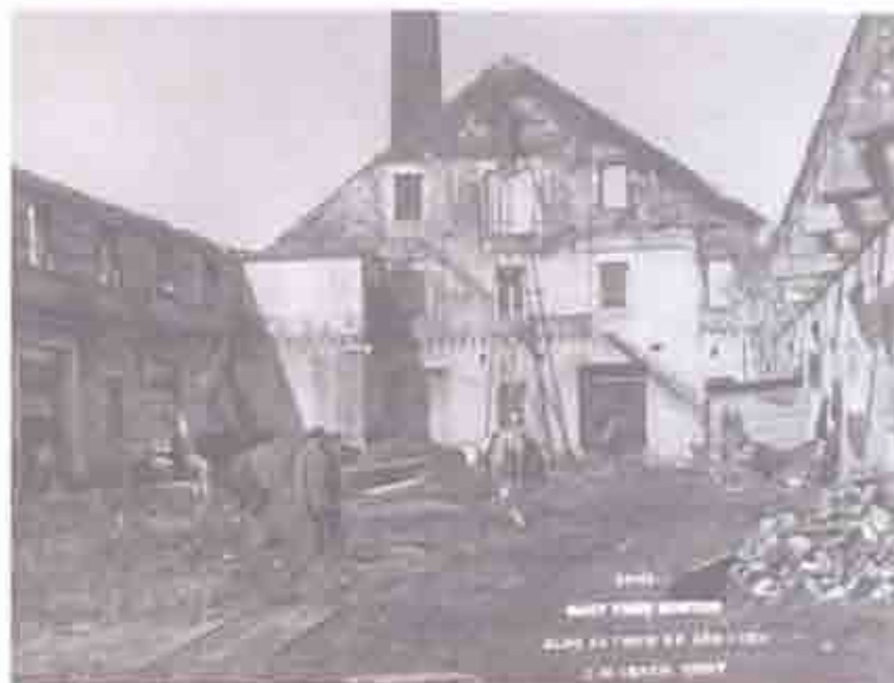
(B18) "24-17 NAVY YARD BOSTON BLDG 24 FROM SE APR 1 1914 C M LEACH CONT". Interior after the 1910 fire, looking north in a photo from 1913.
