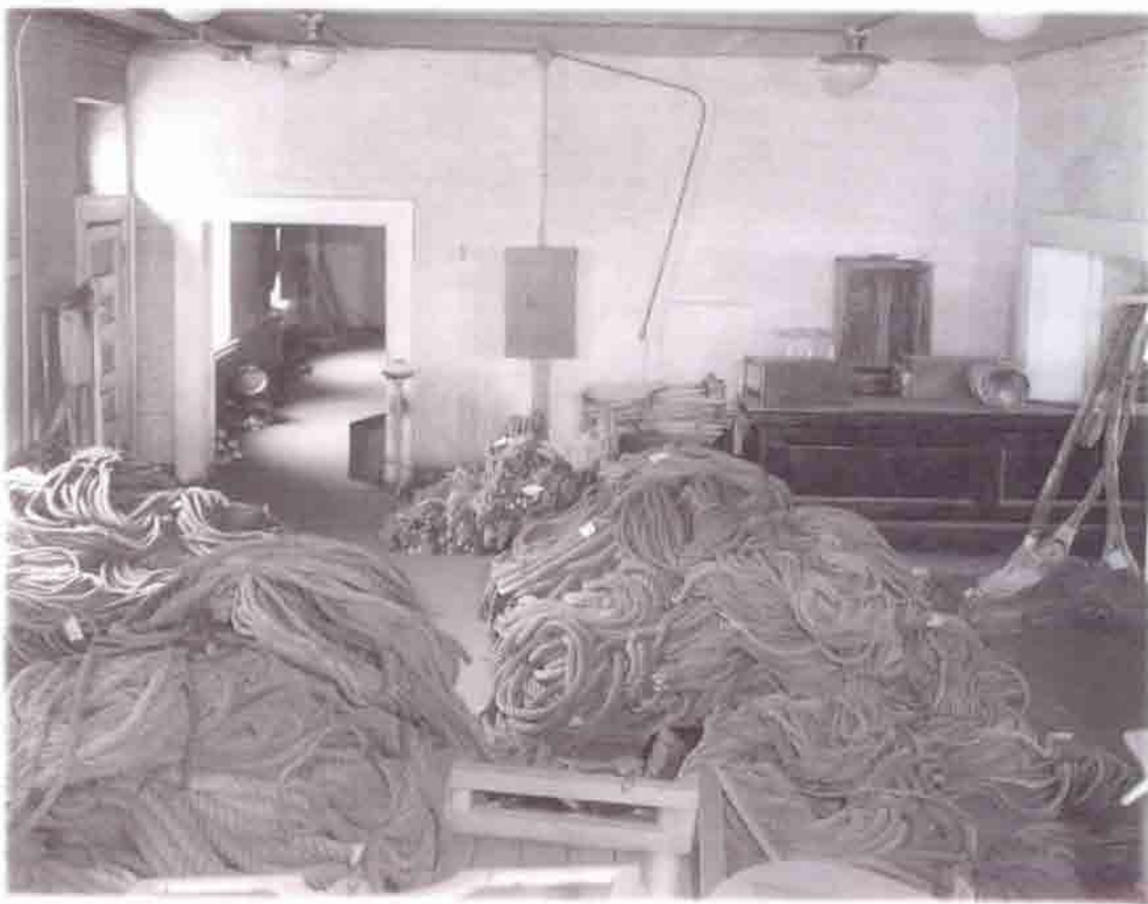
Fig. B-47 Photo "223-36 Mar 27-36 Constitution" in pencil on back. 1936. Interior photo, appears to be first floor. Note light fixtures.
