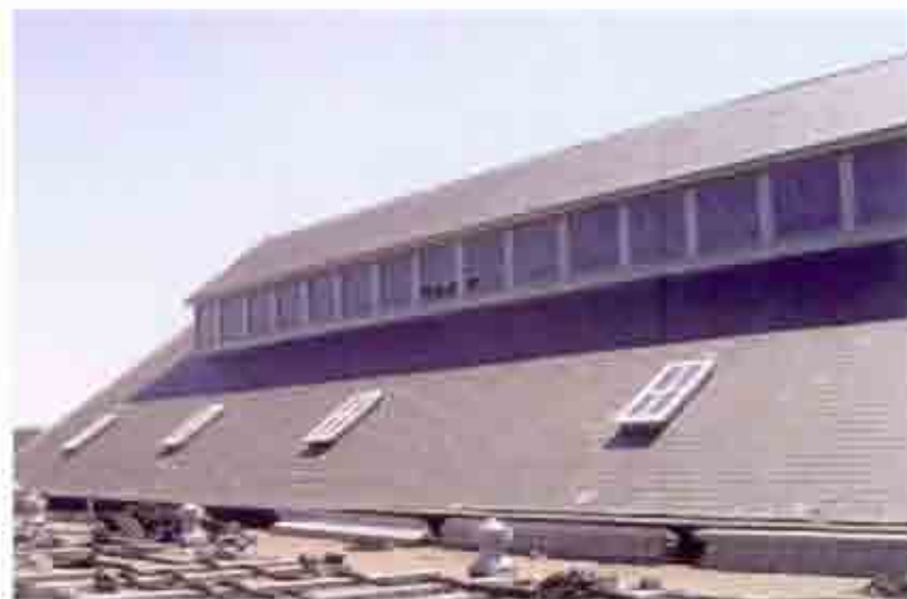
Fig. 11 The slate roof, installed in 1913-14, has been on the building longer than the original gable roof.
