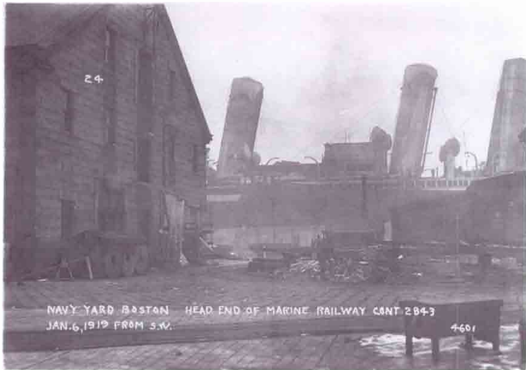
Fig. B-42 Photo "NAVY YARD BOSTON HEAD END OF MARINE RAILWAY CONT 2843 JAN. 6, 1919 FROM S. W. 4601". North elevation. First floor eastern most window lintel has been raised, probably as part of the work to install the marine railway. The vertical wooden slats have been removed from below the third floor opening.
