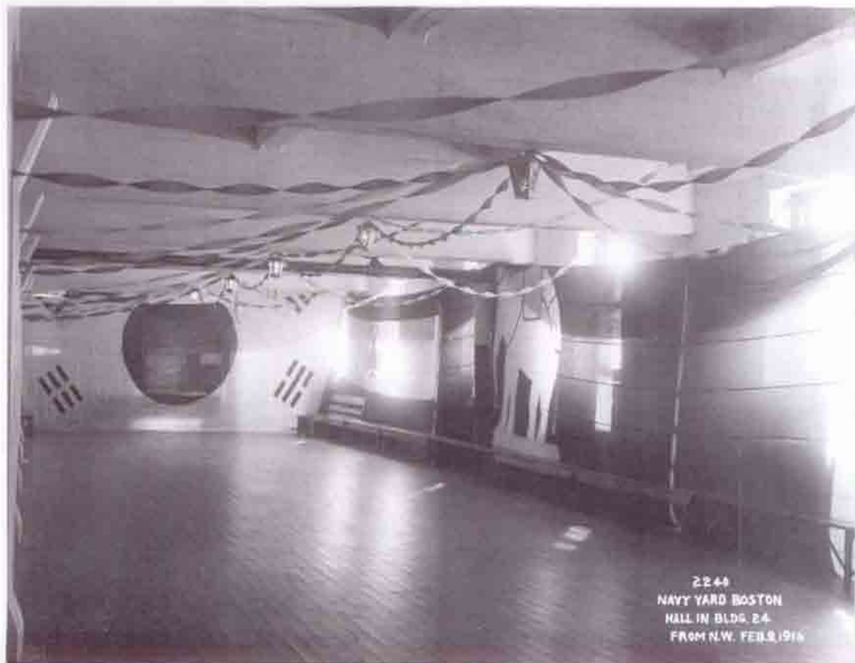
Fig. B-36 Photo "2240 NAVY YARD BOSTON HALL IN BLDG. 24 FROM N.W. FEB. 8, 1916". Second floor hall, looking southeast. Banners, lights and flags in place.
