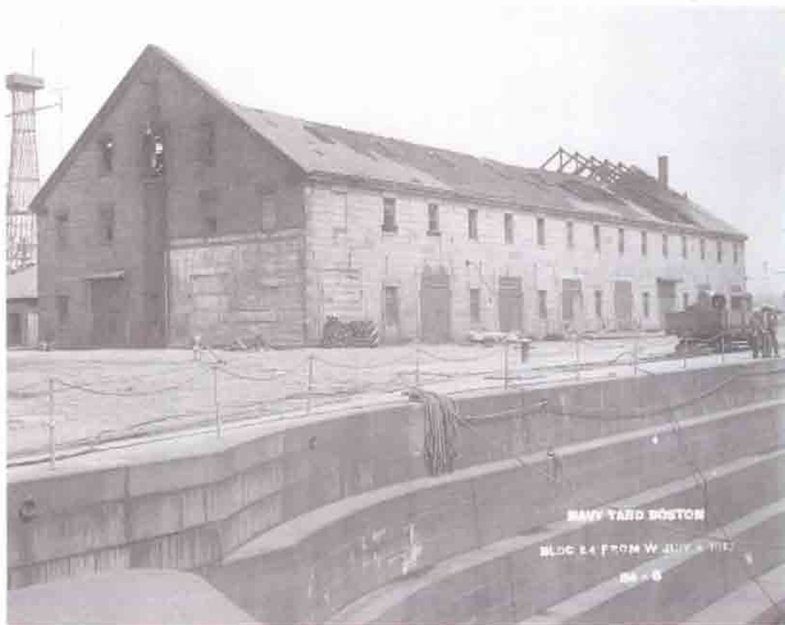
Fig. B-9 Photo "NAVY YARD BOSTON BLDG 24 FROM W JULY 2 1913 24-8". Looking southeast. Shows the building after the 1910 fire and before the demolition of the roof and interior framing for reconstruction. Note the ghosting of where the galvanizing shed was.
