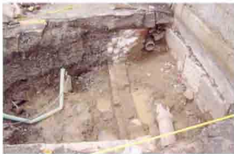
Fig. 36 During test pit excavation on Aug. 18, 2002, a brick wall was found at a depth of three feet, preventing further digging.
