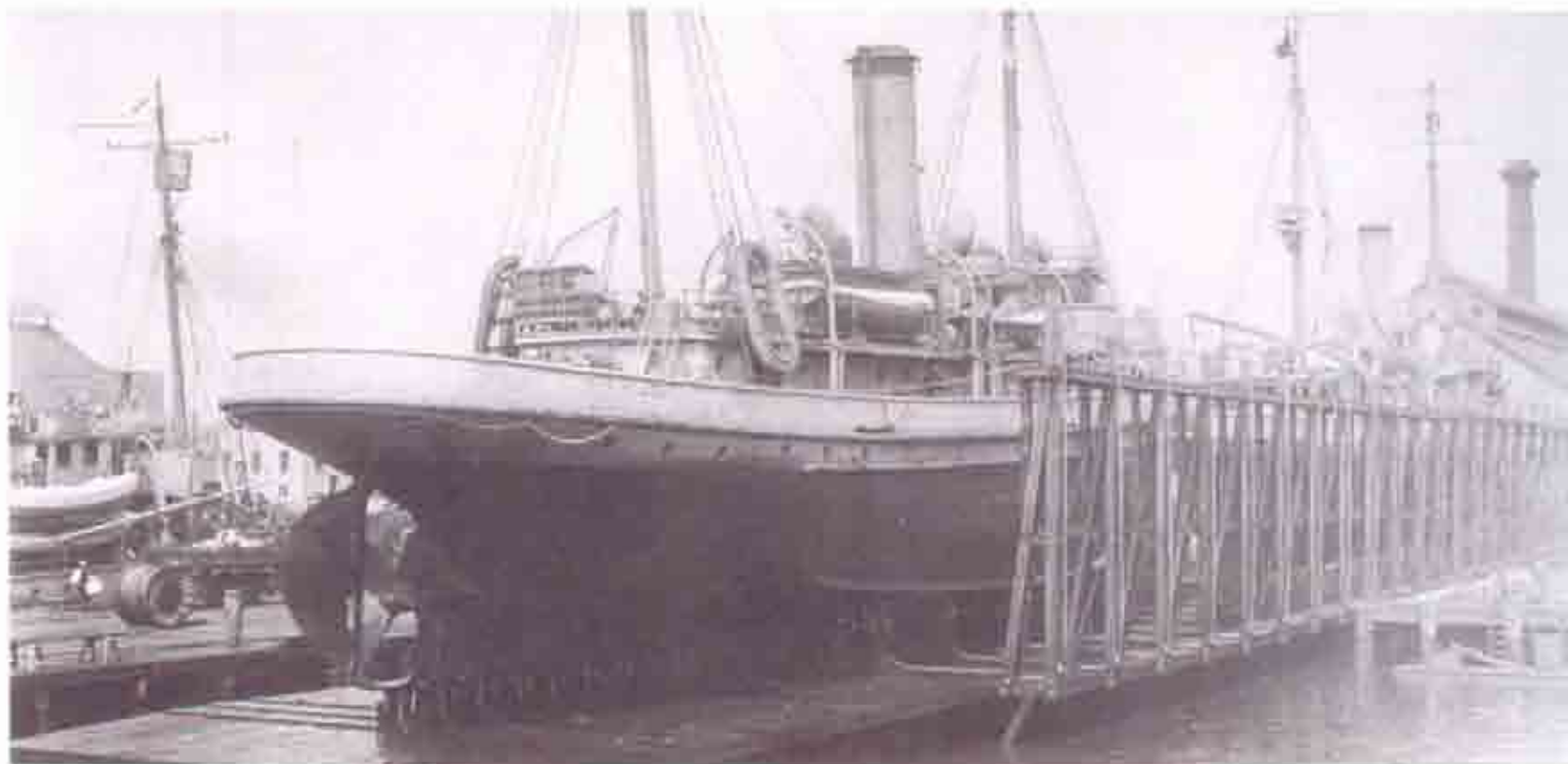
(B45) 1919 photo showing marine railway in operation. Building visible in background, monitor windows open.
