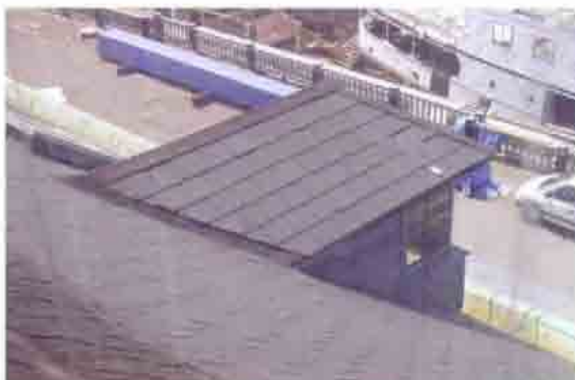
Fig. 16 West elevation dormer. Note temporary repairs made to metal flashing.
