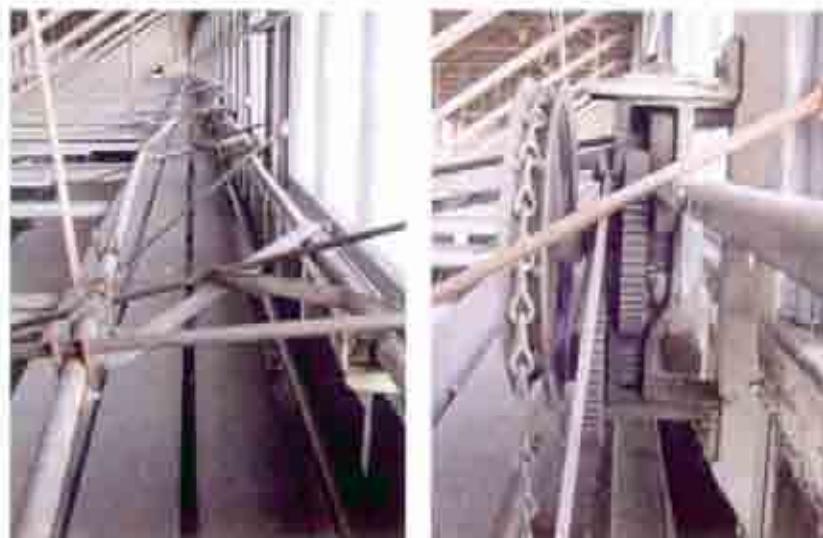
Fig. 18 & 19 Monitor interior. Operating mechanism for window sash.
