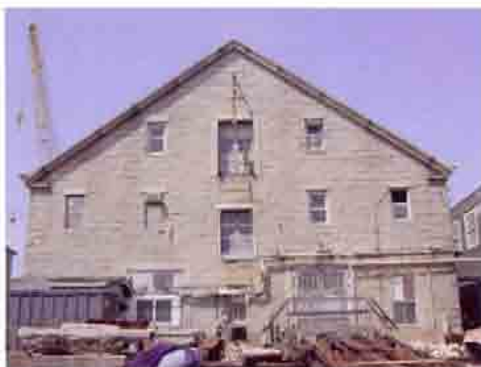
Fig. 4 South Elevation, 1847 Original Building
