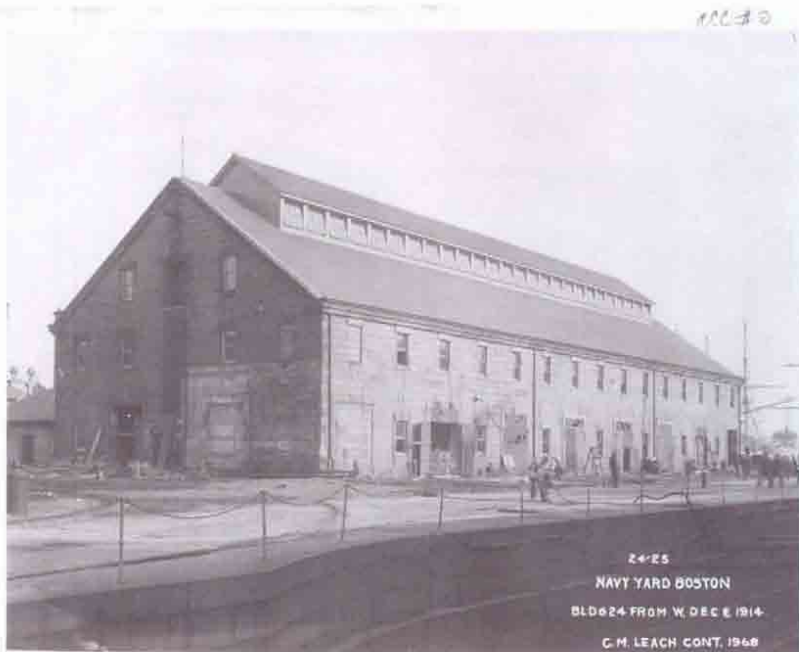
Fig. B-27 Photo "24-25 NAVY YARD BOSTON BLDG 24 FROM W DEC 3 1914 C. M. LEACH CONT. 1968". Exterior, looking southwest. Roof complete, monitor windows installed and partially open, original doors still in place with broken window panes in transoms, new 1/1 windows installed.
