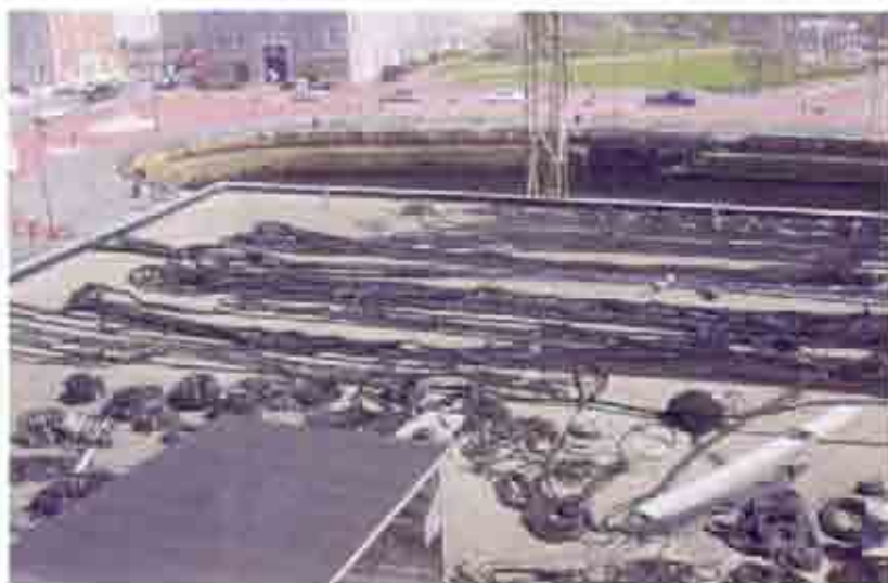
Fig. 21 Flat roof North end of roof
