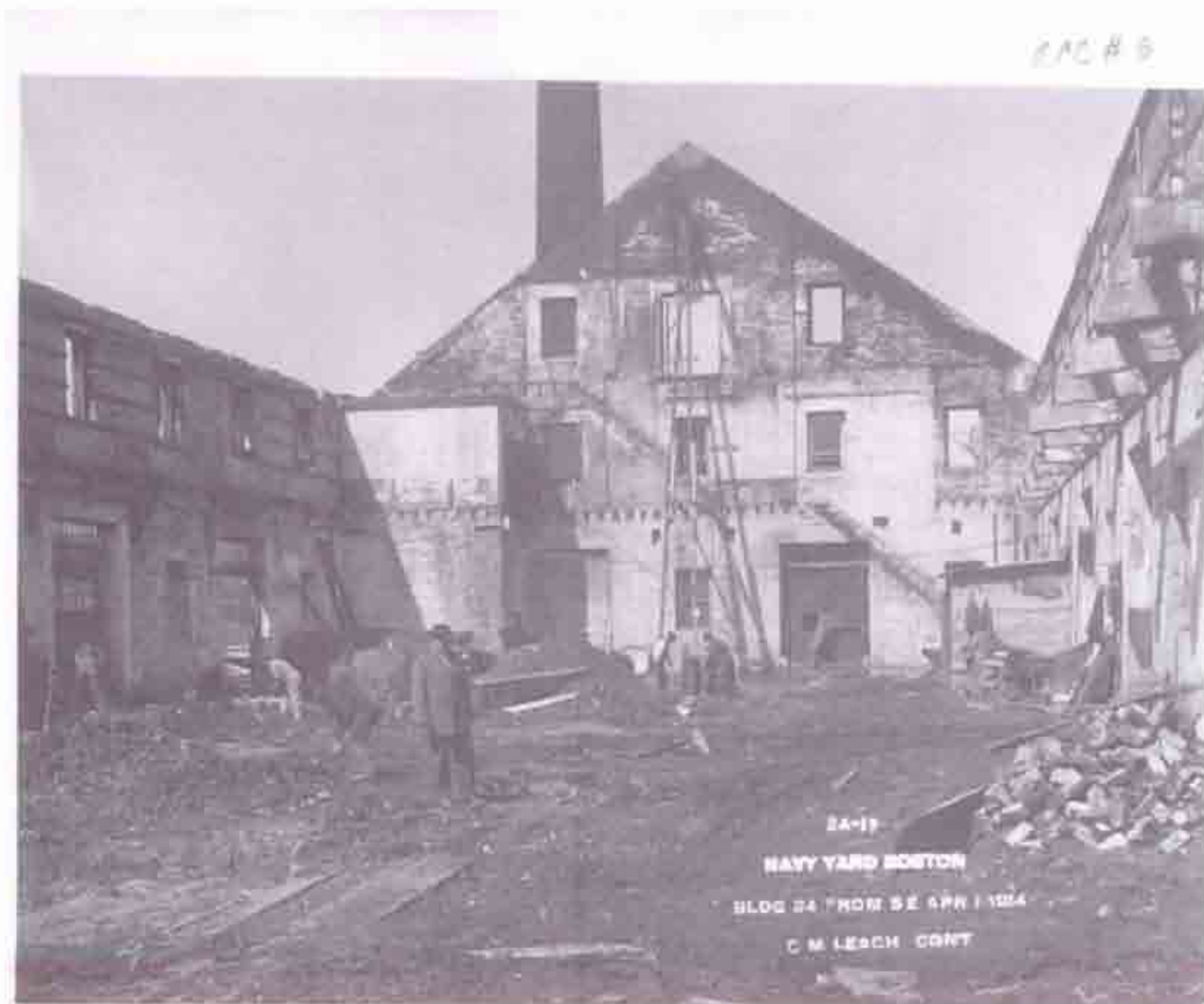
Fig. B-18 Photo "24-17 NAVY YARD BOSTON BLDG 24 FROM SE APR 1 1914 C M LEACH CONT". First floor interior, looking north. All of the roof and floor framing removed. Vault visible in the northwest corner. Ghosting of stairs along north wall.
