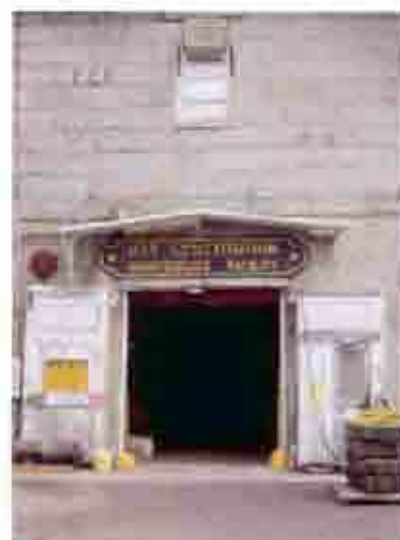
Fig. 25 The main service door, with roll-down door inside.
