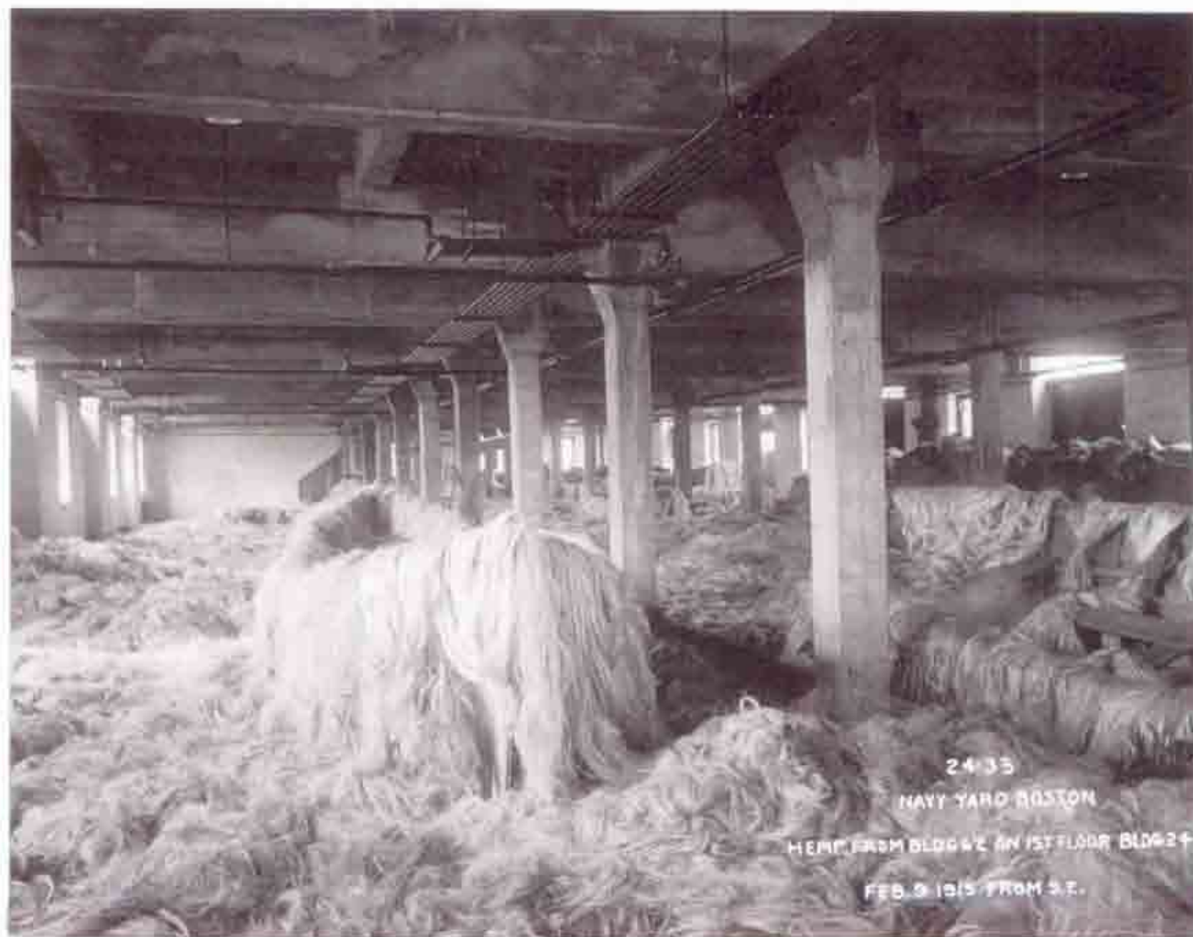
Fig. B-32 "24-33 NAVY YARD BOSTON HEMP FROM BLDG 62 ON 1ST FLOOR BLDG 24 FEB. 9 1915 FROM S.E." First floor interior, looking northwest. Open floor plan.
