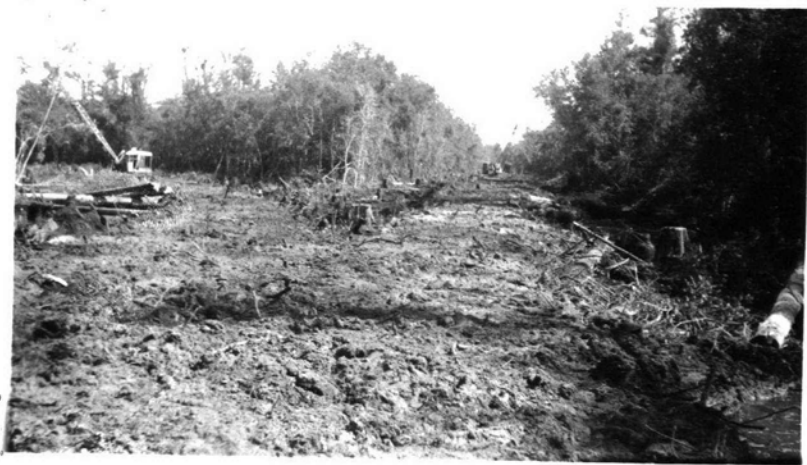
Draglines at work on main road and spur making railroad grades
