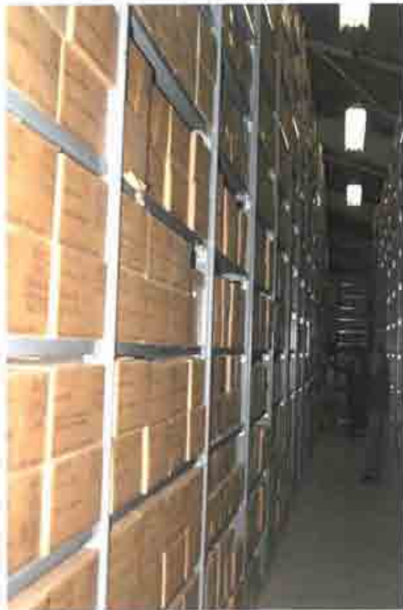
Figure 35: Building 33 has boxes stacked from floor to ceiling on sturdy metal shelving
