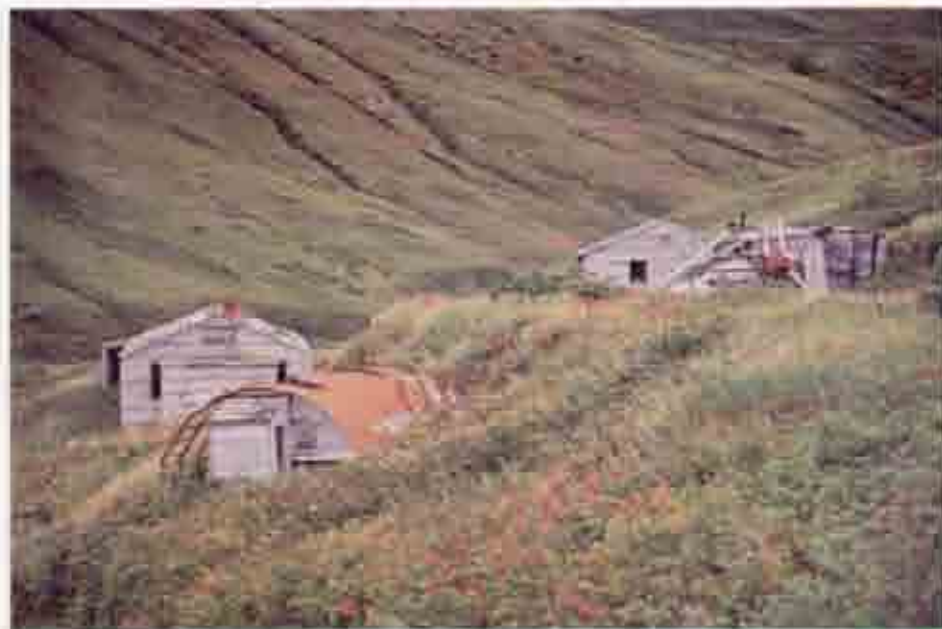
Wood frame mess hall and quonset huts at Eider Point
