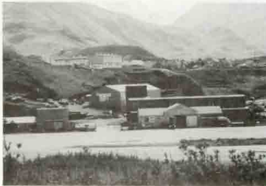
Aerology Building (left) and Torpedo Bombsight Shop with warehouses (right) at the airport. World War II period officers' housing on the hill to the right.
