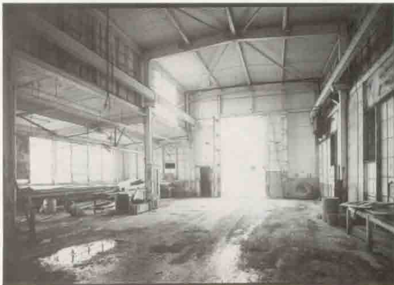
Torpedo Bombsight Shop interior. HABS photo by Jet Lowe, 1985.
