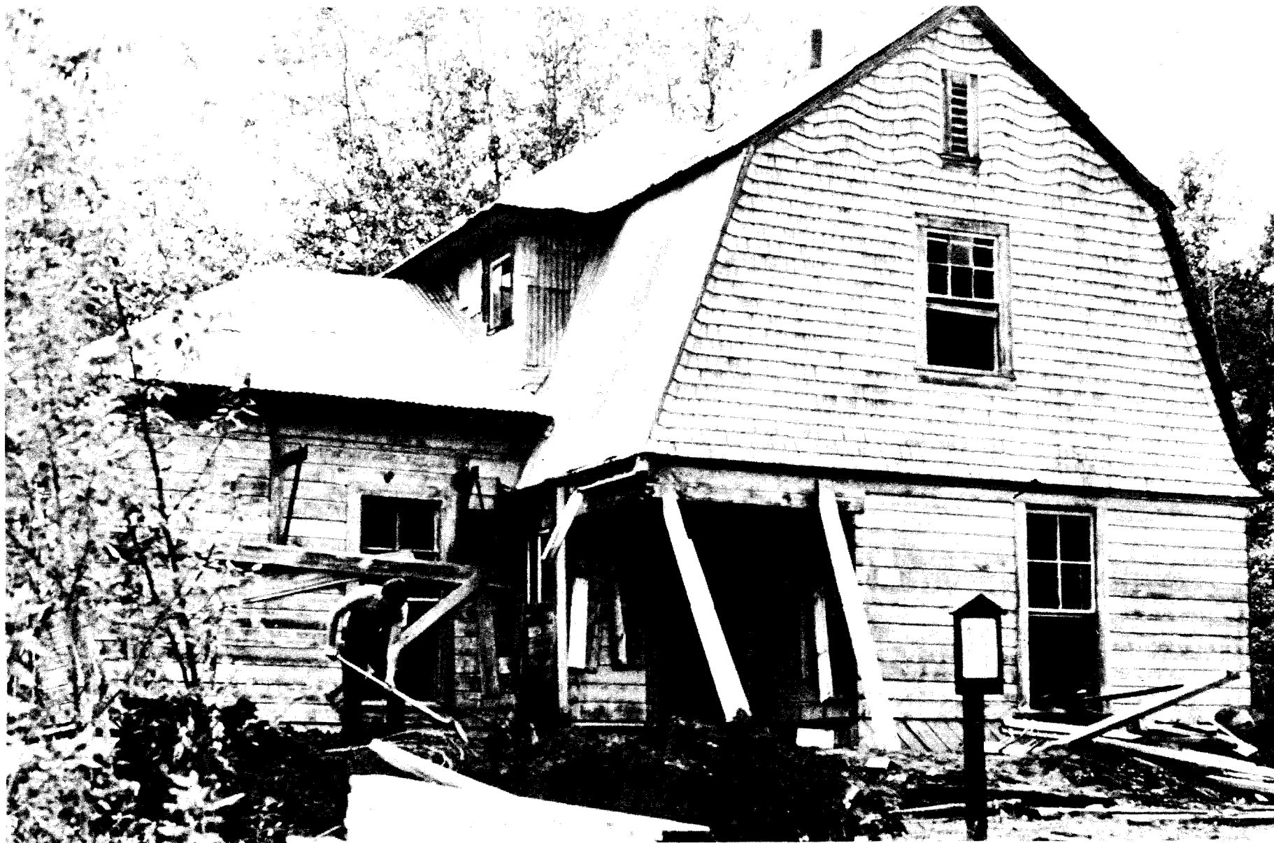
Fort Egbert restoration. (Bureau of Outdoor Recreation)
