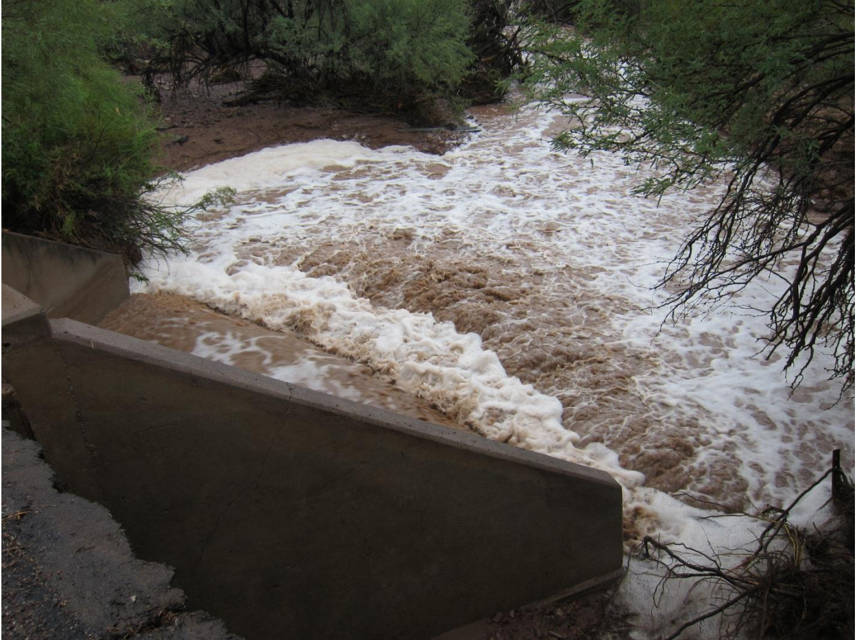
Figure 3. The culvert crossing at mile 66.5 after floodwaters reached Highway 85, August 16, 2012.
