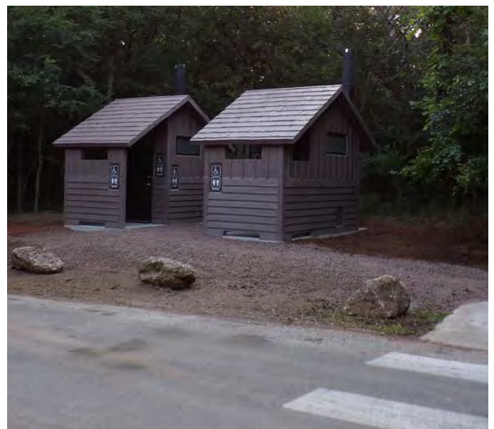
New vault toilets at Panther Falls / NPS Photo
