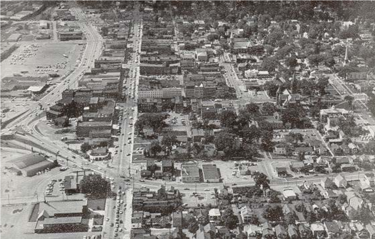
Aerial view of Rome, NY prior to reconstruction of Fort Stanwix, 1969 (FOST Park Archives).
