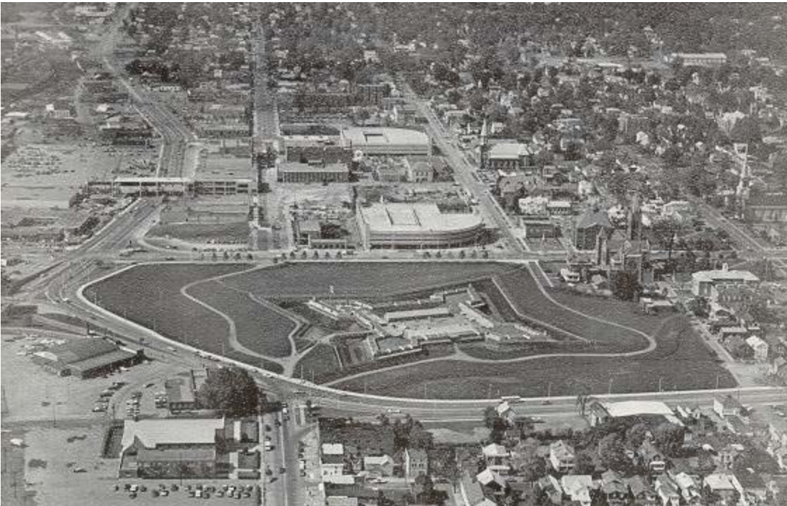
Aerial view of park, showing organization of area surrounding Fort Stanwix, 1976 (Fost Park Library).
