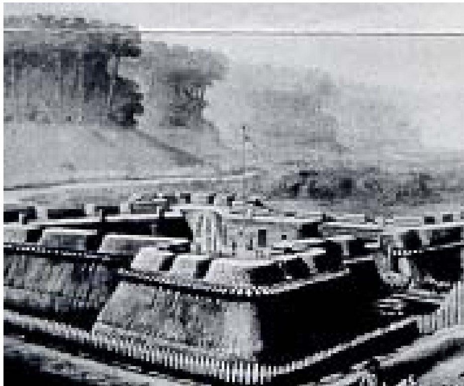
Sketch of Fort Stanwix as it appeared 1777, by Peter Hugonine in 1897 (Rome Historical Society).
