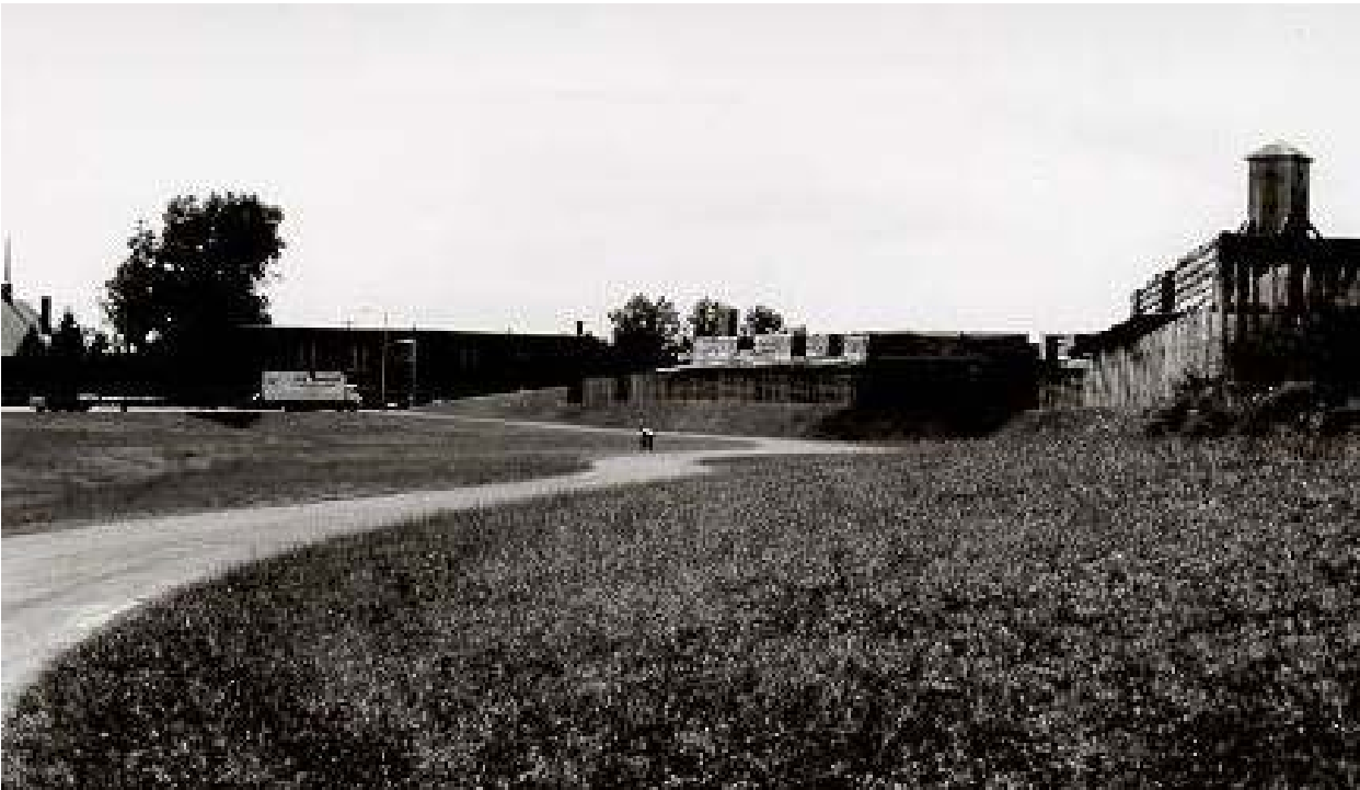
Exterior of fort, 1998 (OCLP FOST CLI Files).
