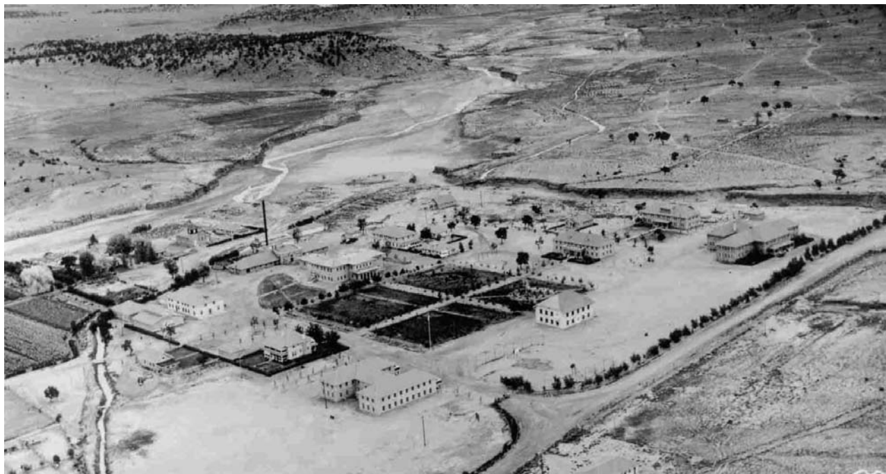
Sage Memorial Hospital School of Nursing Historic District, Ganado, Arizona.
