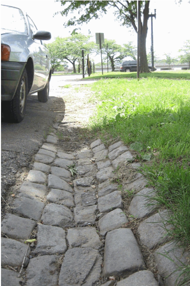
Stone-lined drainage ditch along the Survey Lodge service drive (NCR CLP 2009).
