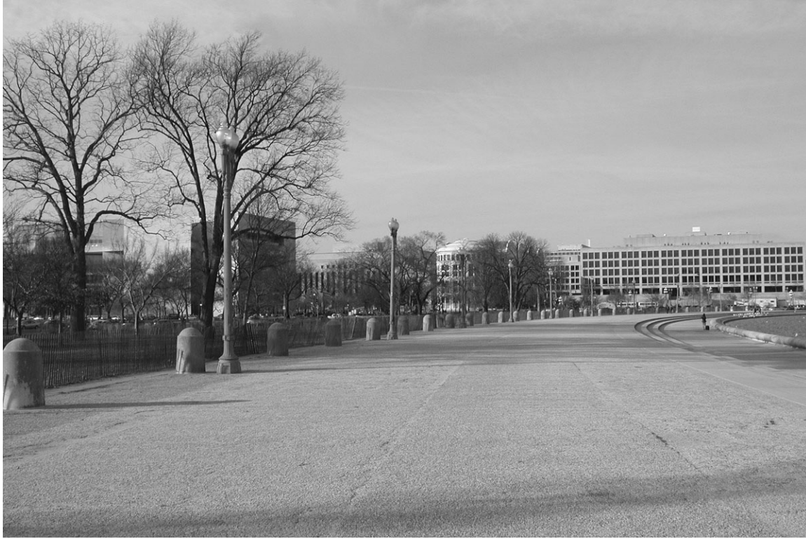
A concrete plaza extends west of the Capitol Reflecting Pool. View looking north. (CLP file "plaza west of pool" Feb. 10 2006)
