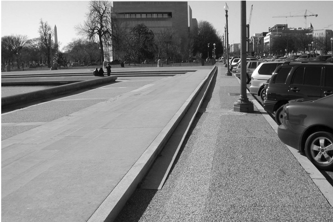
Two odd steps are located next to the sidewalk northwest of the pool. View looking west. (CLP file "granite step along N edge pool plaza, slope" Feb. 24 2006)
