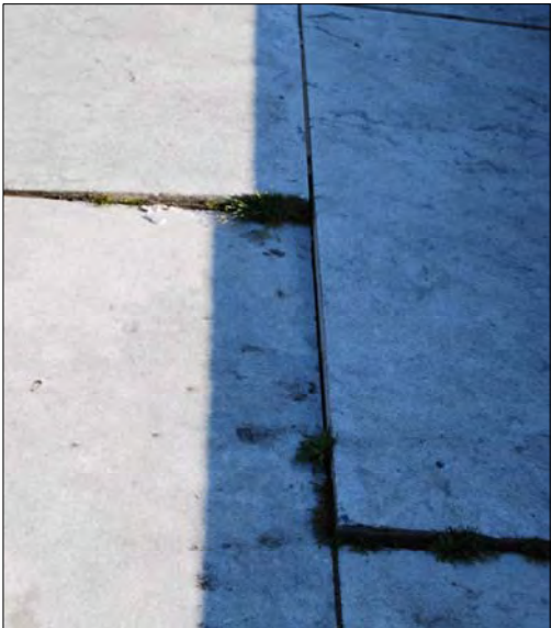
Paving is uneven and shows damage from skateboarding.
