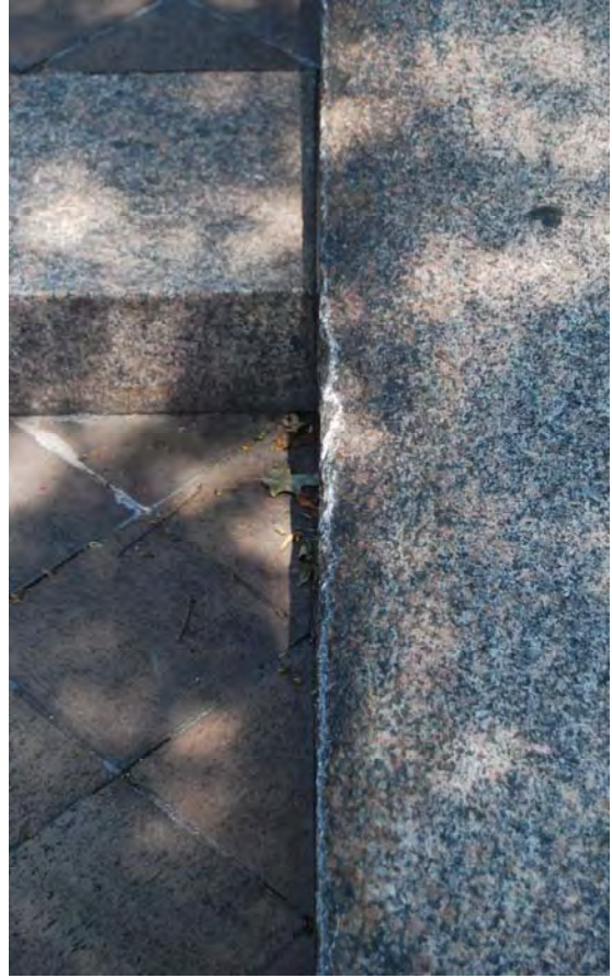
Some lampposts are out of alignment. Low places collect water, making tables unusable. Skateboarding has damaged granite curbing (above).
