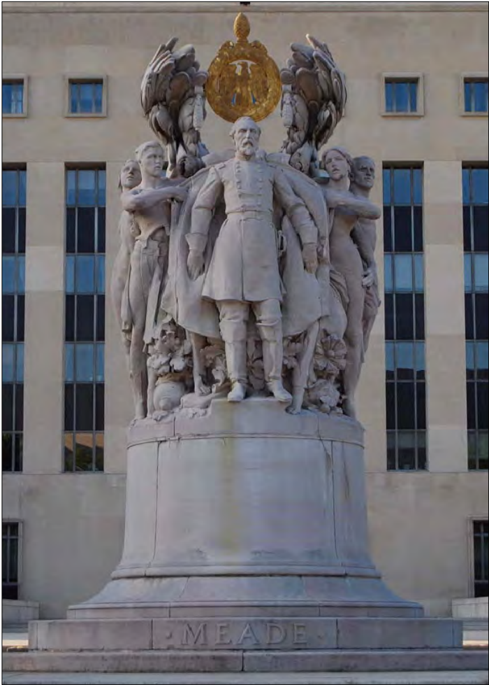
The pedestal shows signs of staining and deterioration. Skateboarding damage occurs on stairs, walls, and the base of the statue.
