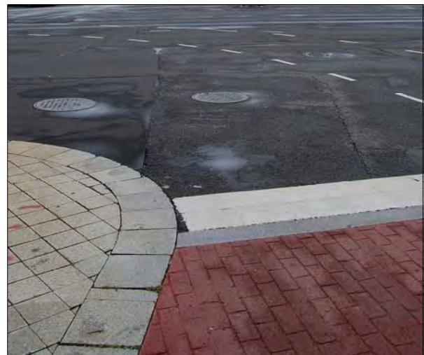
The crosswalk at 3rd and Pennsylvania Avenue is paved with brick to indicate the pedestrian right-of-way.
