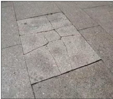
A granite paver in Freedom Plaza (above) is cracked. Paving at Indiana Plaza (right) combines brick and granite in a stacked bond pattern.
