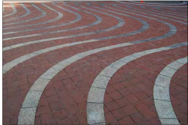
Paving in Franklin Plaza in front of the Old Post Office combines red brick and granite pavers in a curvilinear design.
