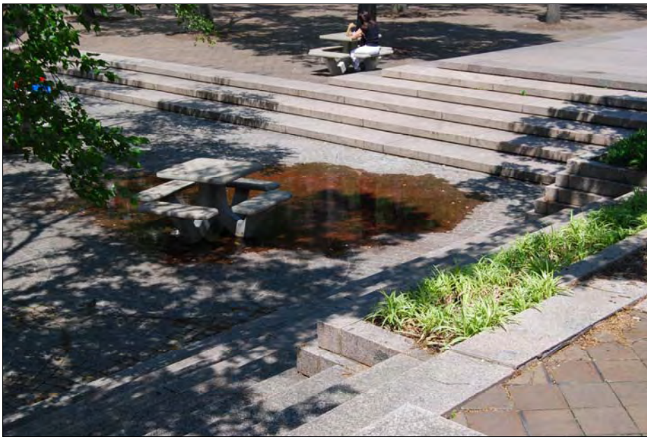
Some lampposts are out of alignment. Low places collect water, making tables unusable. Skateboarding has damaged granite curbing (above).
