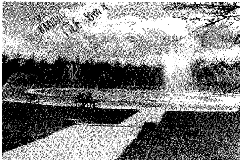
Figure 47 - Concrete walks radiating from the Rainbow Pool, April 1933. MRC 2-126.
