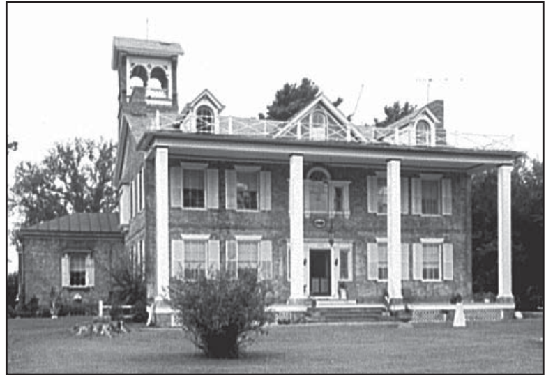
Figure 2.1. The Campbell colonial revival style porch Source: Library of Congress
