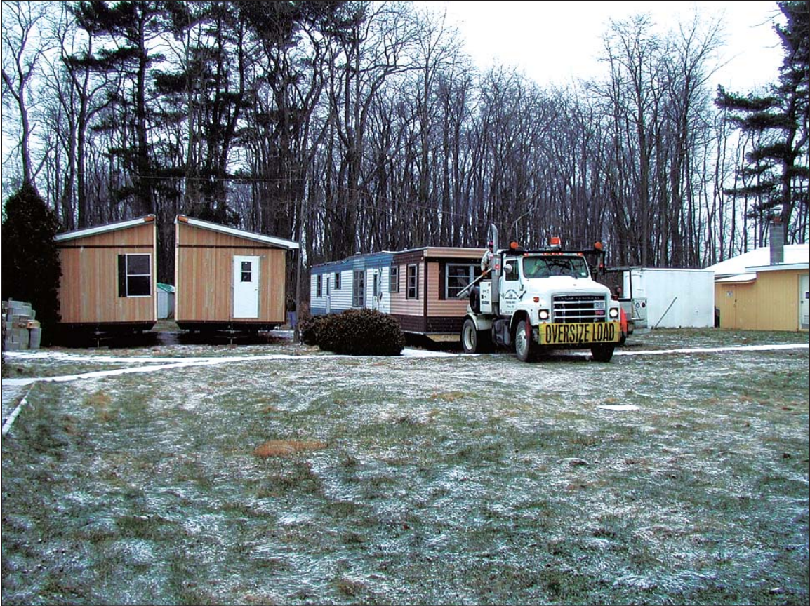
Figure 6.1. Removing old trailers behind maintenance garage, 2001 Source: Photograph MAVA Collection
