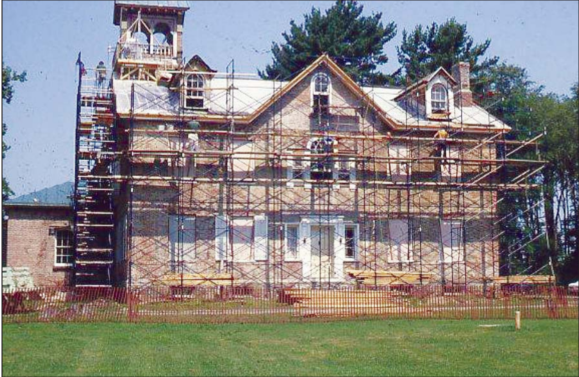
Figure 3.3. Exterior restoration in progress Source: Photograph MAVA Collection
