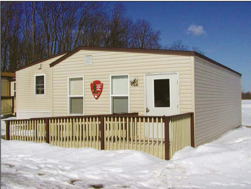
Figure 6.4. Makeshift Visitor Center attached to trailers Source: Photograph MAVA Collection
