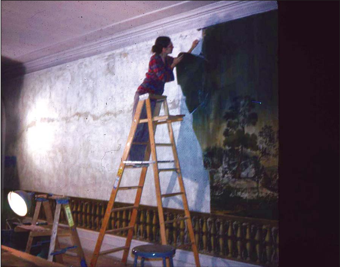
Figure 2.7. Patricia Dacus Hamm removes historic wallpaper Source: Photograph MAVA Collection
