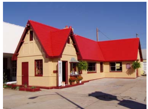
Top: Rehabilitation of the Vickery Phillips 66 Station was completed this year in Tulsa, Oklahoma with program grant assistance. The property is now in use as a rental car facility.
