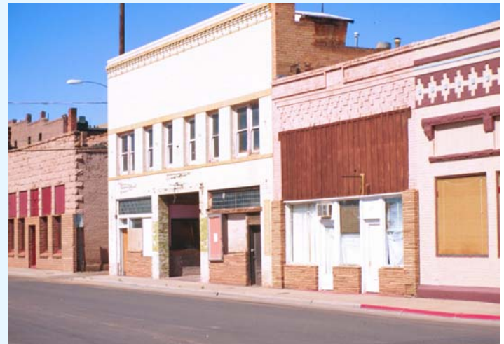
Rialto Theatre in 2001, before rehabilitation.
