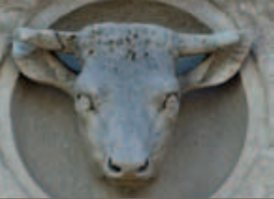
Detail, Old Stone Gate, Chicago Union Stockyards Illinois
