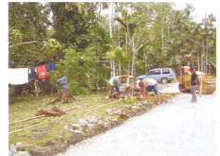
BAC Staff surveying a site
