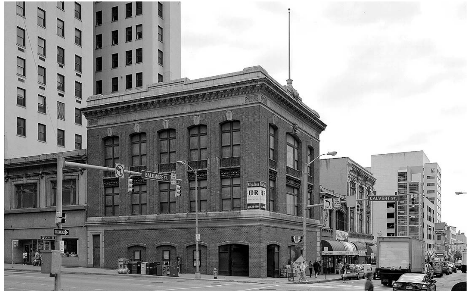
Pennsylvania Railroad Company District Office from southwest. James W. Rosenthal, photographer, Summer 2001.
