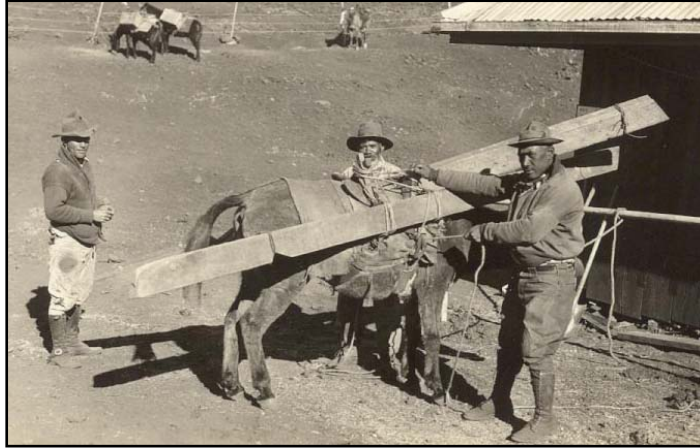
Figure 18. Labor crews preparing loads at Red Hill Rest House for construction of the Summit Rest House (ca. 1934) (photo courtesy of the National Park Service, Hawaii Volcanoes National Park).
