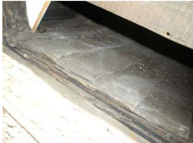
Original roof shingles, circa 1802
