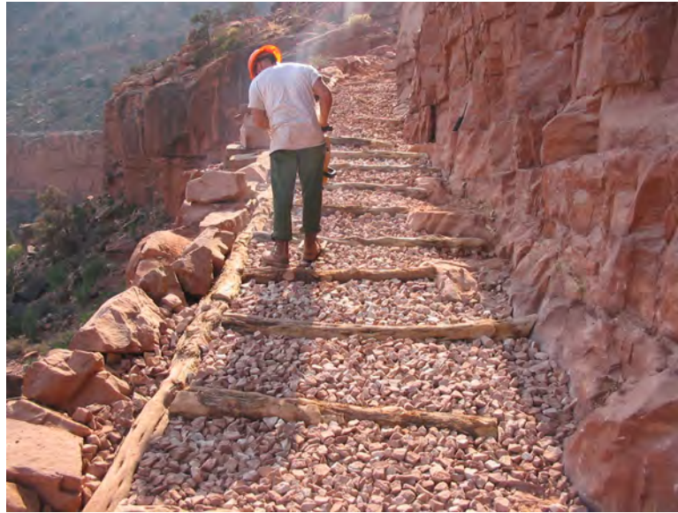
Figure 40: ‘working the canyon’s rocks - connecting with American history’
