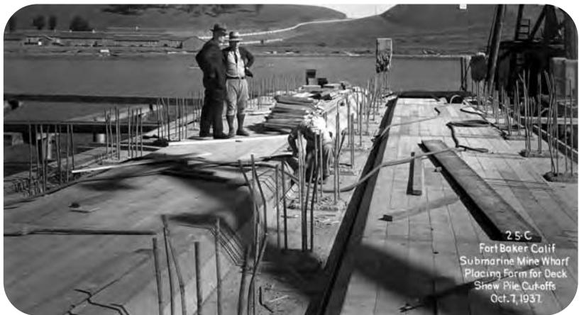
The army undertook a major construction project at Horseshoe Cove, building a submarine mine wharf to accommodate the large mineplanter ships. The new wharf, constructed with concrete and pilings, abutted the existing 1903 quartermaster supply wharf. Note Fort Bakers' open landscape in the background. (photo 1937)
