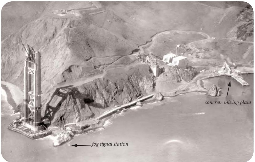
The Golden Gate Bridge was constructed between 1933 and 1937; the pier for the north tower abutted at the base of Lime Point. The Horseshoe Cove area was used as a staging area for construction activity. Note the fog signal station at the lower left and the bridge-related concrete mixing plant just north of the Needles. (photo circa 1934; courtesy of the Golden Gate Bridge District)
