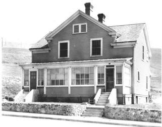
Historic view of FB523. (NPS photo, 1938 Quartermaster Report)
