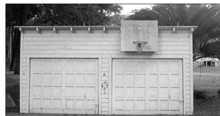
Basketball Hoop, 2001 Location: FB538 Extant, non-historic, incompatible
