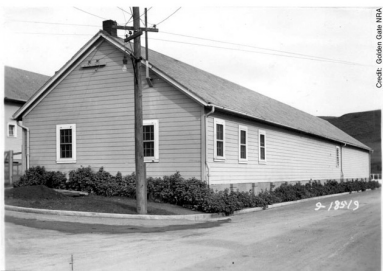
Building FB561 (NPS photo, 1938 Quartermaster report)
