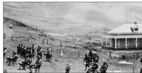
Fence, Circa 1915 Location: FB533, looking east Removed
