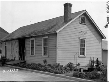
Building FB644 (NPS photo, 1938 Quartermaster report)
