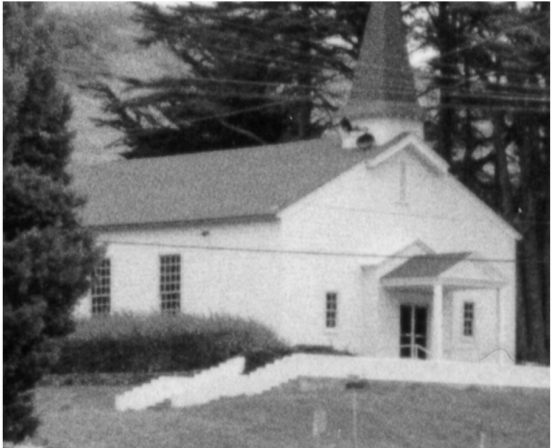
Building FB519, view looking west. Removal of historic vegetation has altered the landscape character. (NPS, 2001)
