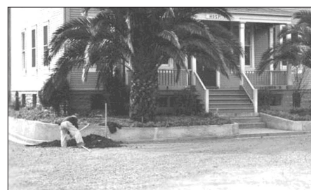
Concrete Retaining Wall, Circa 1938 Location: FB533 Extant
