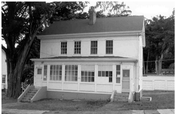
Contemporary view of FB530.(NPS, 2001)
