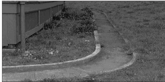
Walkway, 2001 Location: FB607 Extant
