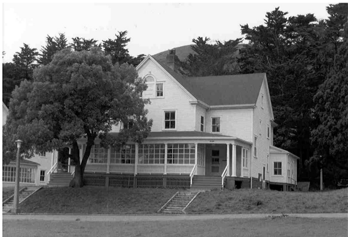
Building FB629, view looking west. Removal of historic vegetation has altered the landscape character. (NPS, 2001)
