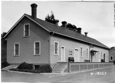
Building FB559 (NPS photo, 1938 Quartermaster report)
