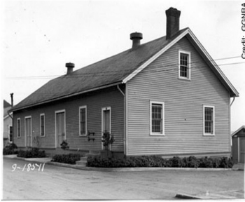
Building FB666 (NPS photo, 1938 Quartermaster report)
