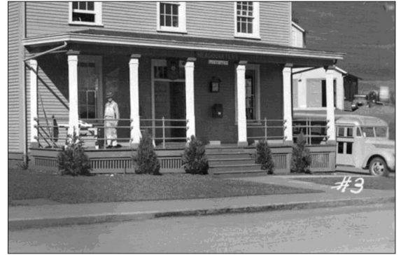
Sidewalk Curb, Circa 1938 Location: FB603 Extant
