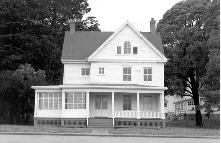
Building FB604, looking north. The foundation plants have all been removed.
