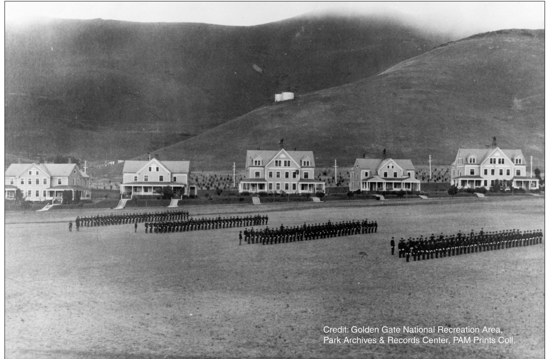
SH12 Concrete walkways and stairs led at regular intervals from the Murray Circle sidewalk to each building, looking west. Circa 1915 (GGNRA Park Archives and Record Center, 1766.0021).
