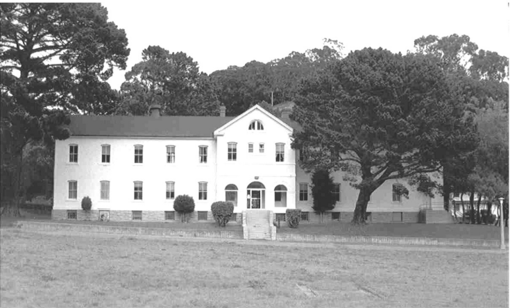
Building FB636, looking east. (NPS, 2001)
