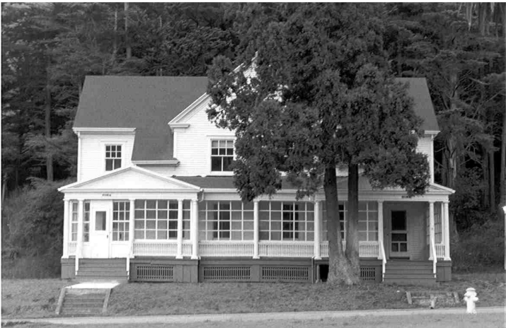
Building FB606, view looking west. Removal of historic vegetation has altered the landscape character. (NPS, 2001)
