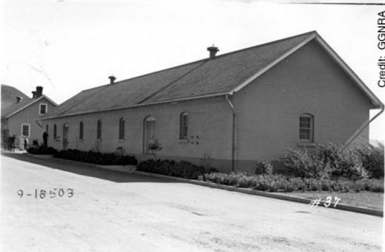
Building FB637 (NPS photo, 1938 Quartermaster report)
