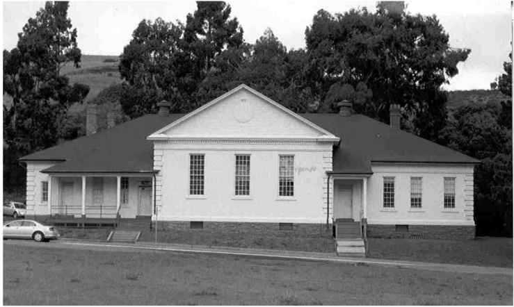
Building FB623, looking east. All plant material has been removed. (NPS, 2001)
