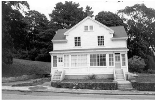
Contemporary view of FB523. (NPS, 2001)
