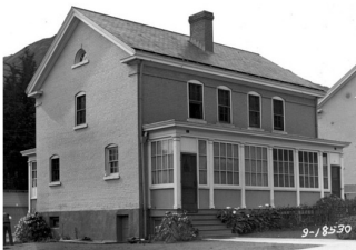
Historic view of FB530.(NPS photo, 1938 Quartermaster Report)
