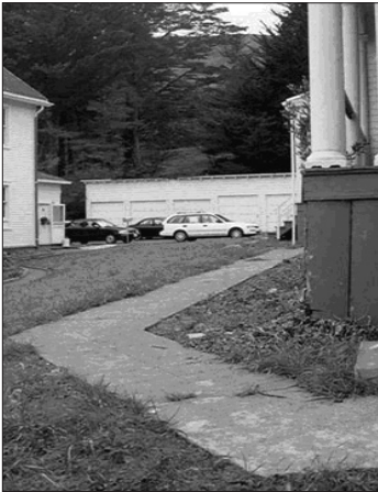
Walkway, 2001 Location: FB631 Extant
