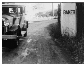
Fence, Circa 1925 Location: East Road Entrance Removed
