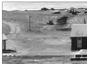
Fence, Circa 1937 Location: Waterfront, looking south Removed
