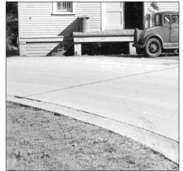
Road Gutter, Circa 1925 Location: FB631 Extant
