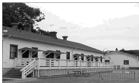
Railing, 2001 Location: Service area Extant
