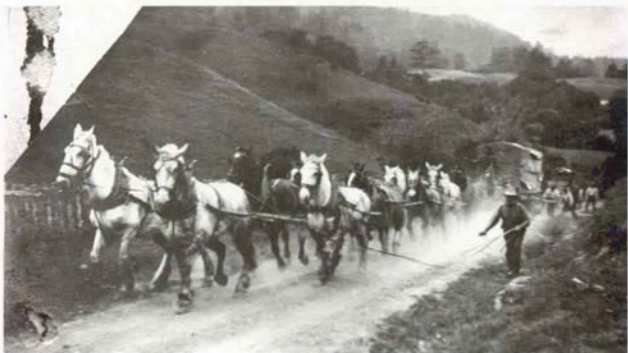
A load of equipment for the Marconi Wireless station at Bolinas is hauled from the train depot at Point Reyes Station up Muscio Hill in 1914. Courtesy of Helen Harris.
