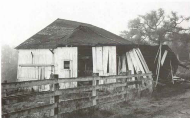
The horse barn shortly before it was demolished, February 1994. NPS photograph by Dewey Livingston.
