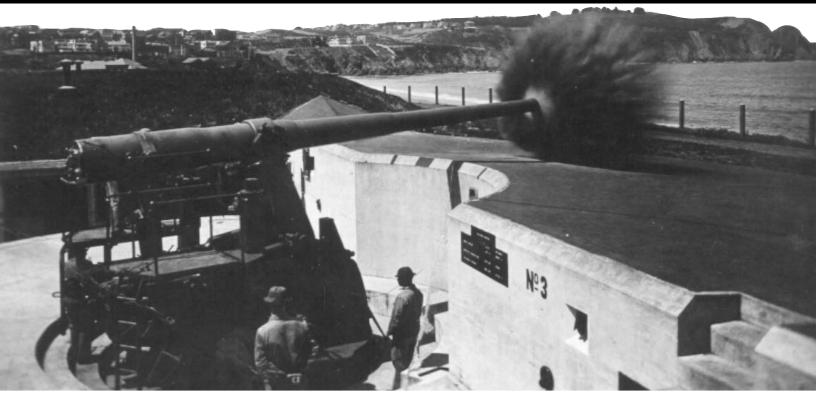
Practice firing of an original 6-inch gun mounted on a disappearing carriage, around 1910.
