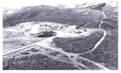
Tracking Radar. Now looking west to the right of it, down the steps and behind the Volkswagon, is the radar control computer van. To its right is the Low Power building, renamed from "corridor building" as previously referenced. It too had essential air-conditioning, and it too still exists. To the northwest is the generator building and then the fuel dump. We are now looking north. All three of the Coast Guard's transmitter buildings are visible as is its
