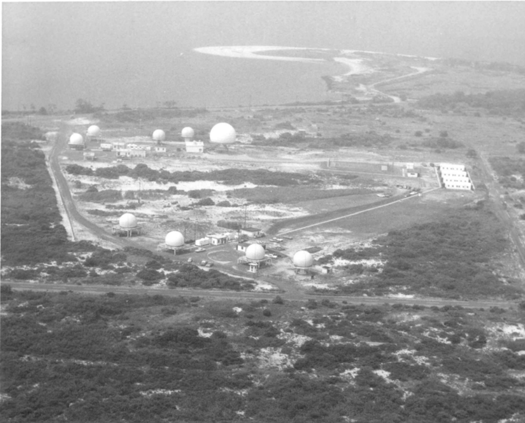
The Fort Hancock IFC where Mr. Busch worked. C-2 is in the foreground, barracks are to the right and C-1 is in the background.
