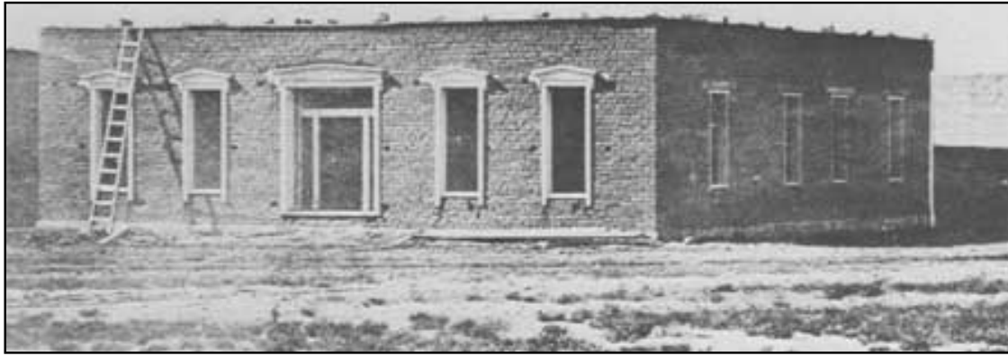
Officer's quarters under construction at third Fort Union, U.S. Signal Corps Photo No. 88013, courtesy National Archives.
