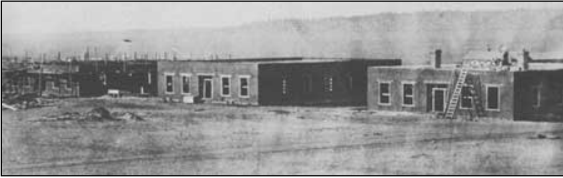
Officers' row under construction, U.S. Signal Corps Photo No. 87996, courtesy National Archives.
