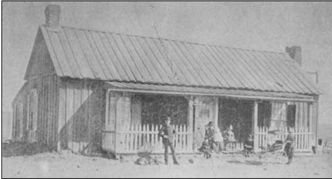
Thomas and Robina Keeshan with their children (five of their six children survived) at the post commissary sergeant's quarters at Fort Union, about 1887. These board and batten frame quarters were located north of the depot storehouses. Keeshan Collection, Fort Union National Monument.
