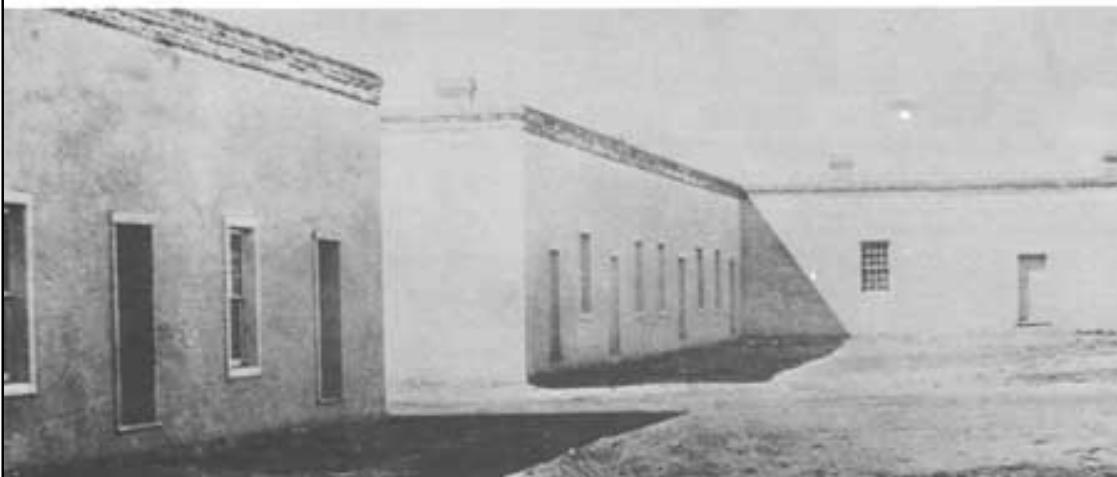
Four views of company quarters under construction at the third Fort Union, from top to bottom, U. S. Signal Corps Photos Nos. 88014, 88015, 88018, 88017, courtesy National Archives.
