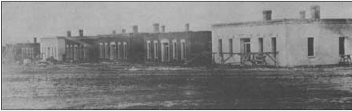
Officers' row under construction; note that two of the buildings have been plastered on exterior. U.S. Signal Corps Photo No. 88012, courtesy National Archives.
