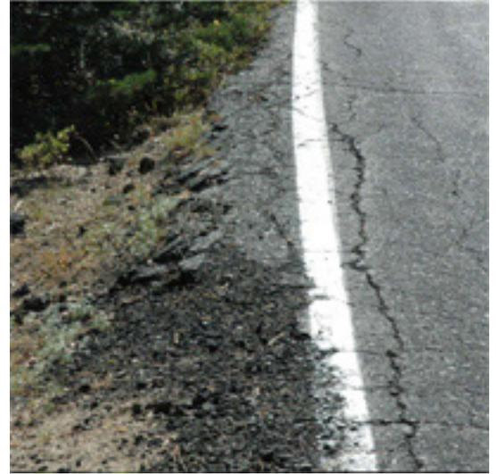
**Cracking and deteriorating asphalt on the Tioga Road can undermine the road's structure and cause potential safety hazards.**
