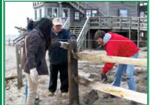
Park volunteers help rebuild split rail fence damaged by Hurricane Sandy.
