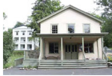
The Peters Valley Craft Store and Greek Revival House today. (NPS Photo by Ken Sandri)
