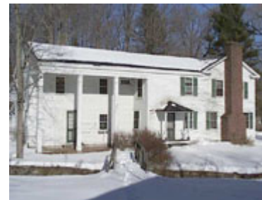
Valley Brook Farmhouse. (NPS Photos by Ken Sandri)
