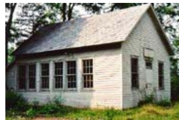
The south exterior of Calno School in 2004.
