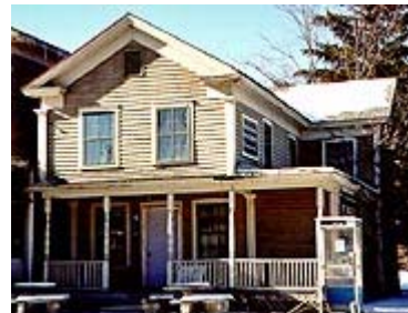
(Above) The tinsmith's shop (now the north wing of the Turn and Cook General Store building) in Bushkill PA shows Greek Revival influence on vernacular architecture.
