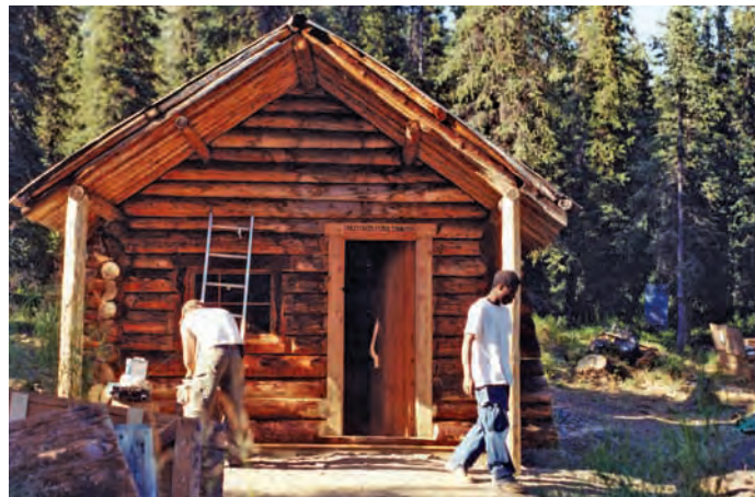
Projects to restore historic cabins, such as the Riley Creek Cabin, are required to comply with the National Historic Preservation Act.
