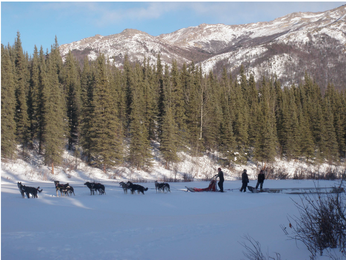
Sled dogs hauling materials for Riley Creek footbridge
