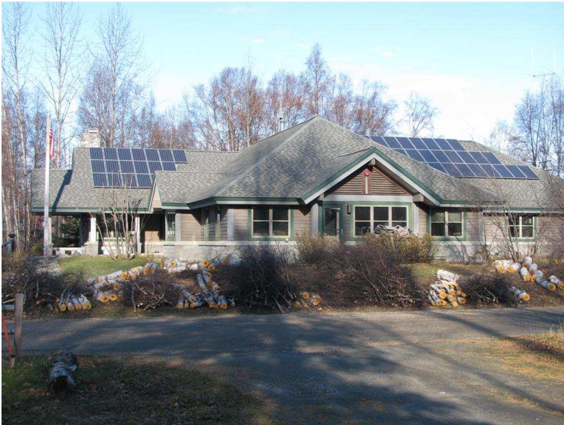
Talkeetna Ranger Station with new solar panels
