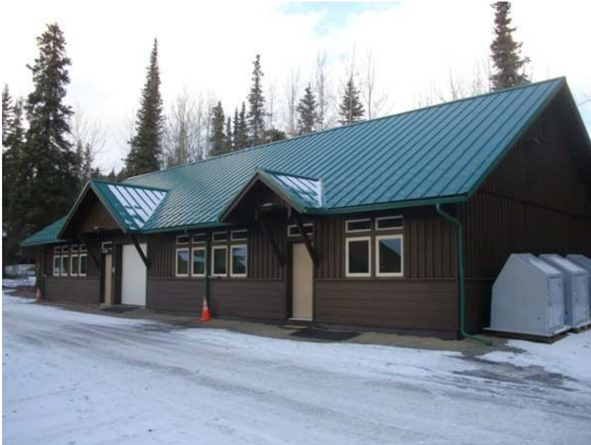
New IT building
