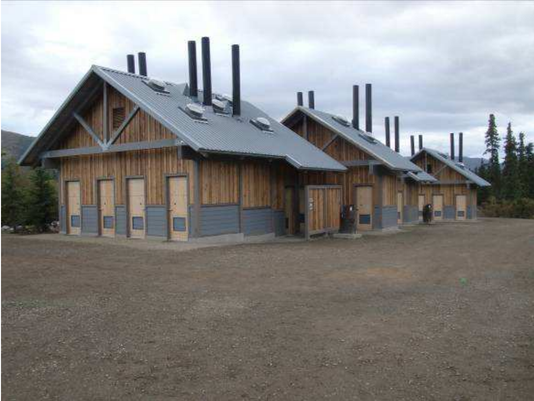
New vault toilets at the Teklanika River Rest Area
