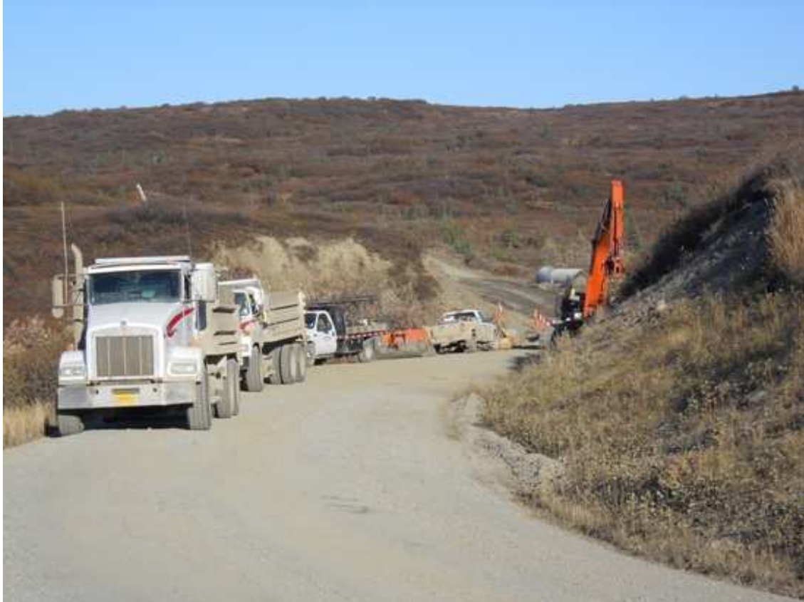
Work at Mile 82
