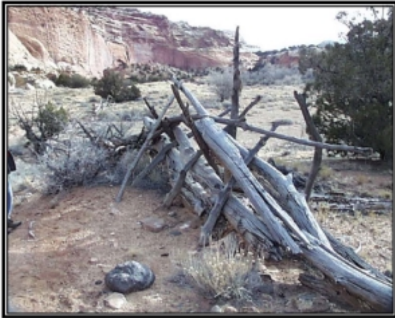
Detail of Fence Construction on Sleeping Rainbow Ranch, 2000 (NPS Photo).
