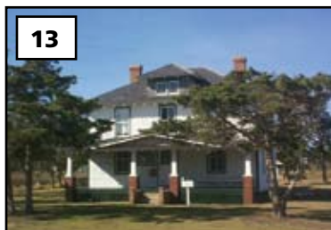
13 Theodore and Annie Salter House: serves as a visitor center; inside are exhibits and public restrooms.
