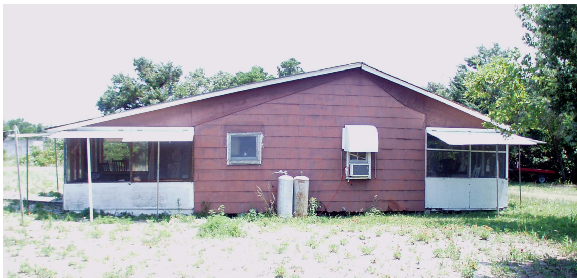
Figure 5 View of southwest side of house, showing line of original roof prior to installation of present roof after 1976. (NPS-SERO-CRS, 2002)
