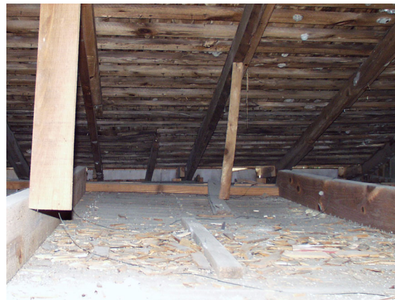
Figure 4 View to southeast in attic of original house. (NPS-SERO-CRS, 2002)
