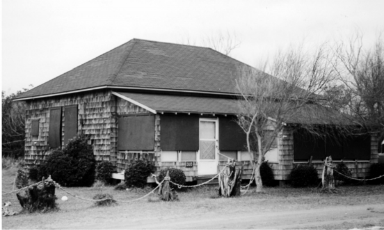
5 Life Saving Station Boathouse
