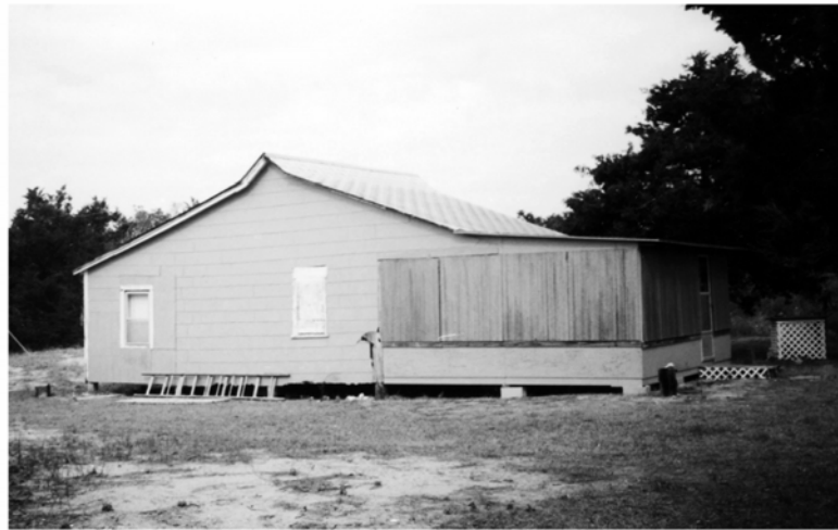
6 O'Boyle-Bryant House (Bryant)
