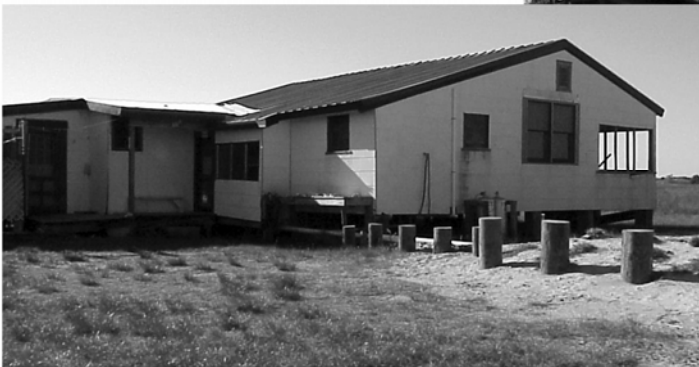
11 Jetty Workers House #2
