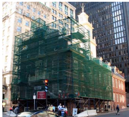
Old State House during restoration
