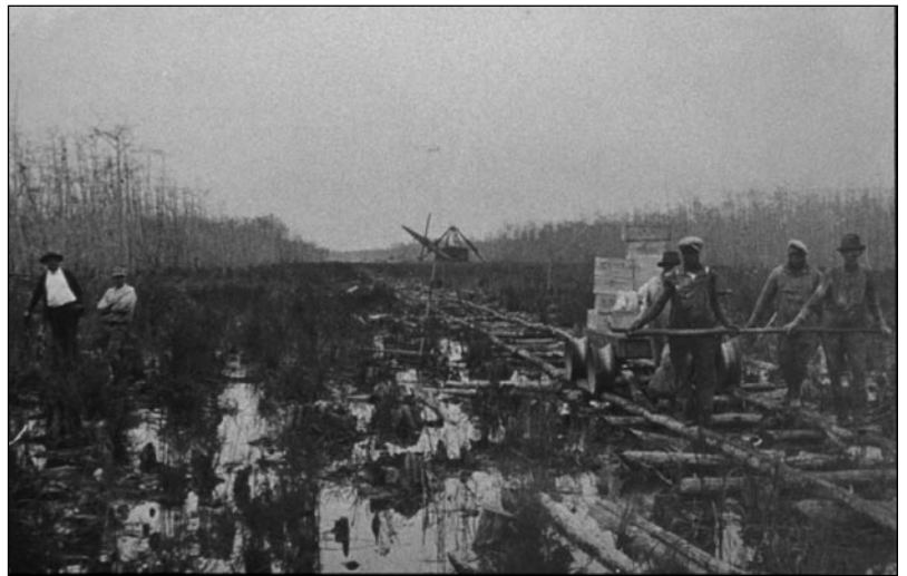
Laying a railroad track into the heart of the swamp.
