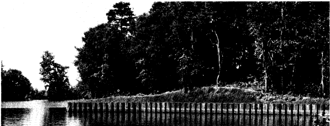
Figure 7. Sheet steel pilings will protect the unexcavated ceremonial mounds at Rood Creek for possible future investigation. Photo credit: Walter Smalling, Jr.
